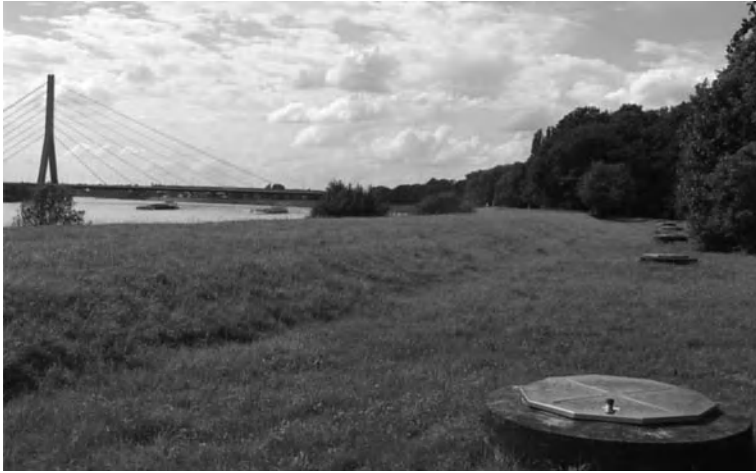
Figure 18.2 Photograph of vertical wells along the River Rhine at Duesseldorf-Flehe.
