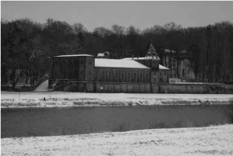
Figure 18.4 Photograph of Dresden-Saloppe Waterworks in 2009.
