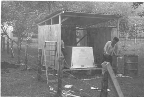
Installation of Lamont seismograph station at Niumate in Tonga, 1964
