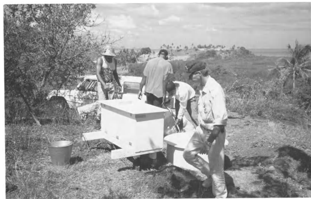
Installation of seismograph station in Fiji, 1965
