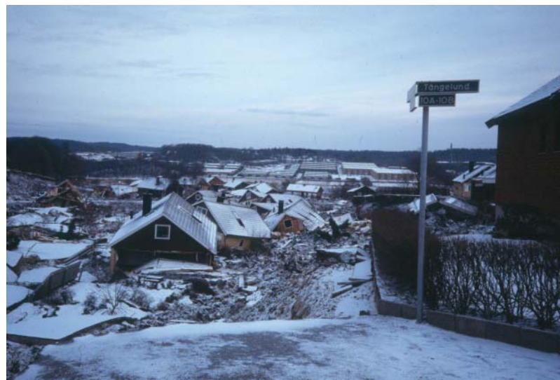
Figure 2.3 Landslide in quick clay near Tuve, Sweden (J. M. Duncan photo and drawing).
