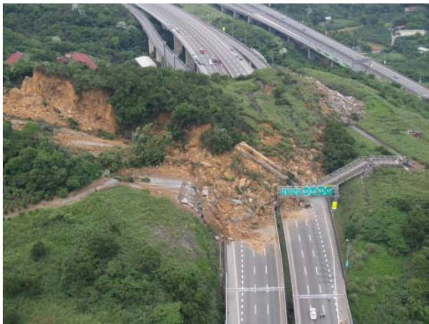
Figure 2.4 Landslide on No. 3 Freeway in Taiwan (Lee et al.; 2012; photograph courtesy Taiwan Geotechnical Society and Ministry of Transportation, Taiwan).
