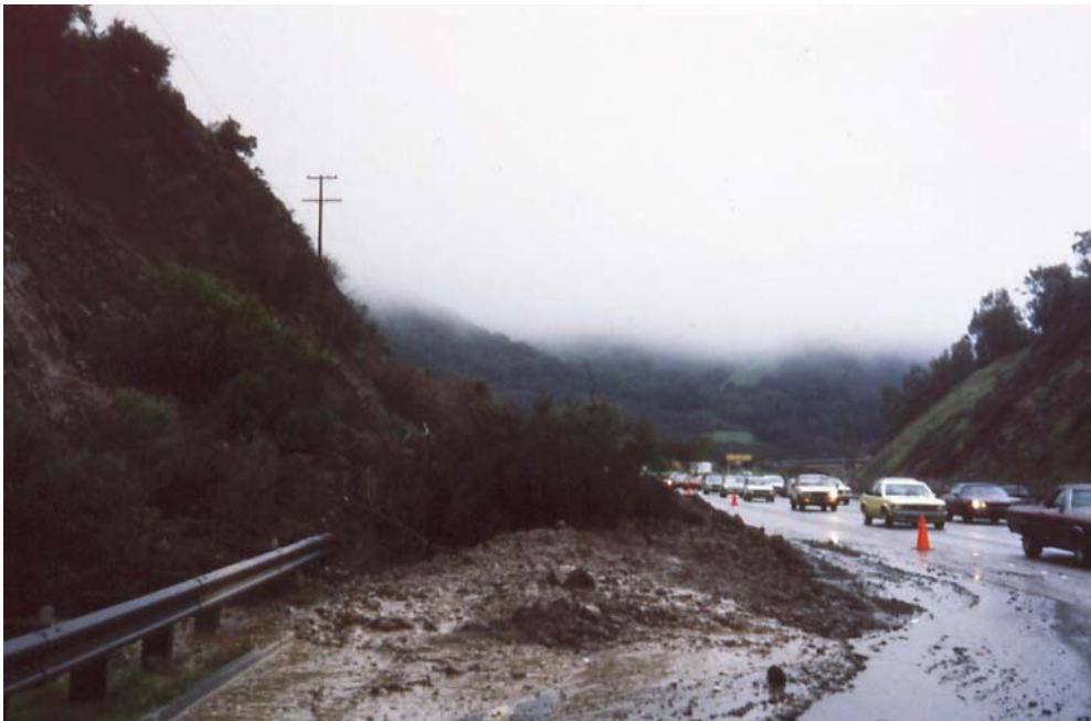
Figure 2.2 Flow slide on Highway 24 near Orinda, California (J. M. Duncan photo).
