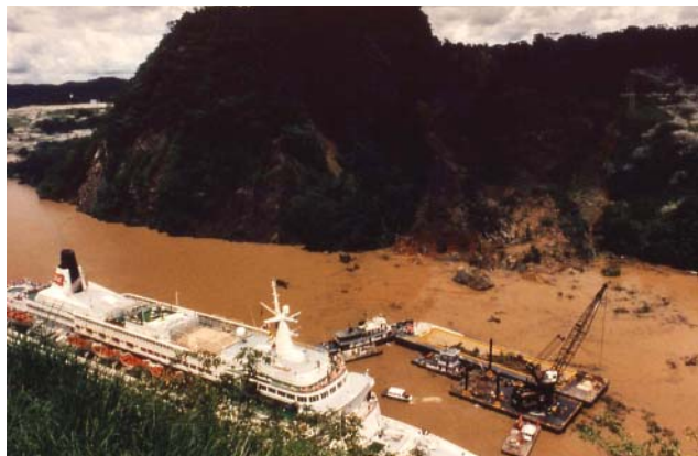
Figure 2.13 The 1986 Cucaracha landslide at the Panama Canal (photograph courtesy of the Panama Canal Authority).
