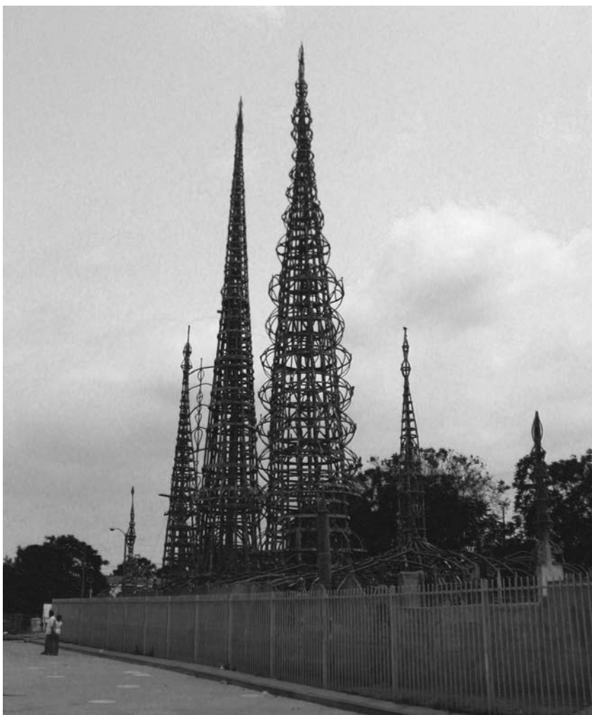
FIGURE 64. Watts Towers. Immigrant Sabato (Simon) Rodia single-handedly constructed two ninety-nine-foot towers and a dozen other buildings between 1921 and 1954 in the community of Watts in Los Angeles County. The towers are twisted steel covered with concrete that is decorated with glass, tiles, and found objects. The site is now protected as a State Historic Park and National Historic Landmark. (Wikimedia Commons.)
