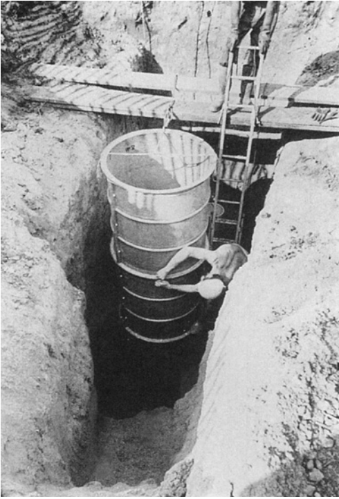
Fig. 10. Installation of prototype 'minipuit' (from IGS Annual Report 1973, Plate 11. Photo British Materials Engineering Limited. IPR/36-16C British Geological Survey. ©NERC. All rights reserved).
