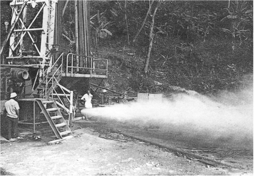
Fig. 11. Discharge of wet steam from Borehole 4 during the St Lucia geothermal project (from IGS Annual Report 1975, Front cover. Photo D.K. Buckley. IPR/36-16C British Geological Survey. ©NERC. All rights reserved).
