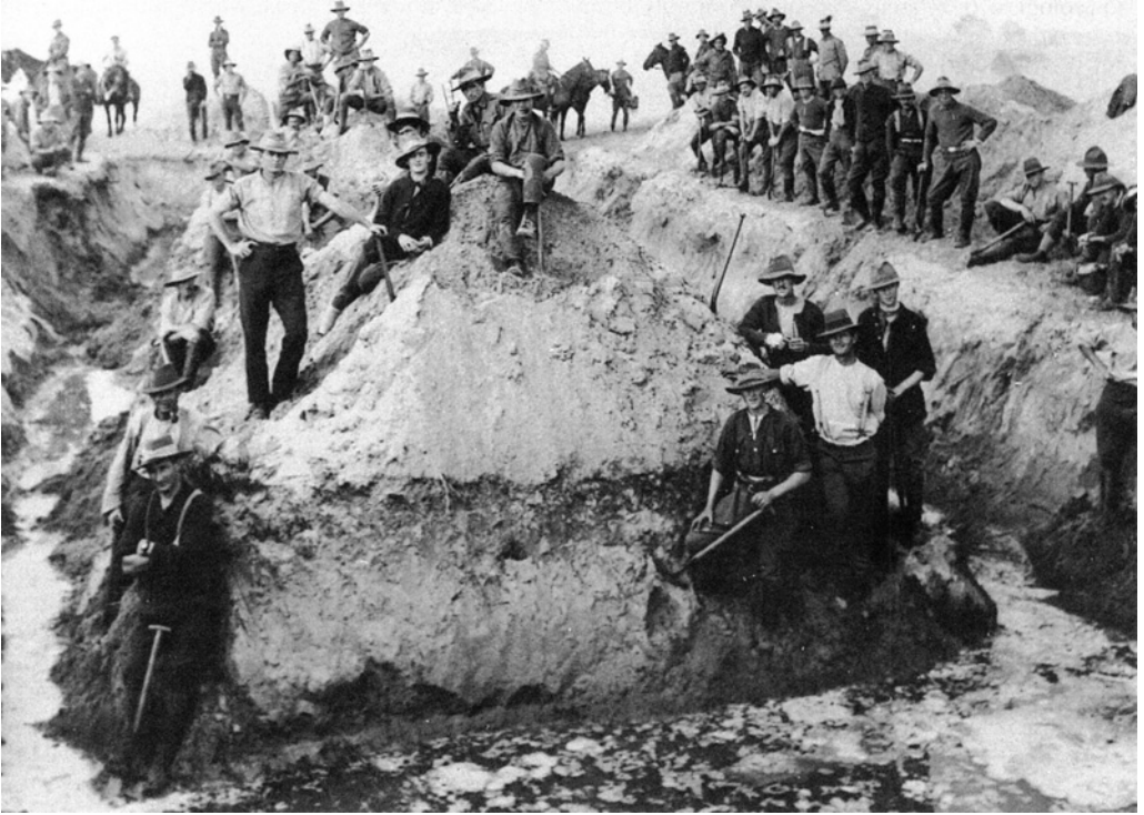
Fig. 9. Anzac (Australia/New Zealand Army Corps) troops 'digging sumps for water supply for a rest camp on the beach near Jaffa – the water was within a few yards of the sea and although brackish was quite fit to drink, not bad for coffee, but ruined tea. Horses and camels got fond of it.' Photograph (dated to 1916–1919; box F50, album 5/8B, p. 28) courtesy of the Royal Engineers Corps Library, Chatham; wording from original caption.
