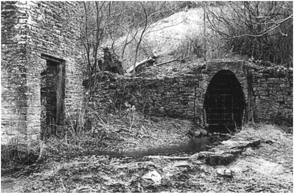
Fig. 1. Two examples of long-established drainage adits remaining long after the closures of their respective mines. (a) A 17th Century coal mine drainage adit: the portal of the Delaval Drift on Scotswood Road, Newcastle Upon Tyne, which was driven from around 1670 onwards to under-drain extensive workings to the west and north of the city of Newcastle (see Table 2). (Photo: P L Younger). (b) A 19th Century lead mine drainage adit: the Blackett Level, Allendale Town, Northumberland in 1997 (see Table 2). (Photo: A Doyle).
