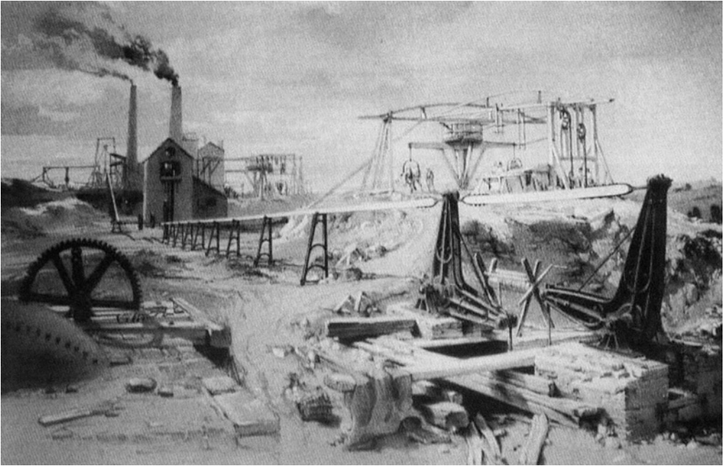
Fig. 5. Pumps for draining the Kilsby Tunnel (Bourne 1839: courtesy of the Institution of Civil Engineers Library).
