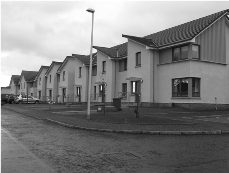
Figure 4.5 Maisonette development following renovation
