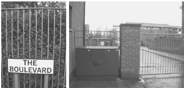
Figure 6.4 Lack of consideration for security in the positioning of street signs and utility boxes provides climbing aids for offenders
