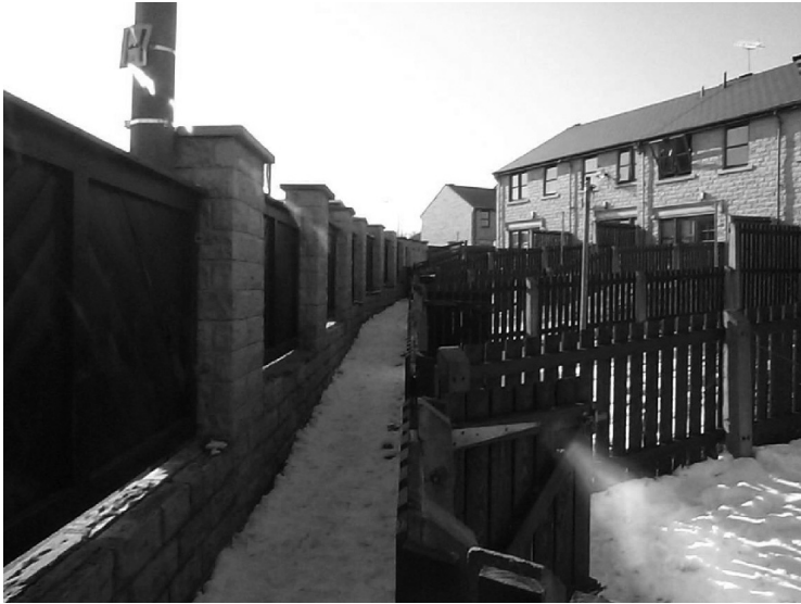
Figure 2.4 A rear footpath which would not be acceptable within SBD developments
