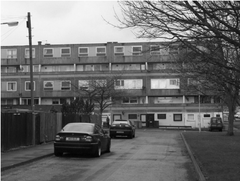
Figure 4.4 Maisonette development before demolition
