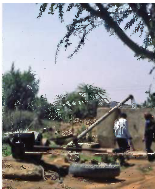
(b) Diesel-powered pumped irrigation well in Yemen. [Photo: Jac van der Gun].
