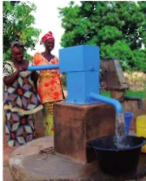
(b) Modern hand pump for community water supply in Gambia. (FairWater Blue Pump). [Photo: FairWater].
