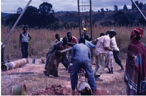
(a) Villagers drilling jointly by hand a shallow well in weathered basement rock, for community drinking water supply in Tanzania.
