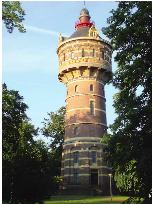
Figure 5.15 Water tower in Deventer, The Netherlands. Built in 1892 and still in use to maintain a constant pressure in the urban drinking water network. Groundwater is – after minor treatment – pumped into this tower’s reservoir, from where it enters the public water supply distribution network. [Photo: Jac van der Gun].
