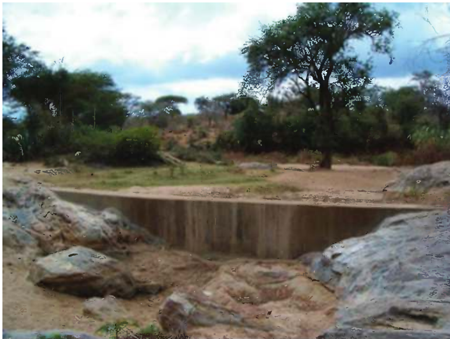
(a) Small sand dam in Kitui district, Kenya. [Photo: Sander de Haas]. The dam has created a small sand reservoir in the stream bed where flood water is stored. This can be abstracted to meet modest local water demands.
