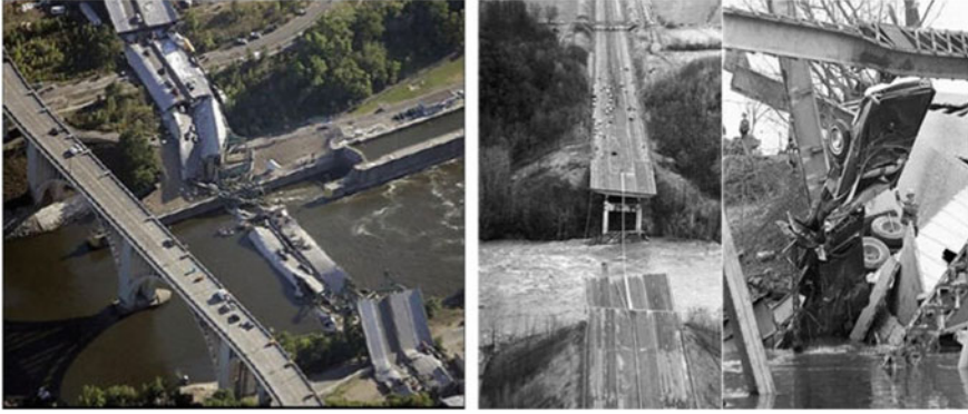
Fig. 2.2 The catastrophic failure of I-35W Bridge in Minneapolis, Minnesota after collapse on August 1, 2007 ( left ); the Point Pleasant Bridge collapse ( right )
