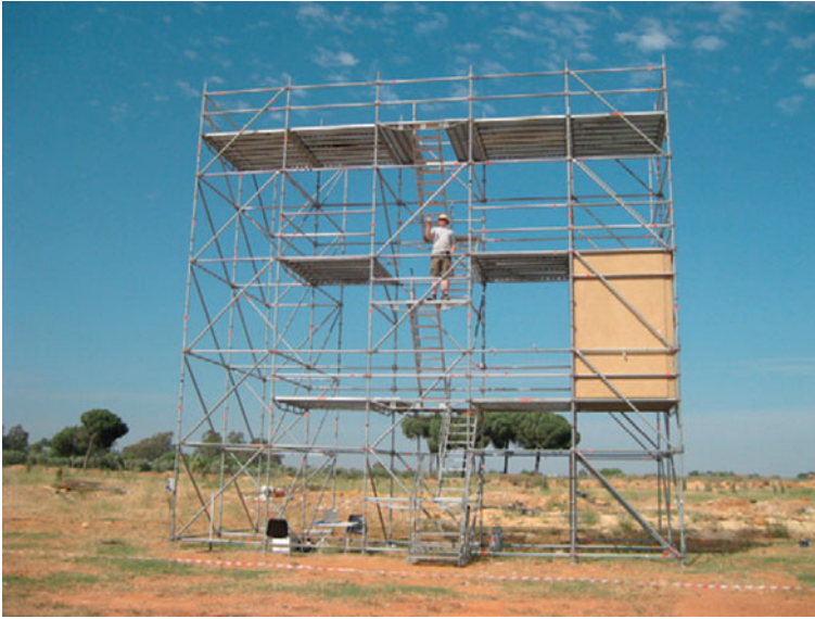
Fig. 3.11 Scenario used in the validation of the AWARE project. It was deployed at the Protec-Fire premises at Utrera, Sevilla. The photograph picture shows the structure used to simulate the building
