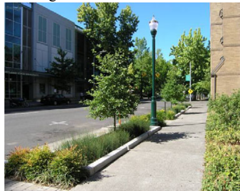
Figure 12: Green Street with Bio-Swale and Unit Pavers, Photo courtesy of Jennifer Rosales, PB
