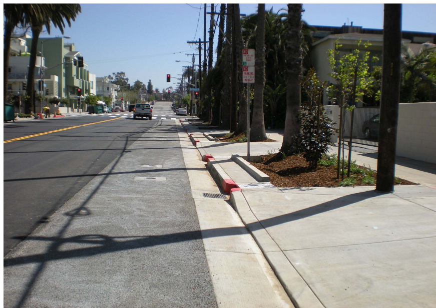
Figure 3. Project completion. Note pervious concrete lane with widened parkways, and catch basins in gutter.
