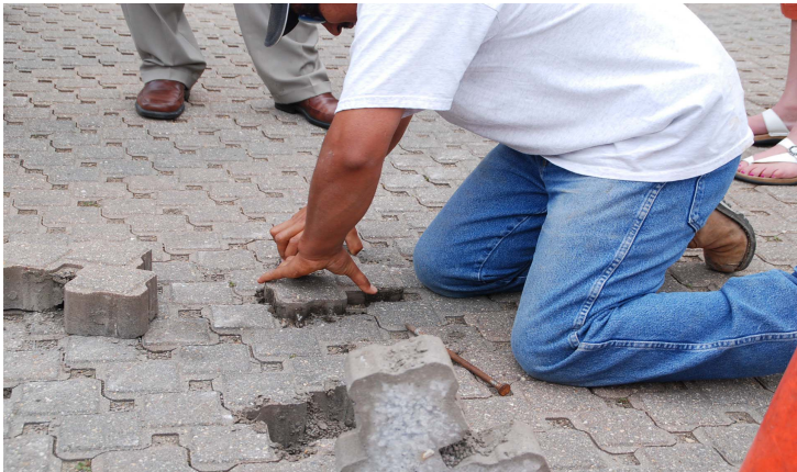
Figure 5. Six year-old paving blocks are removed from the heavily-used and never-previously-cleaned PICP parking lot at Morton Arboretum in Lisle, Illinois. Note the sediment trapped by the stone in the openings. The picture also illustrates PICP's modular construction that facilitates surface repair and access to underground utilities.
