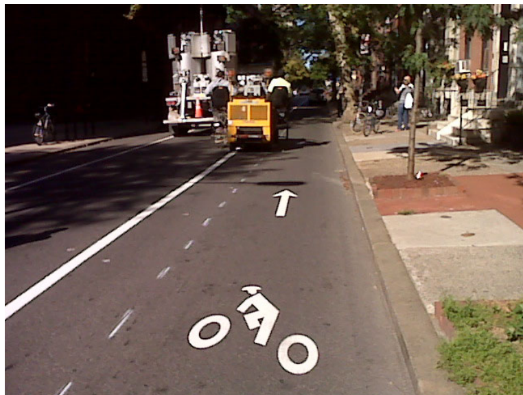
Figure 1 – Installation of Spruce and Pine bike lanes, Fall 2009.
