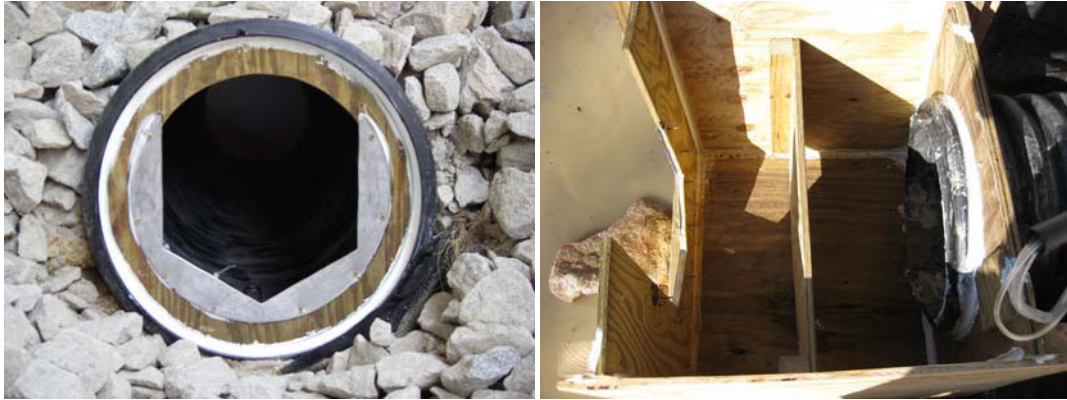
Figure 6. Monitoring installation at inlet (left) and outlet (right) of bioswale.
