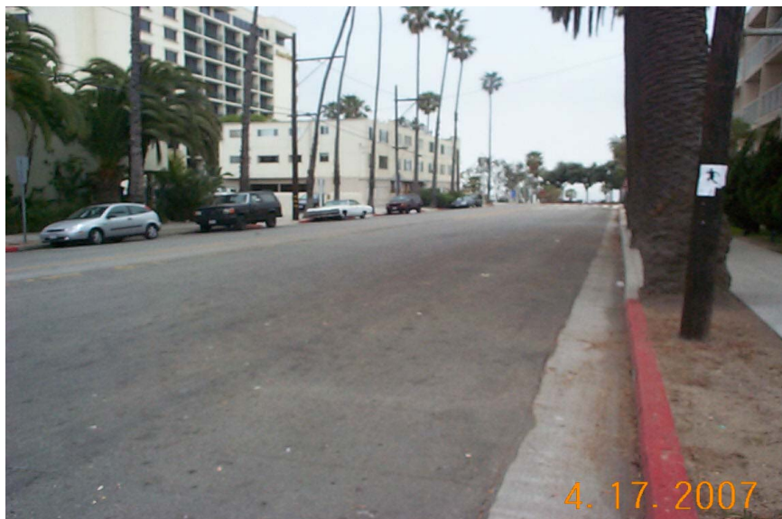
Figure 1. Bicknell Avenue before project installation. Note narrow parkway and impermeable parking lane.
