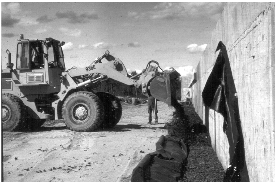
Fig. 5 Placing tire shreds using front end loader for rigid frame bridge.
