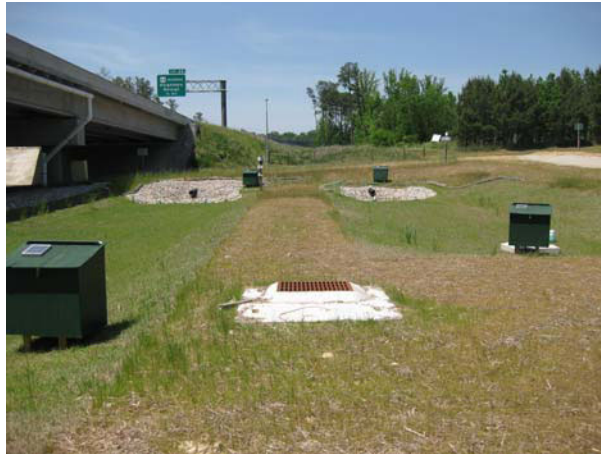
Figure 4. Standard (left) and undersized (right) bioretention cells at Mango Creek.
