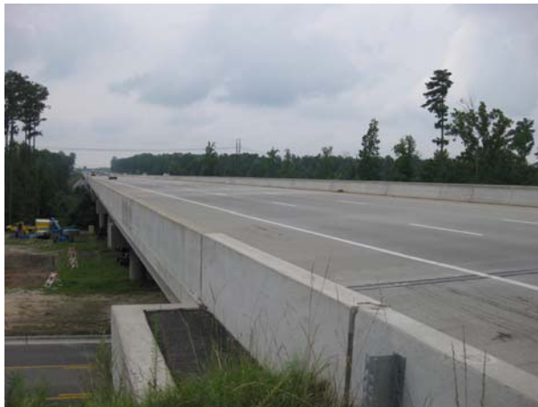
Figure 2. Mango Creek bridge deck (northbound lanes).
