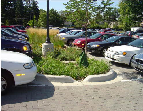
Figure 2. PICP overflow to a bioswale at Elmhurst College parking lot, Elmhurst, Illinois
