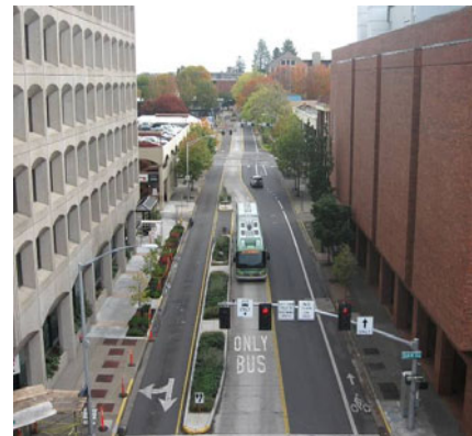
Figure 4: Franklin Corridor, Photo courtesy of Kari Turner, Pivot Architecture
