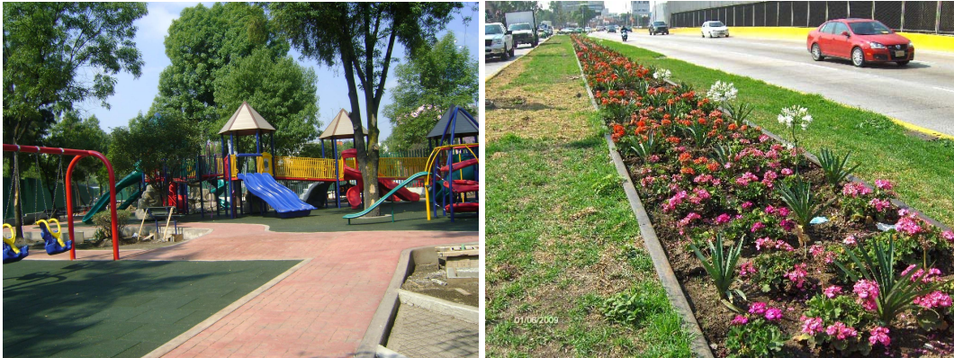
Figure 3. Construction of recreation areas and green areas
