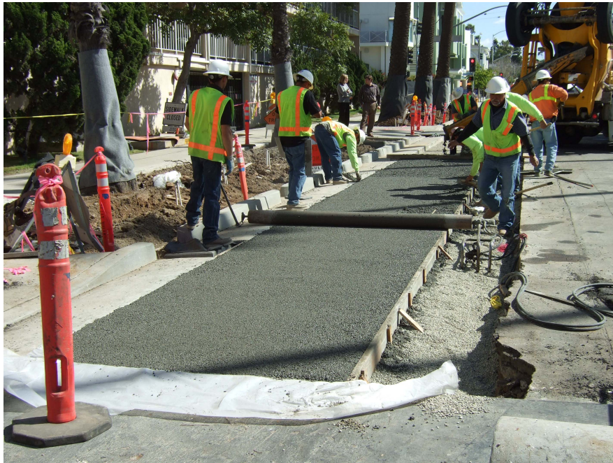
Figure 2. Installation of pervious concrete parking lane.
