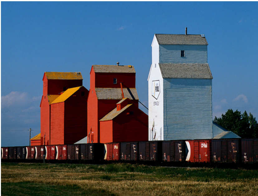
FIGURE 3.3 Grain elevators are regional businesses that store and market grain. Elevators in the northern U.S. and Canada are often constructed of wood. Employees of these facilities are exposed to hazardous grain dust.
