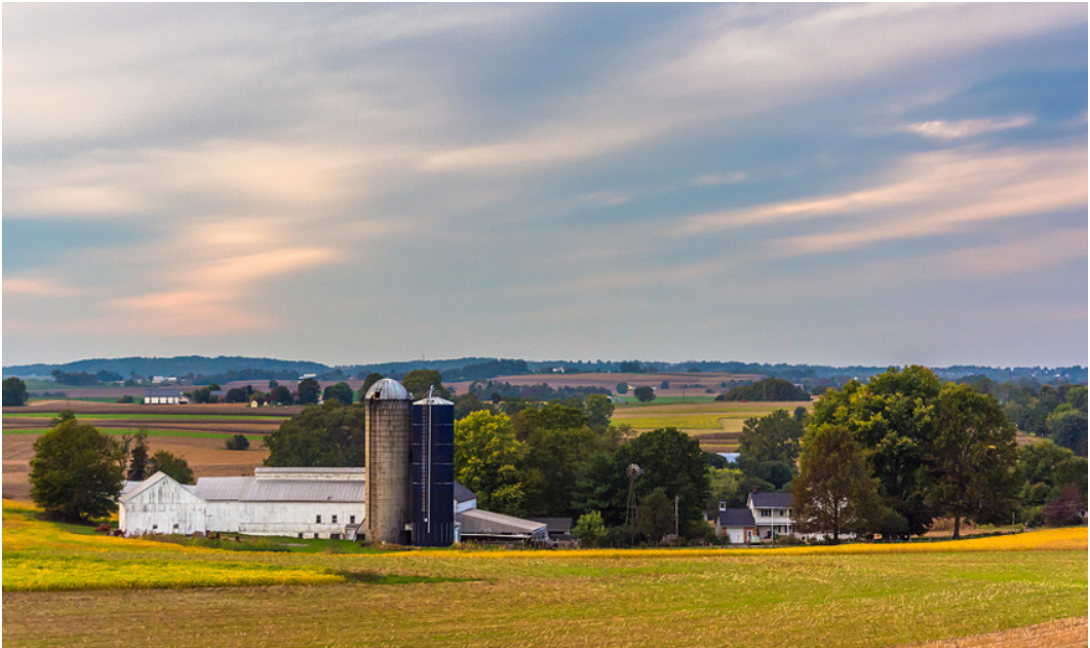
FIGURE 3.5 An oxygen-limiting silo (black) and a non-oxygen-limiting silo (gray). These present different occupational exposures to farm workers. (Source: John Bilous/Shutterstock.com.)
