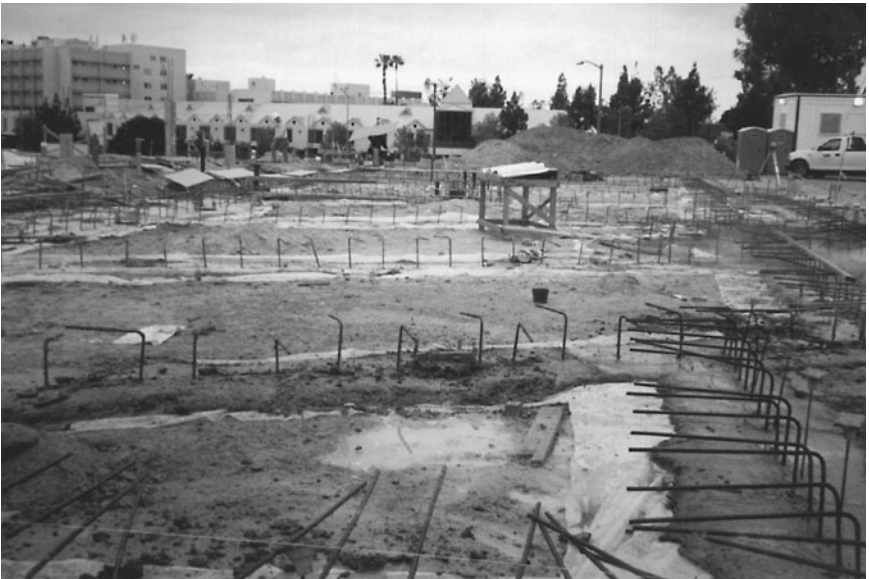
FIGURE 13.14 The concrete for the grade beams has been placed. The steel reinforcement from the grade beams will be attached to the steel reinforcement in the floor slab.
