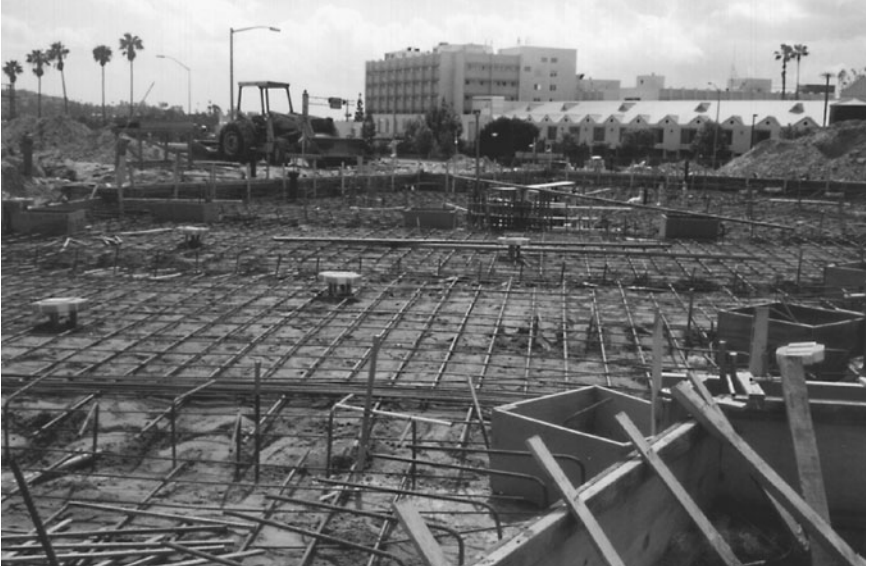
FIGURE 13.15 Positioning of the steel reinforcement for the floor slab.
