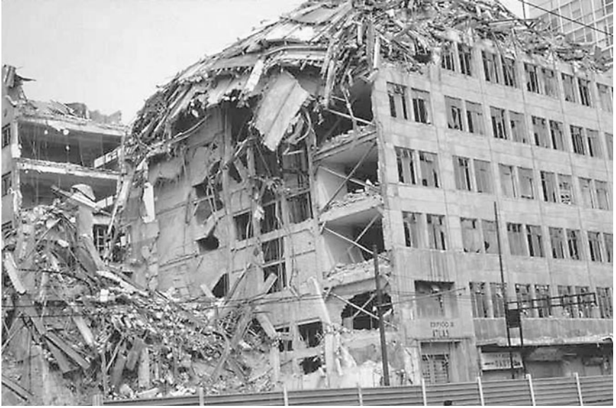
FIGURE 4.23 Building collapse in Mexico City caused by the Michoacan earthquake in Mexico on September 19, 1985. (Photograph from the Steinbrugge Collection, EERC, University of California, Berkeley.)
