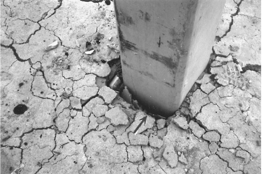
FIGURE 13.23 This prestressed concrete pile struck an underground obstruction, displaced laterally, and broke near ground surface. The arrow points to the location of the breakage.
