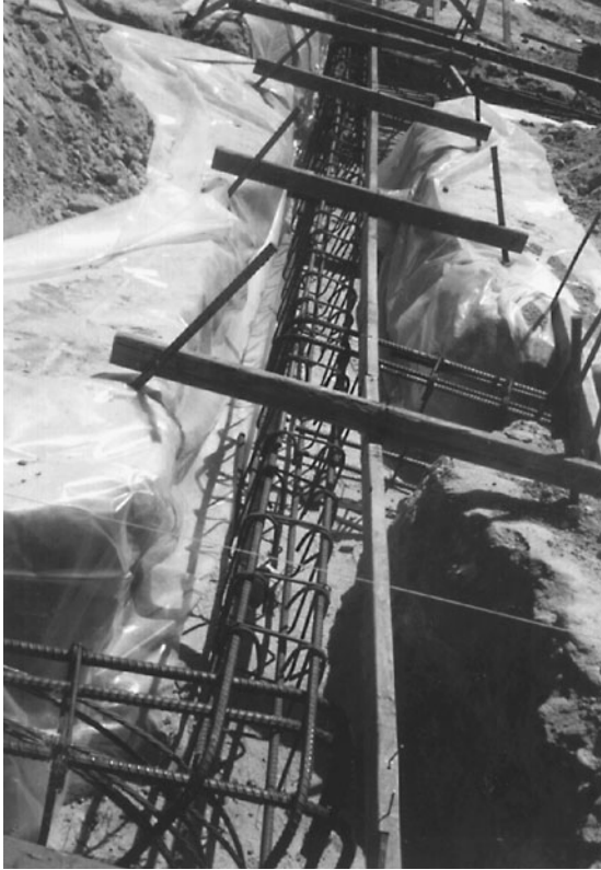
FIGURE 13.34 Overview of the steel reinforcement positioned within the grade beam excavation.
