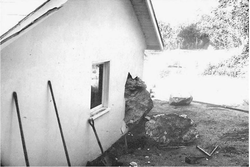
FIGURE 9.1 A rockfall that struck a house located at the mouth of Pacoima Gorge. The rockfall was caused by the San Fernando earthquake (magnitude 6.6) in California on February 9, 1971. (Photograph from the Steinbrugge Collection, EERC, University of California, Berkeley.)
