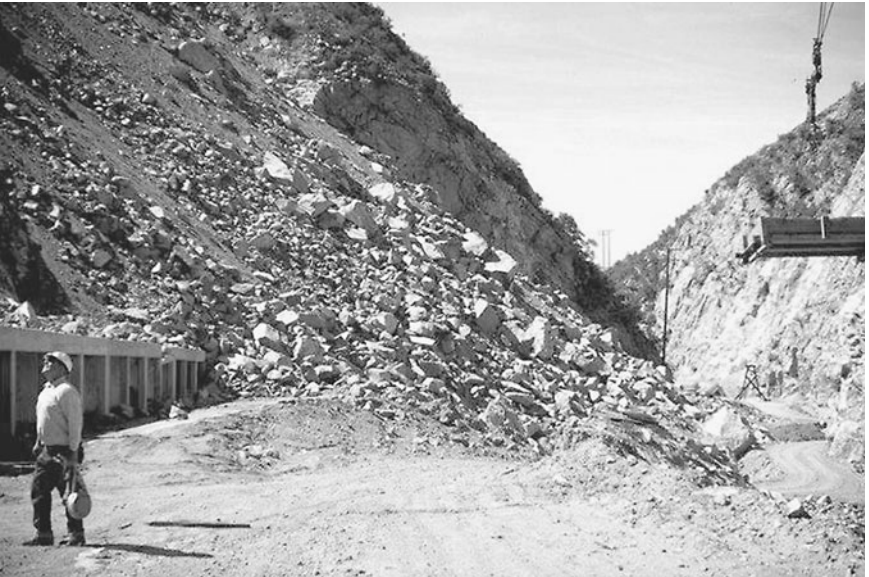
FIGURE 9.4 Rock slide at the Pacoima Dam caused by the San Fernando earthquake in California on February 9, 1971. (Photograph from the Steinbrugge Collection, EERC, University of California, Berkeley.)
