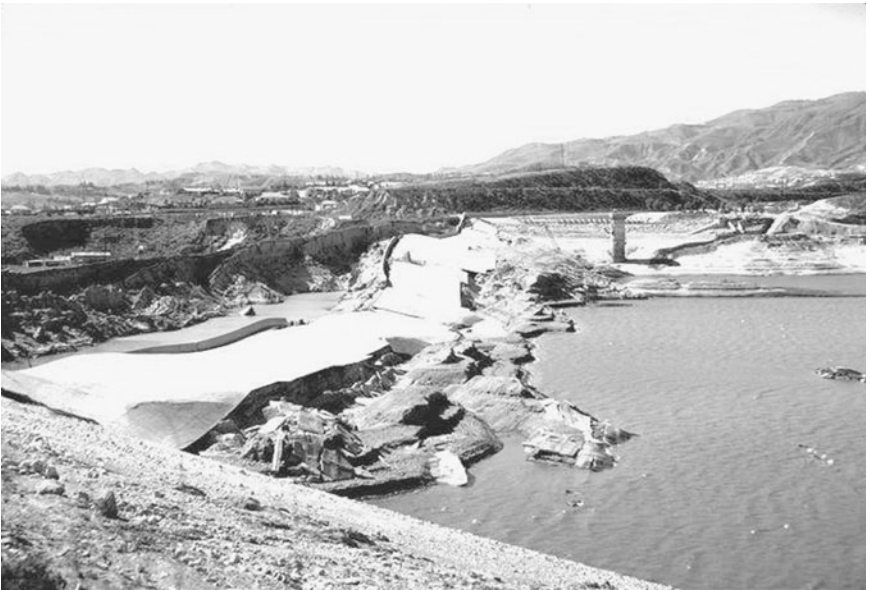
FIGURE 3.40 Flow slide of the Lower San Fernando Dam caused by the San Fernando earthquake on February 9, 1971. The photograph is a view to the west and shows the dam failure after the reservoir has been partly emptied. (Photograph from the Steinbrugge Collection, EERC, University of California, Berkeley.)
