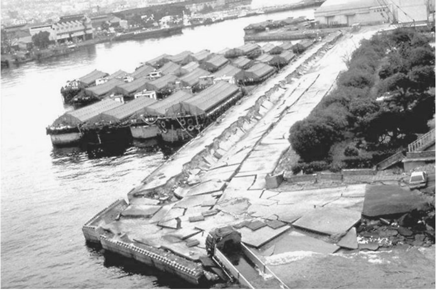
FIGURE 3.30 Retaining wall damage caused by the Kobe earthquake on January 17, 1995. The site is the east bank of the Maya-ohashi Bridge (Harbor Expressway). Liquefaction caused significant lateral displacement of the retaining wall, which in turn created a depression behind the wall and dropped a large truck halfway into the water. (Photograph from the Kobe Geotechnical Collection, EERC, University of California, Berkeley.)
