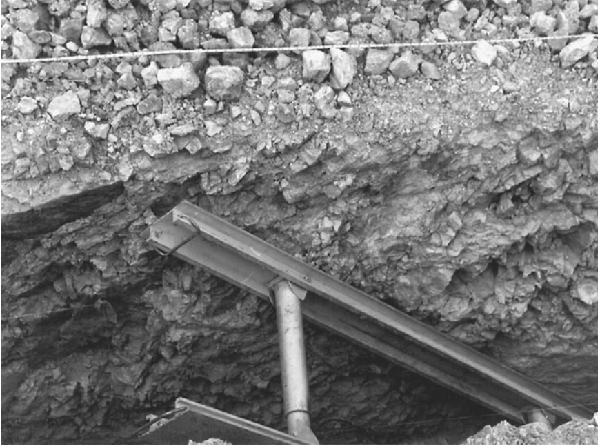
FIGURE 5.9 Close-up view of trench excavation.
