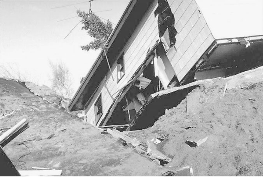
FIGURE 3.49 Damage caused by movement of the Turnagain Heights landslide during the Prince William Sound earthquake in Alaska on March 27, 1964. (Photograph from the Steinbrugge Collection, EERC, University of California, Berkeley.)
