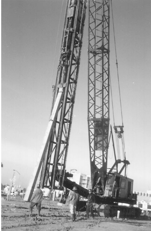
FIGURE 13.20 Pile-driving equipment. A prestressed concrete pile is in the process of being hoisted into position.
