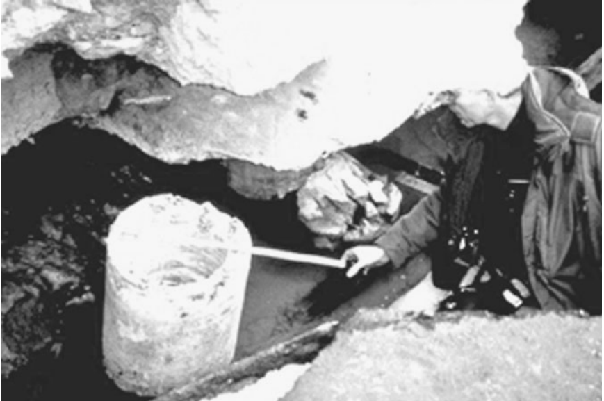
FIGURE 13.36 The top of the concrete pile separated from the concrete pile cap during the Kobe earthquake on January 17, 1995. (Photograph from the Kobe Geotechnical Collection, EERC, University of California, Berkeley.)
