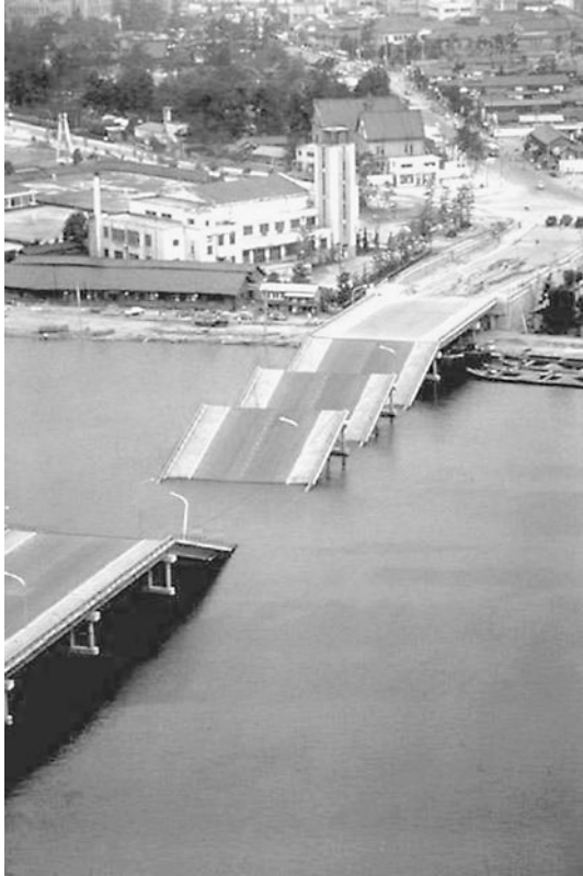
FIGURE 3.25 Collapse of the Showa Bridge during the Niigata earthquake on June 16, 1964. (Photograph from the Godden Collection, EERC, University of California, Berkeley.)
