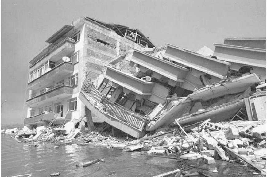
FIGURE 3.18 Flooding caused by regional subsidence associated with the Izmit (Turkey) earthquake on August 17, 1999. (Photograph from the Izmit Collection, EERC, University of California, Berkeley.)
