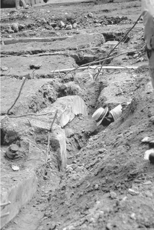
FIGURE 8.6 The building foundation shown above was constructed of individual footings that were interconnected with concrete tie beams. The building collapsed during the Caracas earthquake in Venezuela on July 29, 1967. When the foundation was exposed, it was discovered that the spread footings had punched downward into the soil. Note that the tie beam at the center of the photograph was bent and pulled downward when the footing punched into the underlying soil. (Photograph from the Steinbrugge Collection, EERC, University of California, Berkeley.)
