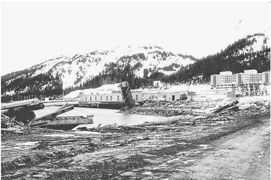
FIGURE 4.1 Overview of damage caused by a tsunami generated during the Prince William Sound earthquake in Alaska on March 27, 1964. Note the tilted tower in the background. (Photograph from the Steinbrugge Collection, EERC, University of California, Berkeley.)
