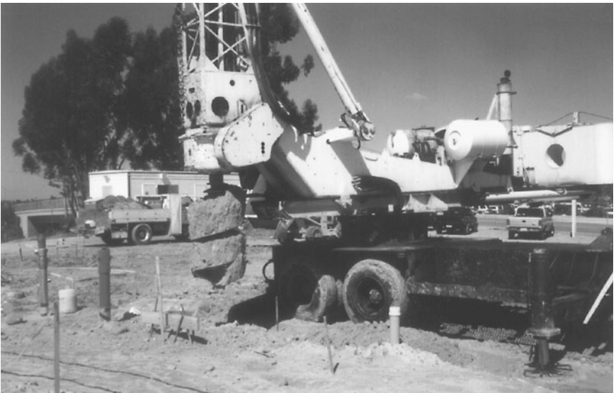
FIGURE 13.6 Truck-mounted auger drill rig used to excavate piers.
