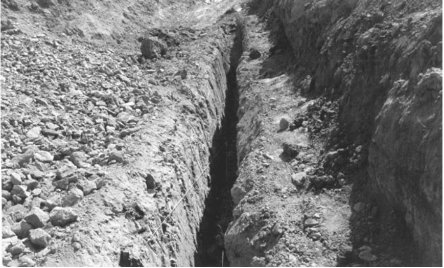
FIGURE 5.8 Backhoe trench for a fault study.
