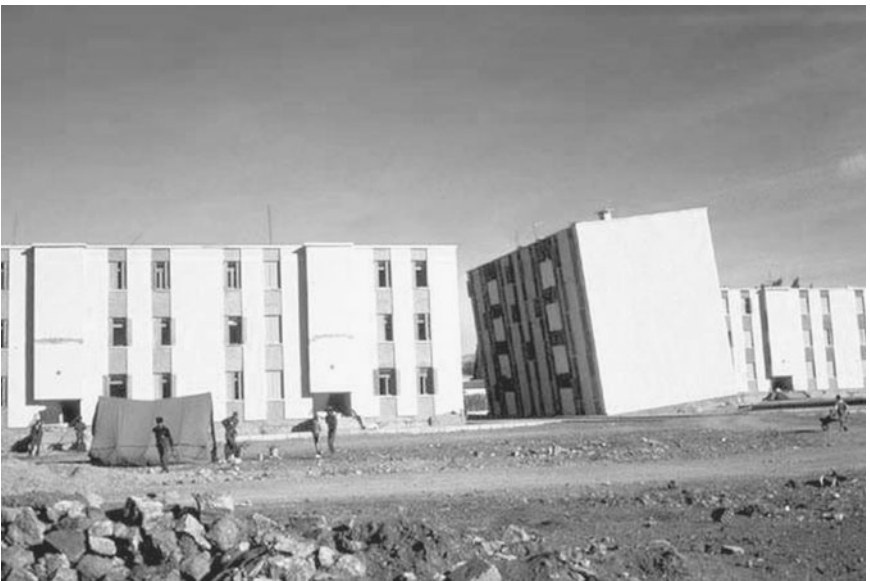
FIGURE 4.11 Building tilting and damage caused by a soft story due to a ground-floor crawl space. The damage occurred during the El Asnam earthquake in Algeria on October 10, 1980. (Photograph from the Godden Collection, EERC, University of California, Berkeley.)
