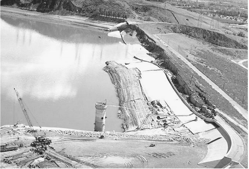
FIGURE 3.39 Flow slide of the Lower San Fernando Dam caused by the San Fernando earthquake on February 9, 1971. The photograph is a view to the east, and the main flow slide is at the eastern end of the dam. (Photograph from the Steinbrugge Collection, EERC, University of California, Berkeley.)
