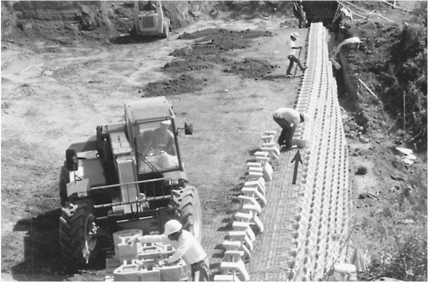
FIGURE 10.6 Installation of a mechanically stabilized earth retaining wall. The arrow points to the wall facing elements, which are in the process of being installed.
