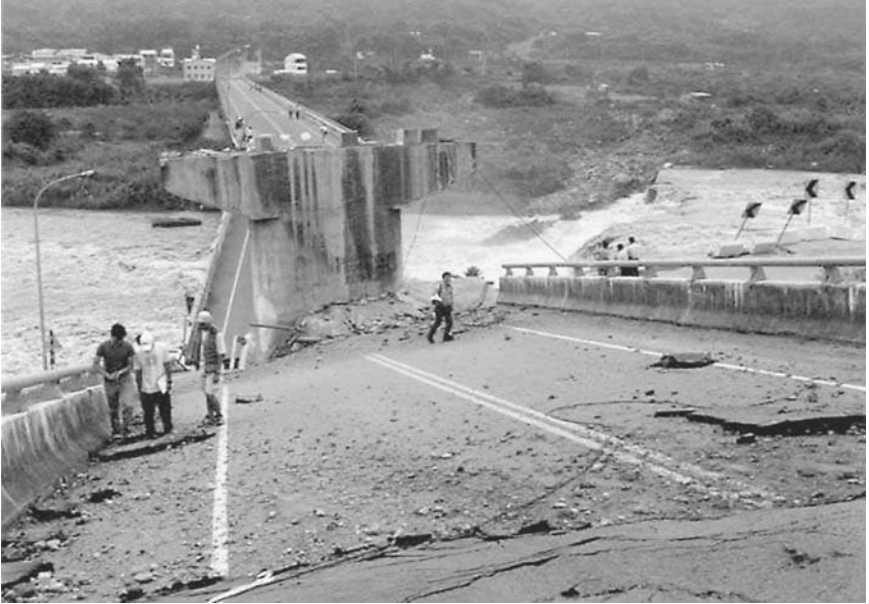
FIGURE 3.11 Another view of the collapsed bridge north of Fengyuen caused by surface fault rupture associated with the Chi-chi (Taiwan) earthquake on September 21, 1999. Note that the surface faulting has created the waterfall on the right side of the bridge. (Photograph from the USGS Earthquake Hazards Program, NEIC, Denver.)
