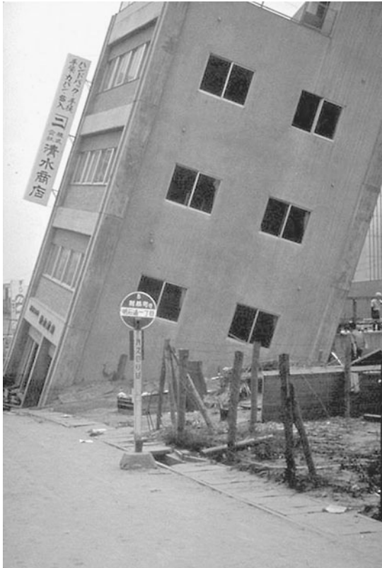
FIGURE 3.23 Settlement and tilting of a building located in Niigata, Japan. The building suffered liquefaction-induced settlement and tilting during the Niigata earthquake on June 16, 1964. (Photograph from the Steinbrugge Collection, EERC, University of California, Berkeley.)
