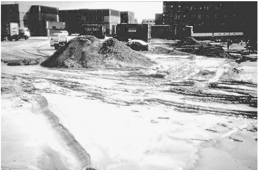
FIGURE 3.26 The interiors of the Rokko and Port islands settled as much as 1 m with an average of about 0.5 m due to liquefaction caused by the Kobe earthquake on January 17, 1995. This liquefaction-induced settlement was accompanied by the eruption of large sand boils that flooded many areas and covered much of the island with sand boil deposits as thick as 0.5 m. In this photograph, a stockpile has been created out of some of this sand. (Photograph from the Kobe Geotechnical Collection, EERC, University of California, Berkeley.)
