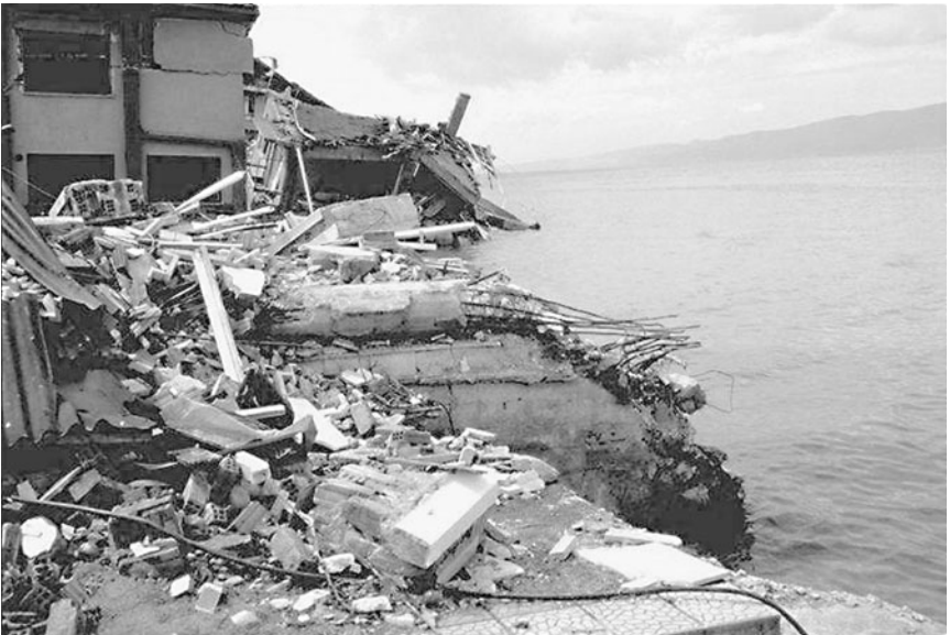
FIGURE 3.17 Flooding caused by regional subsidence associated with the Izmit (Turkey) earthquake on August 17, 1999. (Photograph from the Izmit Collection, EERC, University of California, Berkeley.)
