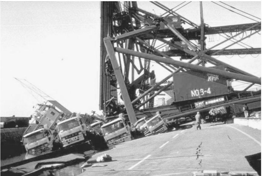
FIGURE 3.34 Collapse of a crane due to about 2 m of lateral movement of the retaining wall on Rokko Island. There was also about 1 to 2 m of settlement behind the retaining wall when it moved outward during the Kobe earthquake on January 17, 1995. (Photograph from the Kobe Geotechnical Collection, EERC, University of California, Berkeley.)
