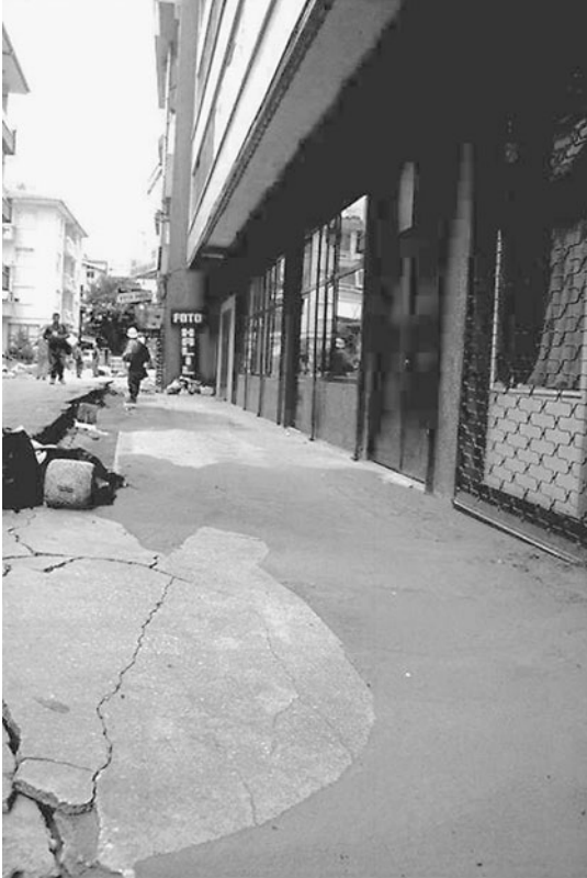
FIGURE 7.5 Surface fissure caused by the Izmit earthquake in Turkey on August 17, 1999. Note that liquefied soil flowed out of the fissure. (Photograph from the Izmit Collection, EERC, University of California, Berkeley.)
