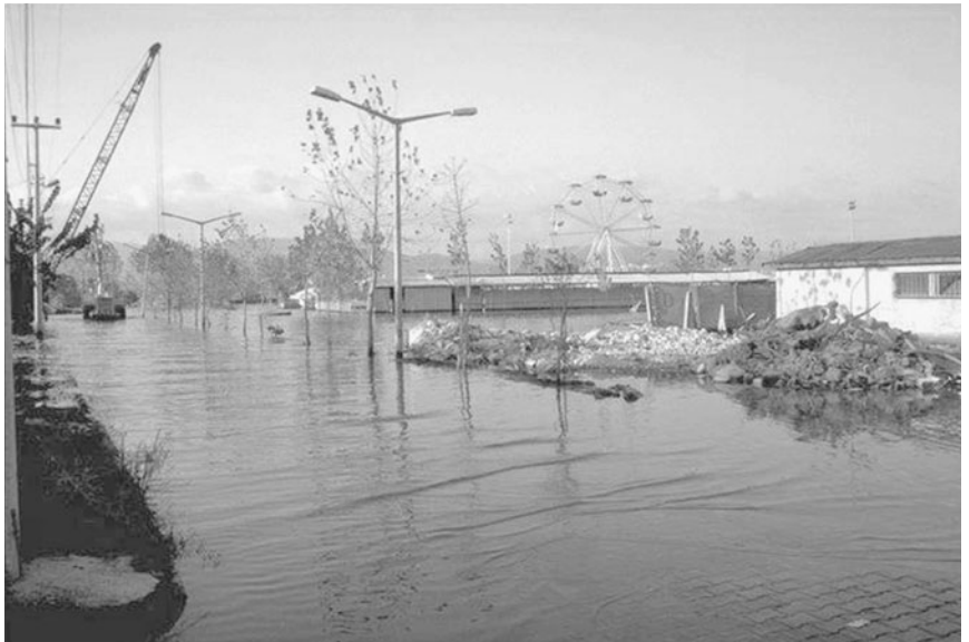
FIGURE 3.15 Flooding caused by regional subsidence associated with the Izmit (Turkey) earthquake on August 17, 1999. (Photograph from the Izmit Collection, EERC, University of California, Berkeley.)
