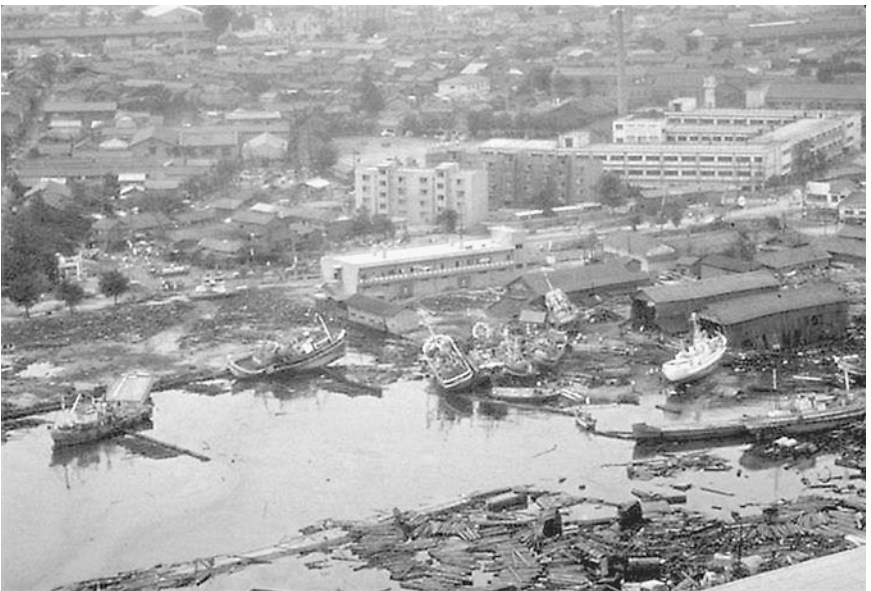
FIGURE 3.56 Tsunami damage caused by the Niigata earthquake in Japan on June 16, 1964. (Photograph from the Steinbrugge Collection, EERC, University of California, Berkeley.)
