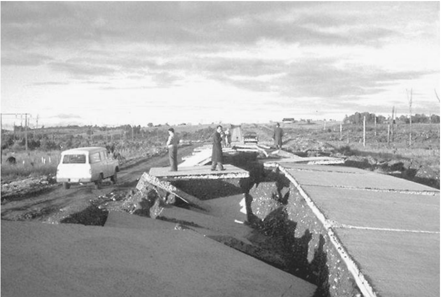
FIGURE 11.6 This picture shows the failure of a concrete surfaced highway due to an earthquake-induced foundation failure. This area was observed to be a marshy region. This main highway is located 6 km north of Perto Montt. The May 1960 Chile earthquake (moment magnitude = 9.5) caused the highway damage. (Photograph from the Steinbrugge Collection, EERC, University of California, Berkeley.)
