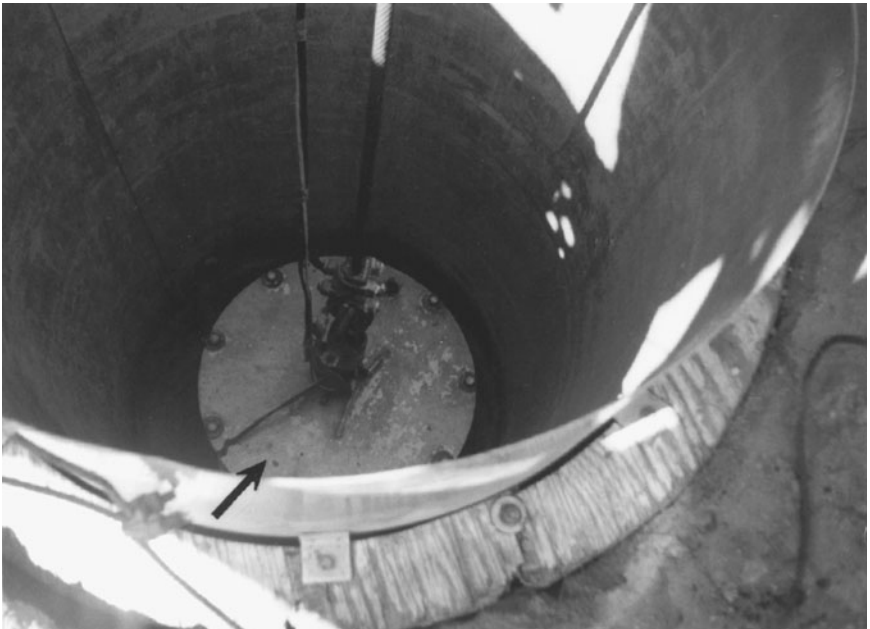
FIGURE 5.5 Down-hole logging. Note that the arrow points to the top of the steel cage used for the down-hole logging.
