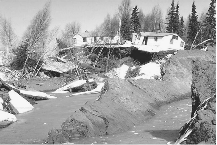
FIGURE 3.51 Damage caused by movement of the Turnagain Heights landslide during the Prince William Sound earthquake in Alaska on March 27, 1964. (Photograph from the Steinbrugge Collection, EERC, University of California, Berkeley.)
