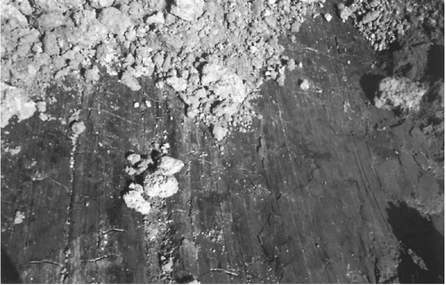
FIGURE 9.7 Photograph of the slide plane, which was exposed during the stabilization of the Niguel Summit landslide. Note that the direction of movement of the landslide can be inferred by the direction of striations in the slide plane.
