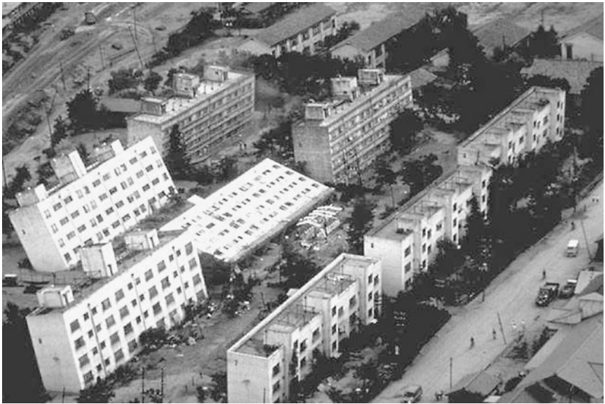
FIGURE 3.20 Kawagishi-cho apartment buildings located in Niigata, Japan. The buildings suffered liquefaction-induced bearing capacity failures during the Niigata earthquake on June 16, 1964. (Photograph from the Godden Collection, EERC, University of California, Berkeley.)
