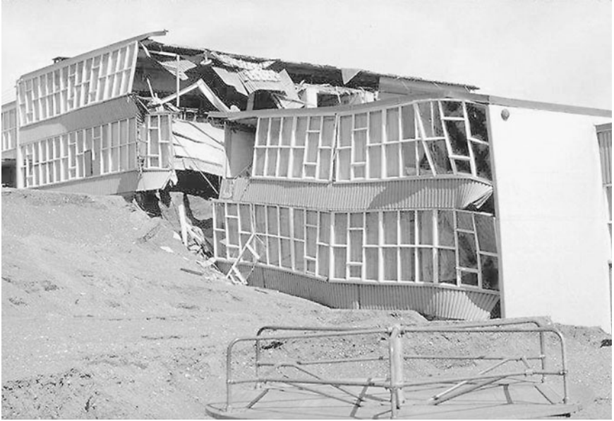
FIGURE 3.53 Close-up view of damage to the Government Hill School located at the head of a landslide caused by the Prince William Sound earthquake in Alaska on March 27, 1964. (Photograph from the Steinbrugge Collection, EERC, University of California, Berkeley.)
