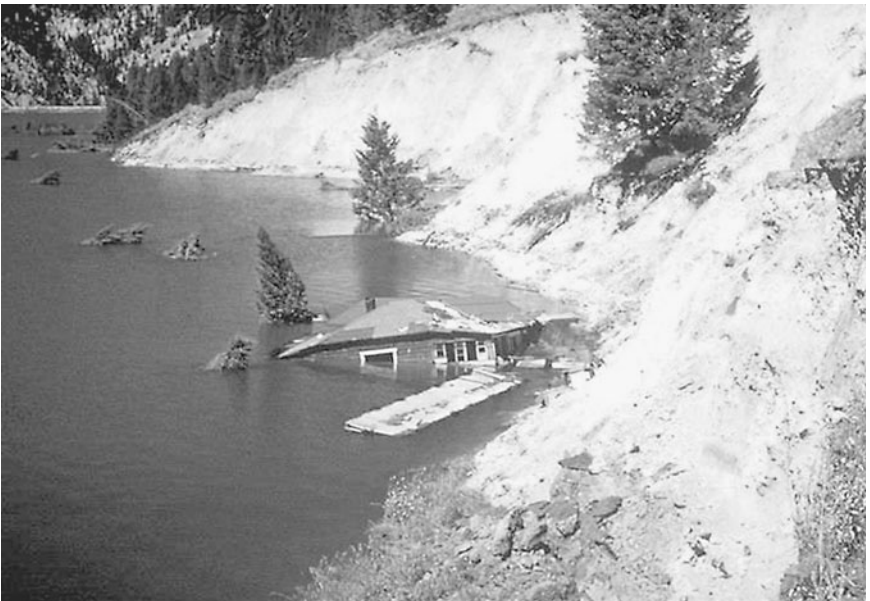
FIGURE 3.59 The building in the water was formerly on the shore about one-quarter mile up the lake. The house was apparently jarred from its foundation by the earthquake and then washed into the lake by the seiche generated during the Hebgen Lake earthquake in Montana on August 17, 1959. The house later drifted into the earthquake-created harbor shown in the above photograph. (Photograph from the Steinbrugge Collection, EERC, University of California, Berkeley.)
