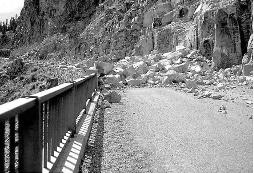
FIGURE 9.3 A large rockfall caused by the Hebgen Lake earthquake in Montana on August 17, 1959. (Photograph from the Steinbrugge Collection, EERC, University of California, Berkeley.)
