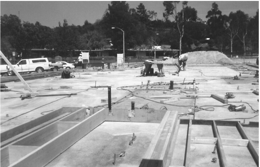
FIGURE 13.16 Concrete for the floor slab has been placed.
