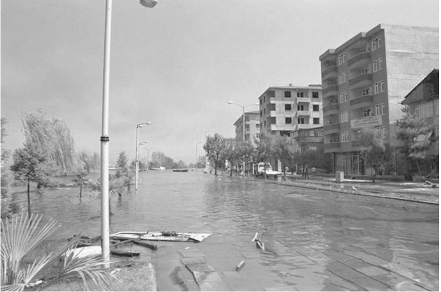
FIGURE 3.14 Flooding caused by regional subsidence associated with the Izmit (Turkey) earthquake on August 17, 1999. (Photograph from the Izmit Collection, EERC, University of California, Berkeley.)
