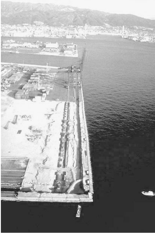
FIGURE 3.32 Retaining wall that moved outward about 2 to 3 m (7 to 10 ft), creating a depression behind the wall that was about 3 m (10 ft) deep. The cause of the retaining wall movement was liquefaction during the Kobe earthquake on January 17, 1995. (Photograph from the Kobe Geotechnical Collection , EERC, University of California, Berkeley.)
