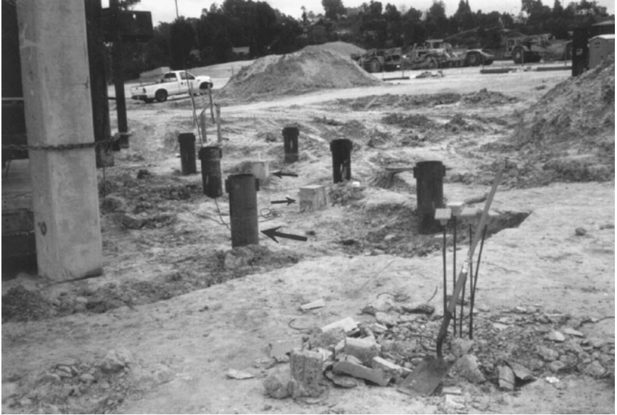
FIGURE 13.24 Pile load test. The small arrows point to the prestressed concrete piles, which will be subjected to a load test. The large arrow points to one of the six anchor piles.
