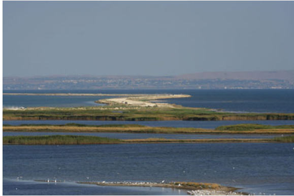
Photo 7.13 Tuzla dam constructed from the Russian side of the Kerch Strait in October–November 2003 (Photo by author)
