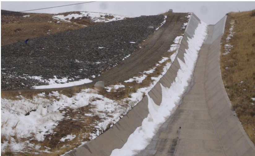
Photo 4. Overview of the chute and repair area from the stilling basin
