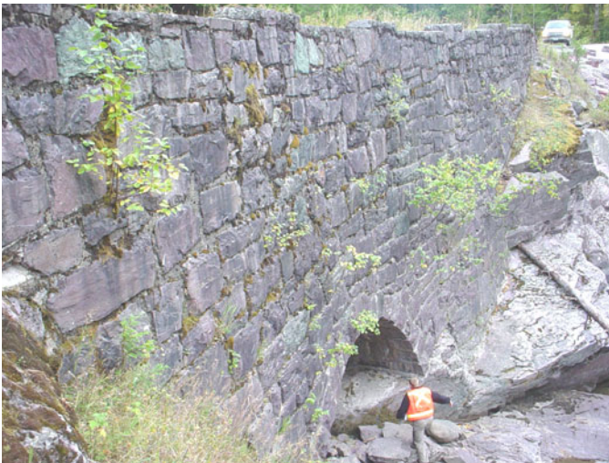
FIG. 5. A retaining wall with dual functions at Glacier National Park.
