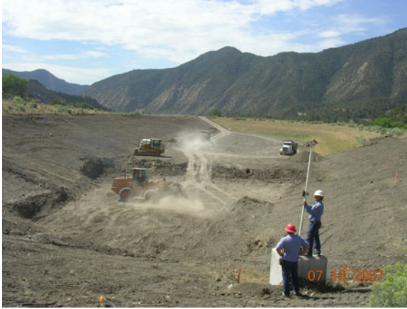
Excavation for Construction of the Soil Filter
