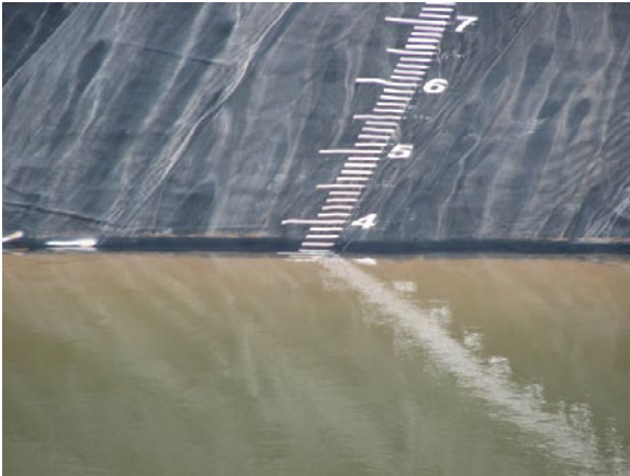
Staff Gauge During Initial Fill of RCC Reservoir No. 1
