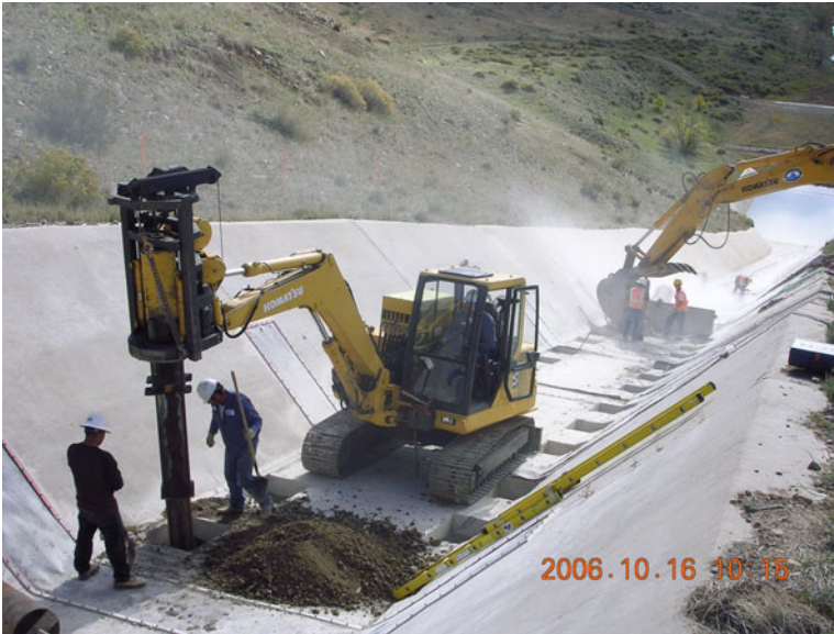
Photo 1. Drilled Pier Installation
