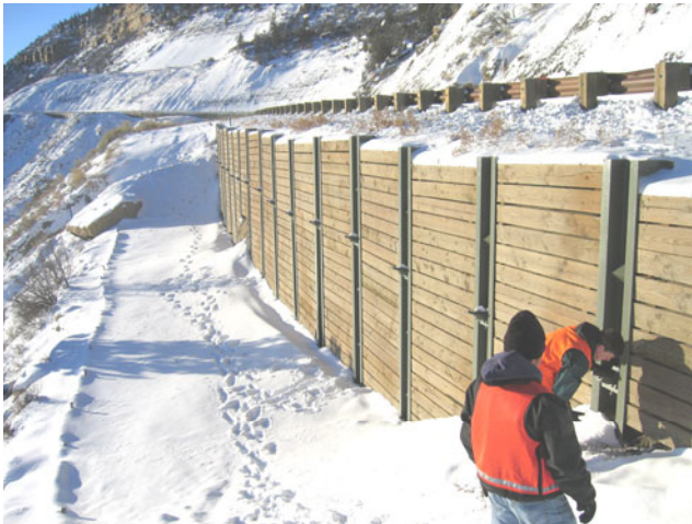
FIG. 1. Retaining wall inspection at Mesa Verde National Park.
