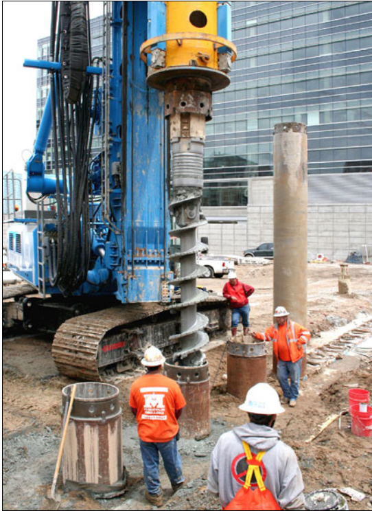
Figure 4: Secant wall installation
