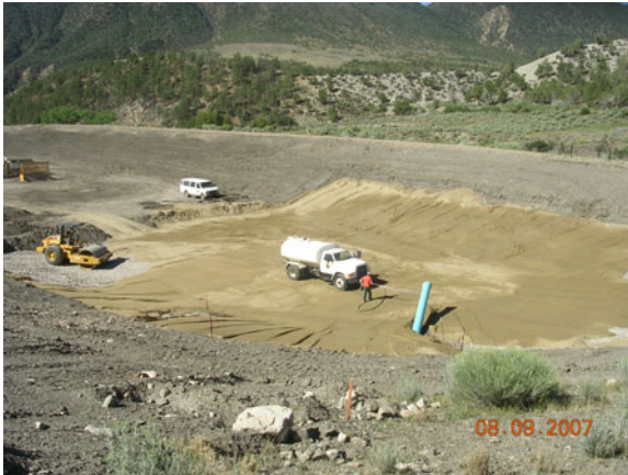
Construction of Two Stage Soil Filter
