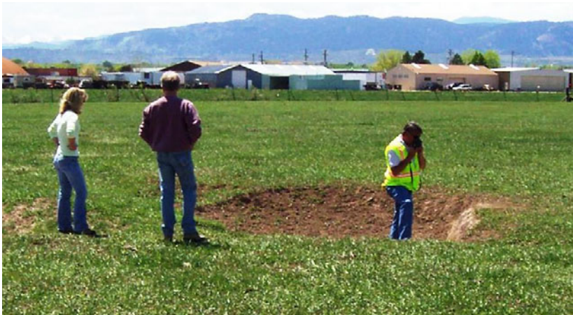
FIG. 4. Large sinkhole features in beet spoil slurry deposit, Fort Collins, CO.
