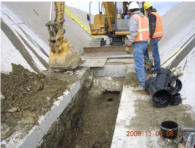
Photo 2. Underdrain Replacement
