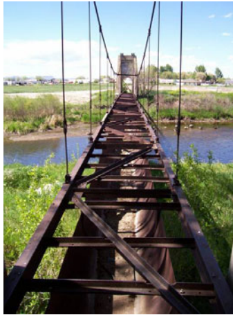
FIG. 2. A flume for conveying beet spoils across the Cache la Poudre River, Fort Collins, CO.
