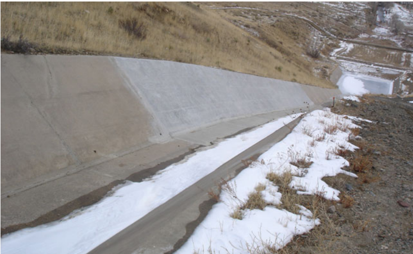
Photo 6. Overview of the chute and repair area from the crest
