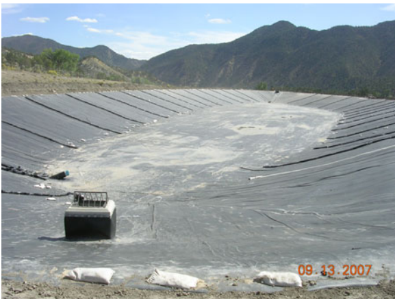
RCC Reservoir No. 1 with Hypalon Liner Installed
