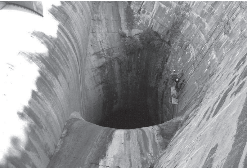
FIG. 7. Rope access work in the intake
