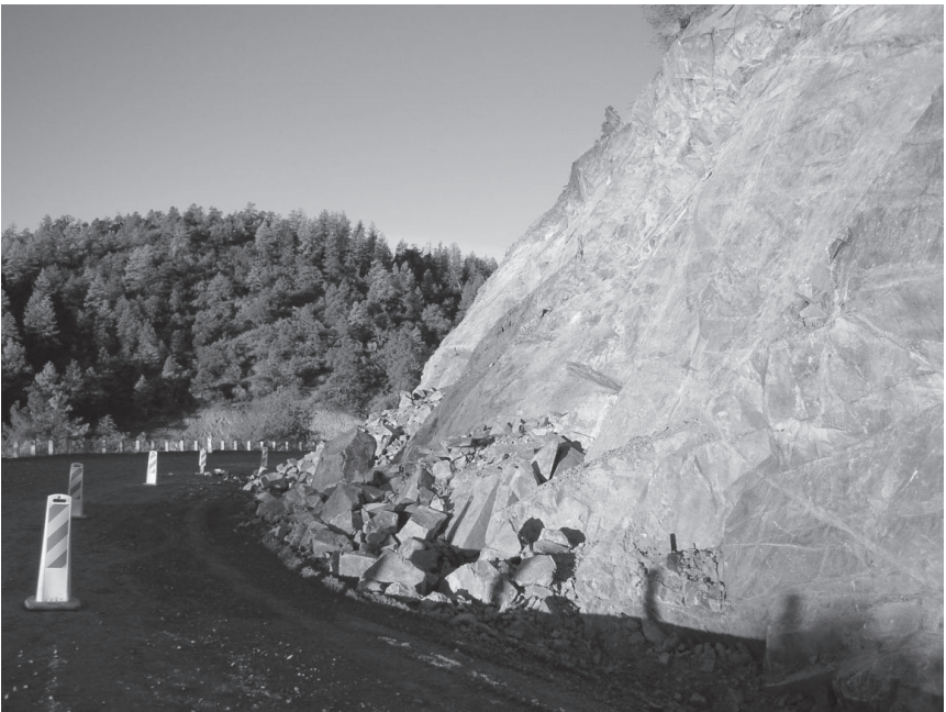
FIG 4. New slope created by widening and straightening to increase roadway capacity and traffic safety
