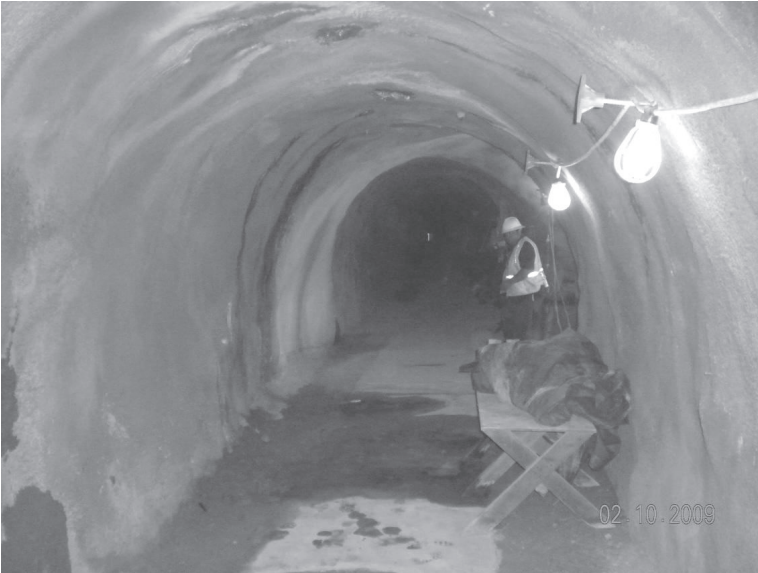
FIG. 4. Completed Emergency Tunnel Repair
