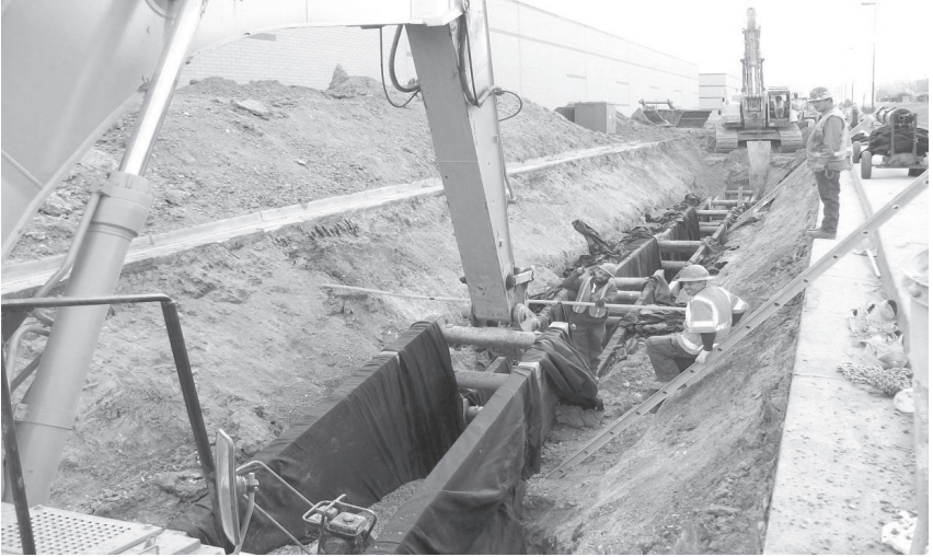
Photo 5: Underdrain Systems Installation
