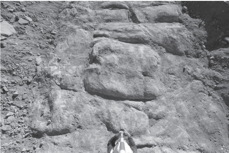
FIG. 1. Photogrammetric image being taken along the spillway foundation
