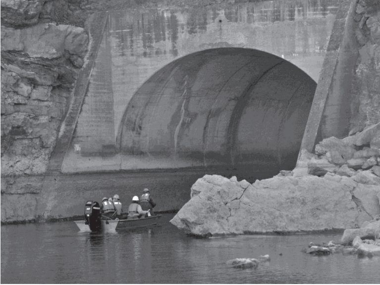
FIG. 6. Boat access at the downstream portal
