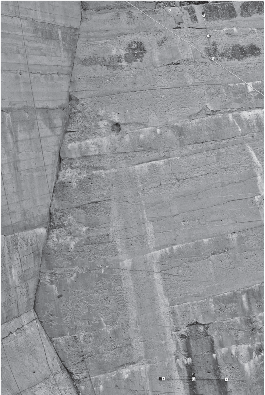
FIG. 4. Scale bars on the intake back wall (right)
