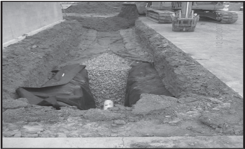
Photo 3: Underdrain system installation
