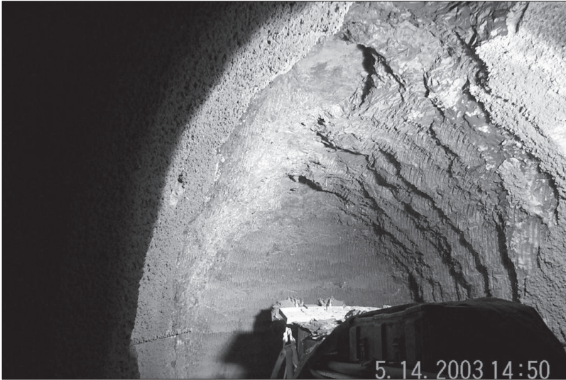
FIG. 10. Standley Lake Tunnel (note slickenside and overbreak of claystone in crown)
