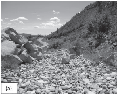
FIG 3. Examples at Mesa Verde National Park where ditch effectiveness and distance from travel lanes effectively confines rockfall to the fallout area, reducing the consequence of failure
