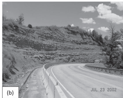
FIG 3. Examples at Mesa Verde National Park where ditch effectiveness and distance from travel lanes effectively confines rockfall to the fallout area, reducing the consequence of failure
