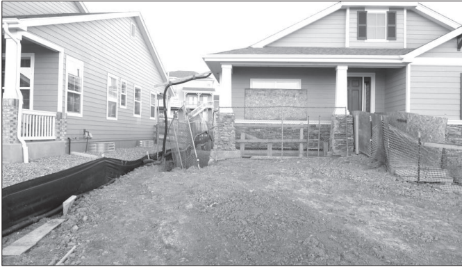
FIG. 3. Vista Ridge, Erie, Colorado. Excavating around house foundation (note the ladder)
