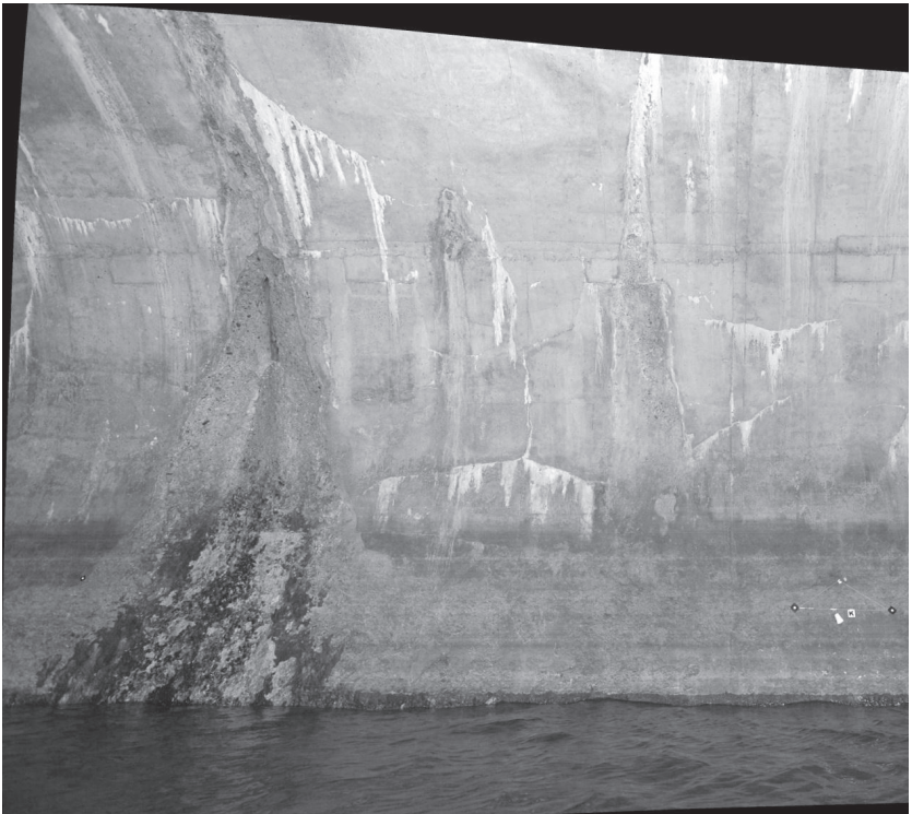
FIG. 3. Epipolar image of tunnel wall with scale bar on the right (above)
