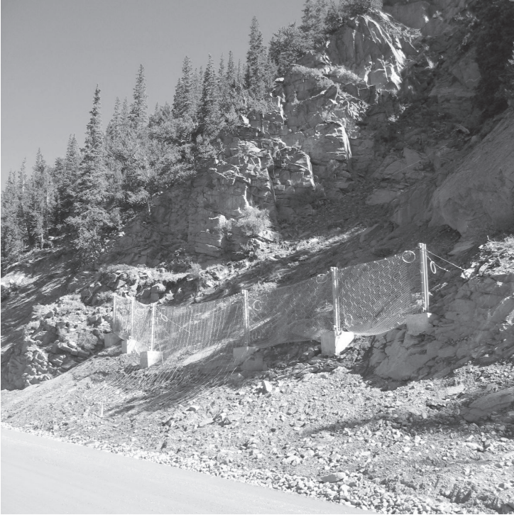
FIG 7. A rockfall fence installed on Guanella Pass Road
