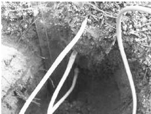
Fig. 6.3 Temperature sensors just after installation
