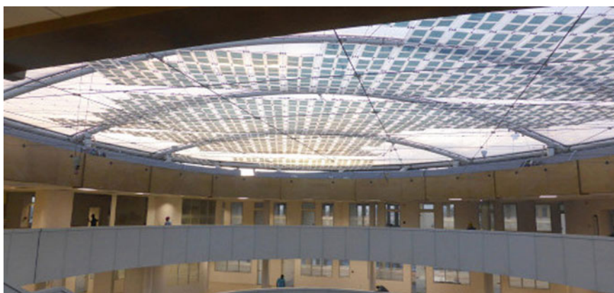
Fig. 2.39 The BIOPV array at the African Union building contains 445 Belectric PSC solar modules
