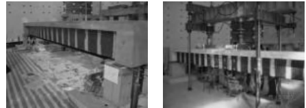
(a) Prestressed CFRP sheet before bonding to the bottom of the beam and the test set-up
