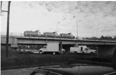
Figure 17. Trucks being positioned for static load tests of Joffre Bridge.
