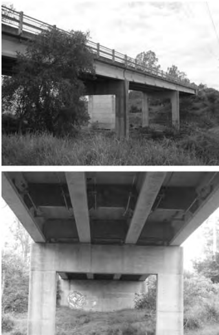
Figure 1. Photos of Tenthill bridge.
