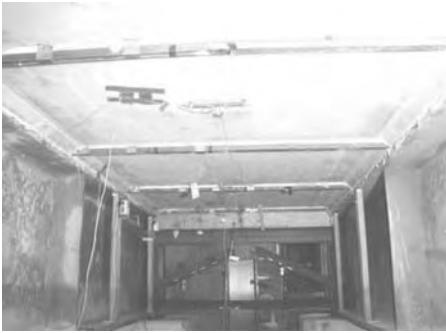
Figure 7(a). Typical bottom view of Segments B & C and instrumentation.
