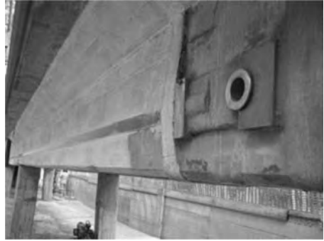
Figure 16. Anchorage on the tension side.
