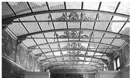
Figure 2. View of undamaged cast iron structure.
