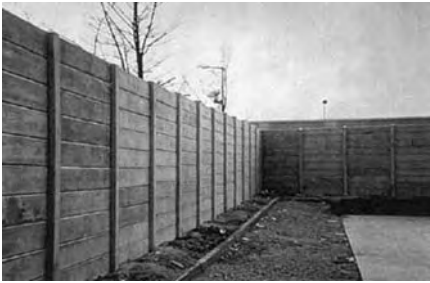
Figure 3. FRP reinforced post and panel fencing around a transmitter (courtesy EUROCRETE project).
