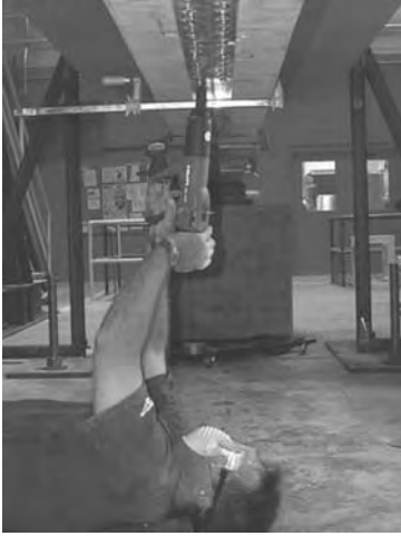
Figure 10. Attaching MF-FRP strip to T-beams.
