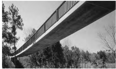
Figure 5. Prestressed FRP cables used in a ribbon bridge in Japan.
