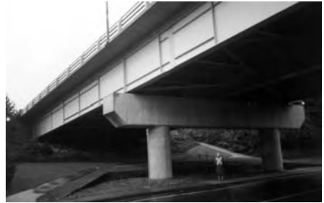
Figure 19a. Portage Creek Bridge.
