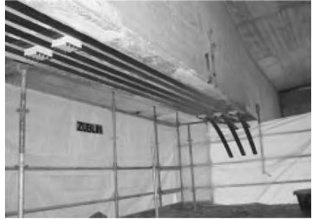
Figure 8. Applied CarboDur CFRP plates.
