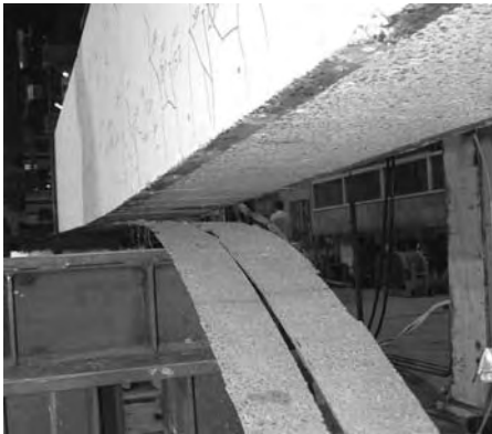
Figure 14. Debonding failure in beam B3.
