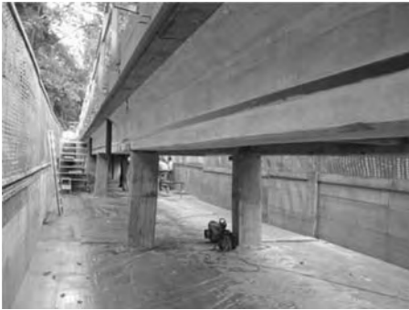
Figure 15. 30 m of prestressed CFRP plate.
