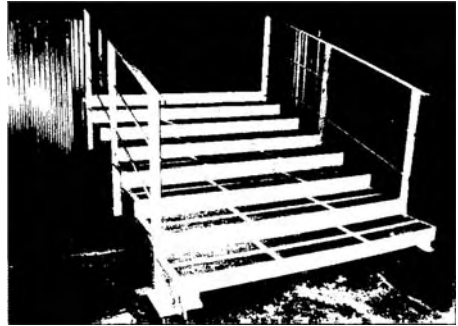
Figure 4. Footway for the railway bridge.
