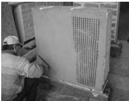
Figure 3. CMF installation.
