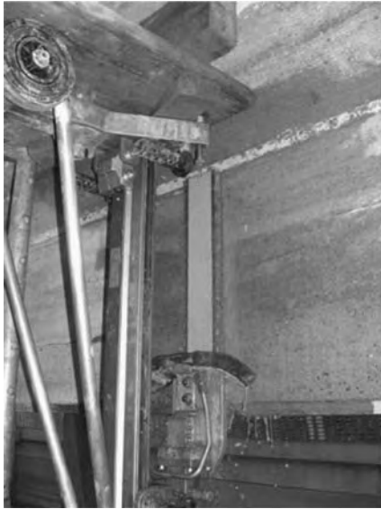
Figure 19. Cutting of the slits for shear reinforcements.
