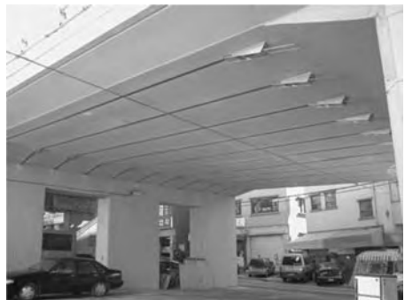
Figure 22. Applied Sika-StressHead tendons.
