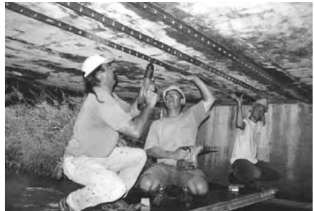
Figure 18. Workers installing FRP strips under bridge.
