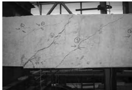
Figure 4. Crack angles (beam RC).
