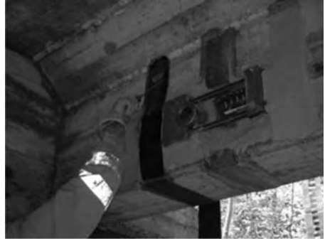
Figure 20. Impregnation of fabric (shear reinforcement).
