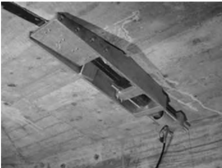
Figure 11. Special designed movable anchorage for redirection.
