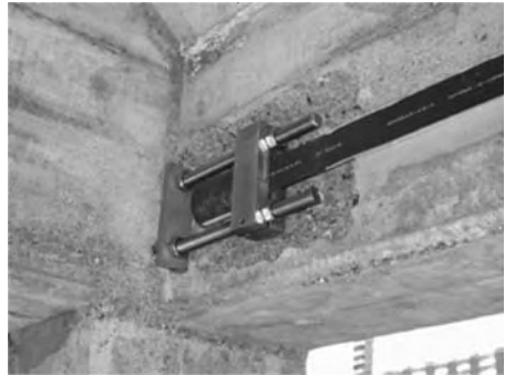
Figure 17. Connection through cross the girders.
