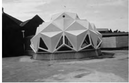
Figure 1. GFRP Composite Class Room System – 1974 conceived by Lancashire County Council UK.
