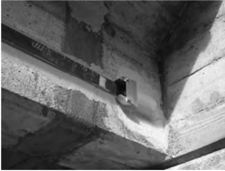
Figure 18. Anchorage on the fix side.
