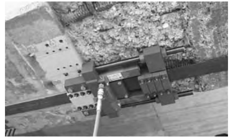
Figure 4. Jack with temporary & permanent anchors.
