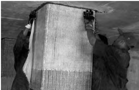
Figure 11. Properly engineered fabrics retain their strength and integrity after saturation and during installation (Jamaji et al. 2003).
