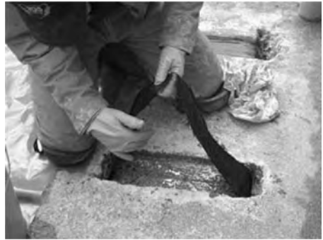
Figure 21. Fabric wrapped around the girders.
