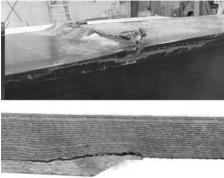
Figure 3. Failure of the compressive flange of a 36 inch DWB.
