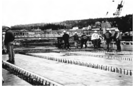
Figure 4. Casting of the steel free deck.
