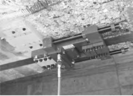
Figure 6. Prestressing in progress.
