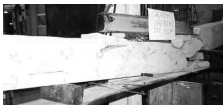
Figure 12. Cracking pattern and failure mode.
