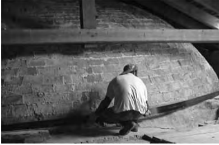
Figure 6. FRP strengthening of a masonry dome.
