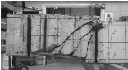
Figure 10. Shear failure of an FRP RC beam.
