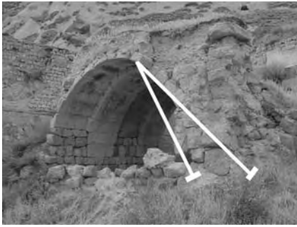
Figure 14. Supporting half arches.
