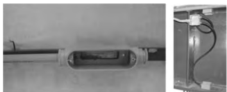
Figure 13. Rigid PVC conduit and junction boxes for externally installed gauges.
