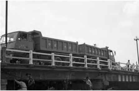
Figure 7. A bridge span strengthened for increase in live loads with a composite system being subjected to full service loads to evaluate its performance (Jamaji et al. 2003).
