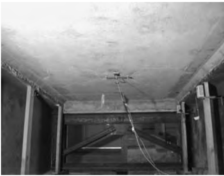
Figure 7(b). Bottom view of Segment A and instrumentation.
