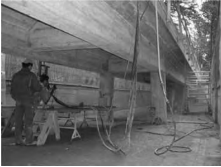
Figure 14. View under the bridge.
