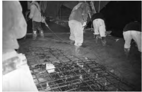
Figure 4. GFRP grid in Centre Street bridge deck.
