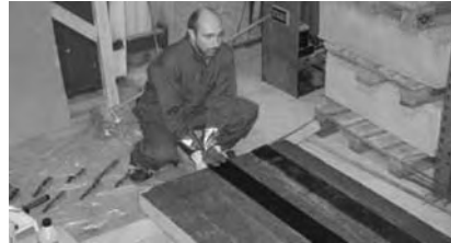
Figure 4. Bonding the CFRP fabric to slab No. 5.
