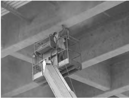
Figure 9. Surface preparation: grinding.
