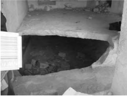
Figure 8. Room carved into rock with thin slabs.
