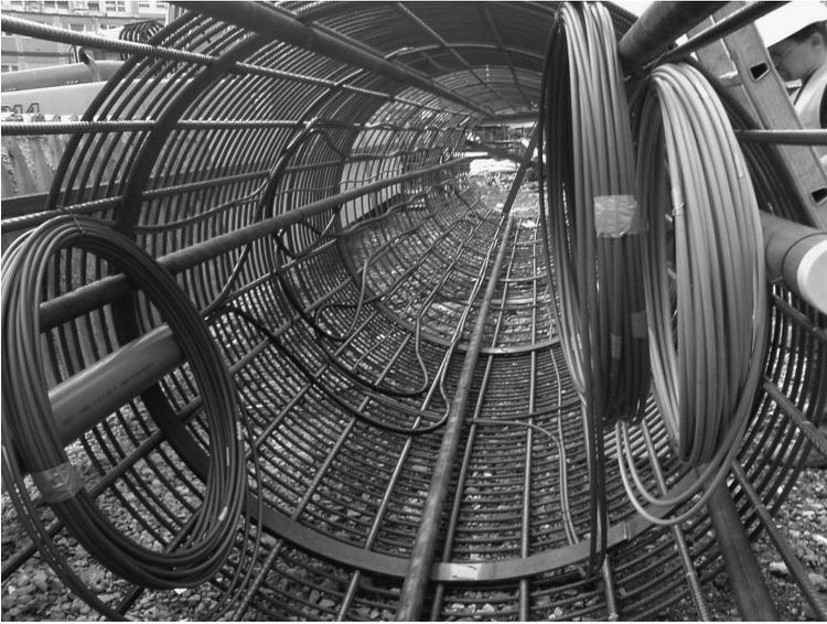
*Figure 7.6* Heat exchanger tubes and measuring cables at the reinforcement cage. (From Katzenbach, et al., *Geothermie*, Ernst & Sohn Verlag, Berlin, 171–220, 2011.)
