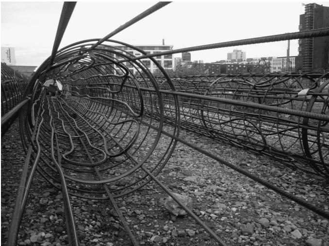
Figure 7.2 Heat exchanger tubes in a reinforcement cage. (From Katzenbach, et al., *Geothermie*, Ernst & Sohn Verlag, Berlin, 171–220, 2011.)
