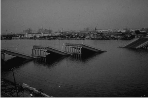
Figure 6.1 Failure of Showa Bridge during Niigata 1964 earthquake: Lateral spreading cause bridge spans to fall. (From Kramer, S.L., Geotechnical earthquake engineering. In: Prentice-Hall international series in civil engineering and engineering mechanics. Prentice-Hall, New Jersey, 1996.)
