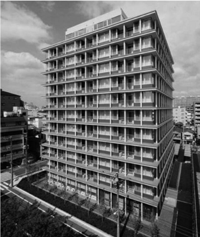
Figure 6.2 Twelve storey building survived after Tohoku Earthquake ( $M_w=9.0$ ) founded on CPRF. (From Yamashita et al., *Soils and Foundations*, 52, 1000–1015, 2012.)
