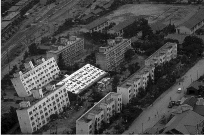
Figure 6.9 Tilting of apartment buildings at Kawagishi-Cho, Niigata during the 1964 Niigata Earthquake due to soil liquefaction. (From Kramer, S.L., *Geotechnical Earthquake Engineering*. Prentice-Hall, Upper Saddle River, NJ, 1996.)
