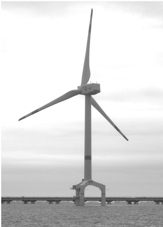
*Figure 7.25* Offshore wind turbines with Tripile foundation.
