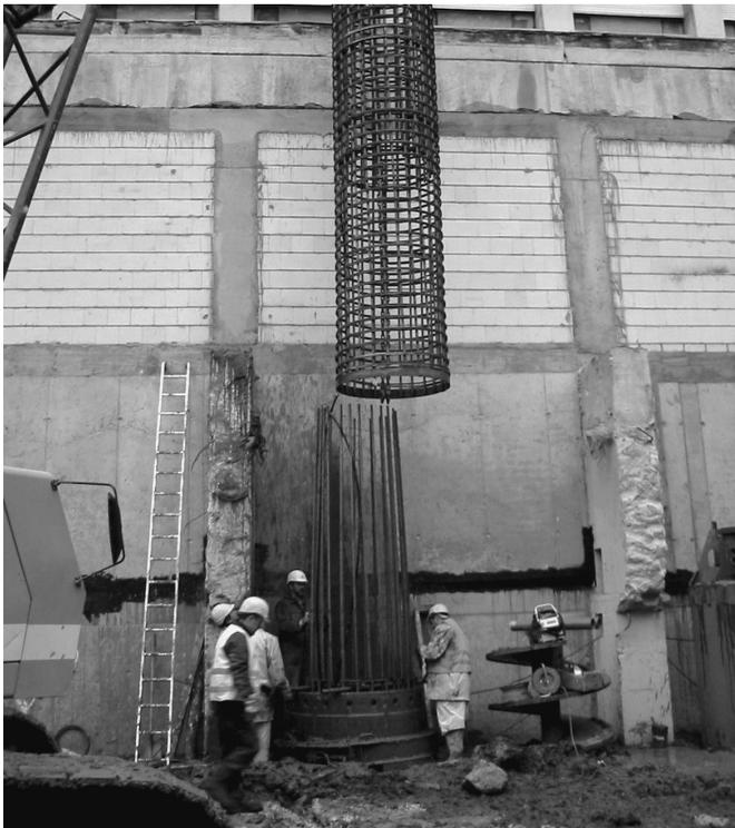
Figure 7.5 Reinforcement joint of an energy pile. (From Katzenbach, et al., Geothermie, Ernst & Sohn Verlag, Berlin, 171–220, 2011.)
