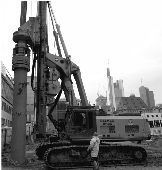
Figure 4.1 Construction of a bored pile in the inner city of Frankfurt am Main, Germany.
