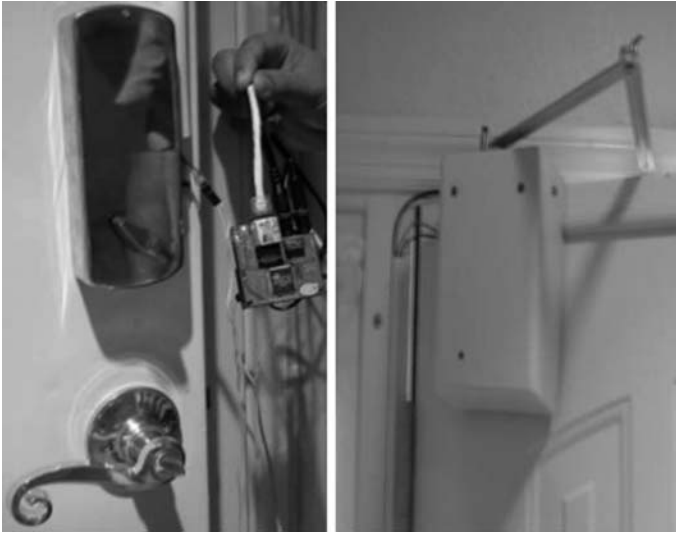
Figure 3. Entry assistant front door, with electronic deadbolt ( left ) and door opener ( right ).
