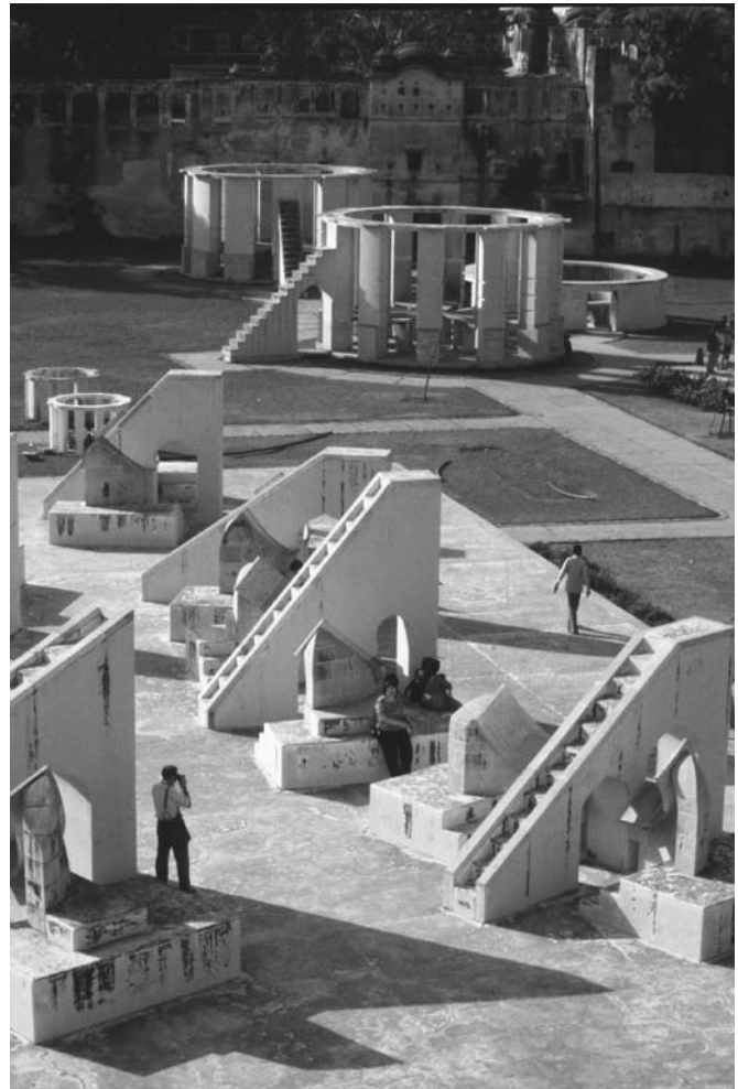
FIGURE 3.24. A selection of astronomical instruments at the Jaipur observatory of the Maharajah Jai Singh: Notice especially the Samrat Yantras that could be used to determine the moment of noon at each of several observatories around the world. The instruments would have been rotated to the hour angles equal to the longitude differences from the local observatory so that the different solar hour angles apply to the meridians of those places simultaneously. This is the equivalent of a wall of clocks registering the local times of different places in the world. Although the Jai Singh observatories were constructed in the 18th century, the instruments were built according to traditional specifications and thus represent classic Indian astronomical tradition. See Figure 9.10 for close-ups of the instruments at Jaipur and at the Maharajah's other observatory, the Jantar Mantar in Delhi. Photo by E.F. Milone.
