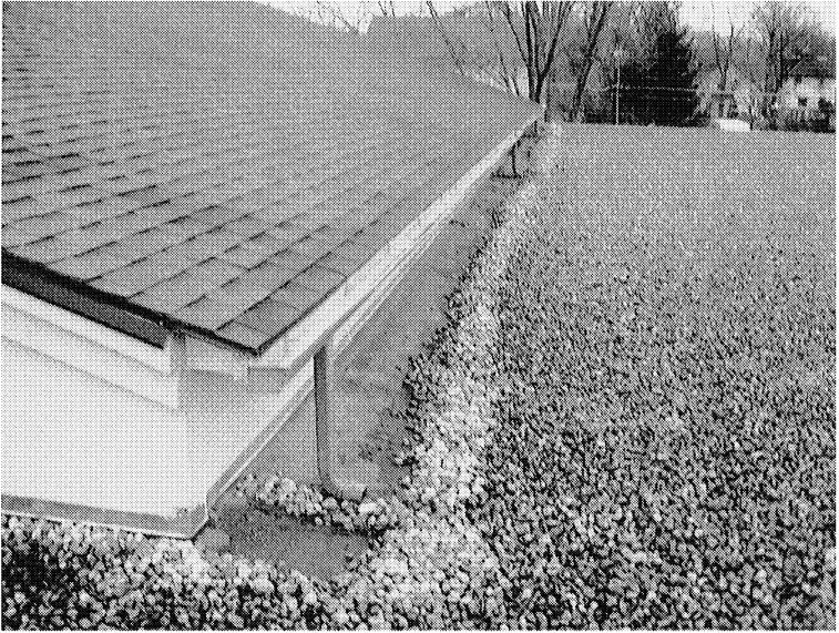
Figure 3. Overall view of sloped roof feature on library building.
