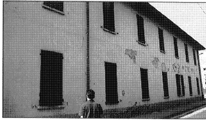
Fig. 3. Bovisio Masciago, BV1 buildings, Eastern elevation
