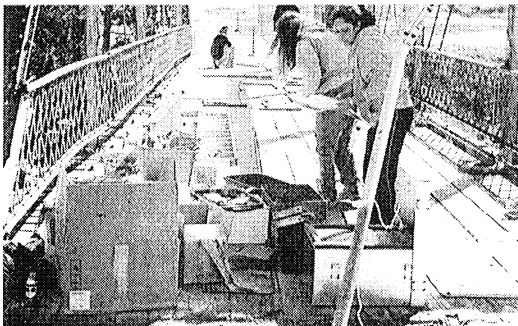
Figure 3. Blue River Test set-up in progress. The deck consists of longitudinal "running boards" on transverse timbers on steel stringers. The orthogonal criss-crossing of running boards and deck timbers creates a much more continuous deck than that at Fruita Bridge. The steel stringers bear on and are mechanically attached to the steel floor beams.
