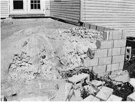
Figure 2. Fill flowed in between pieces of rubble.
