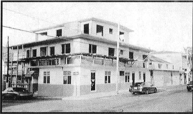
Figure 1. New second and third floor over an existing structure
