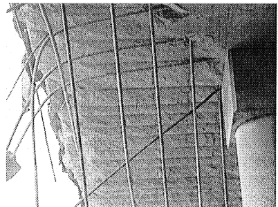
Fig 4. Roof slab steel stripped
