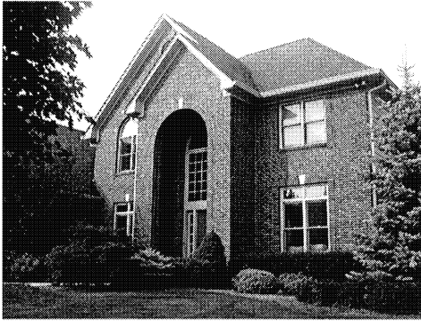
Fig. 1 East elevation of the house.
