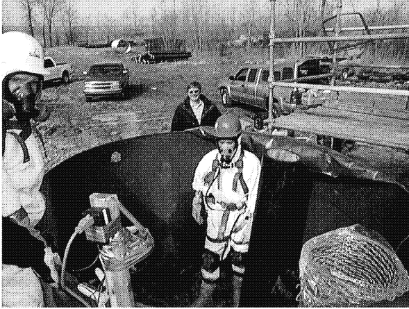
Figure 11. – Full scale mockup
