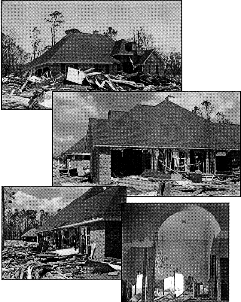
Figure 8: Series of photographs that documented damages to the house. Note that minimal damage was present to the roof covering, while severe damages were on the lower part of the structure. This was a good example of typical damages caused by the storm surge from
