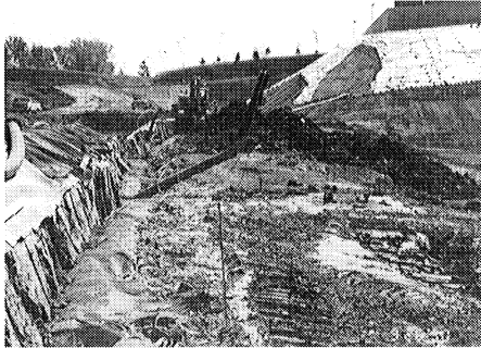
Figure 5. – A-North riser at subcell D tie-in
