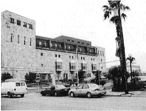
Figure 1. General view of Building A exterior.
