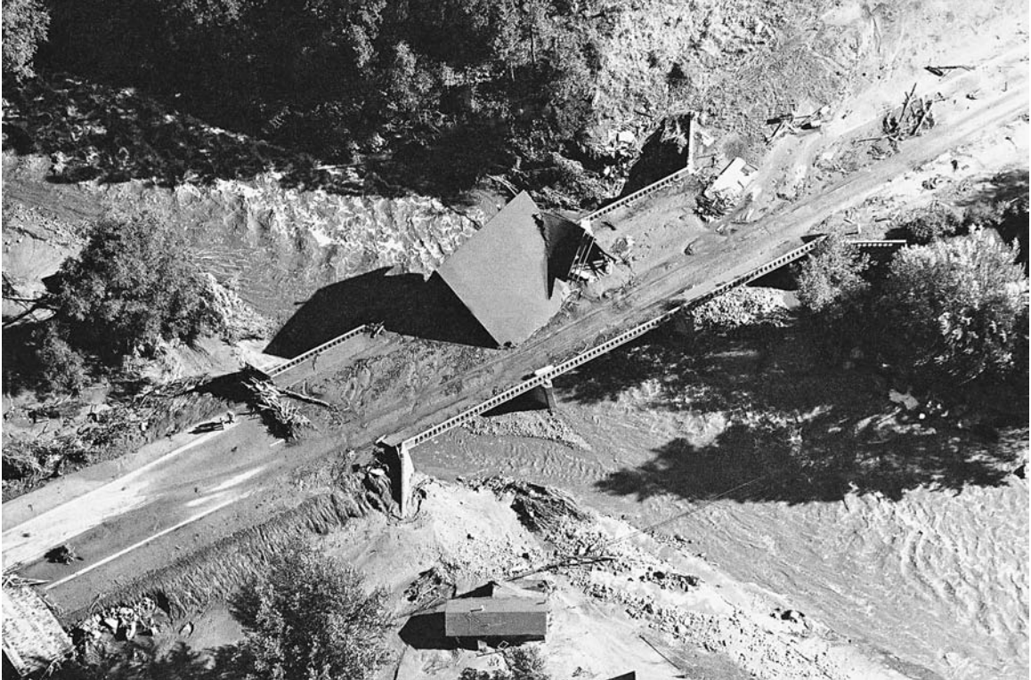
House roof on the bridge over the Big Thompson River near Estes Park, Colorado, August 3, 1976, after the Big Thompson Canyon flood (AP)
