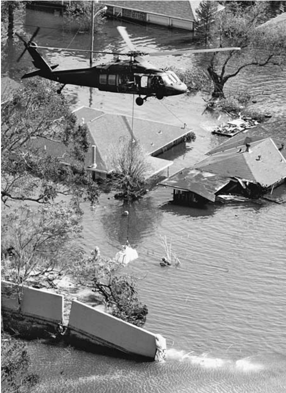
Loading sandbags onto an area where the levee has broken, New Orleans, September 9, 2005 (FEMA)
