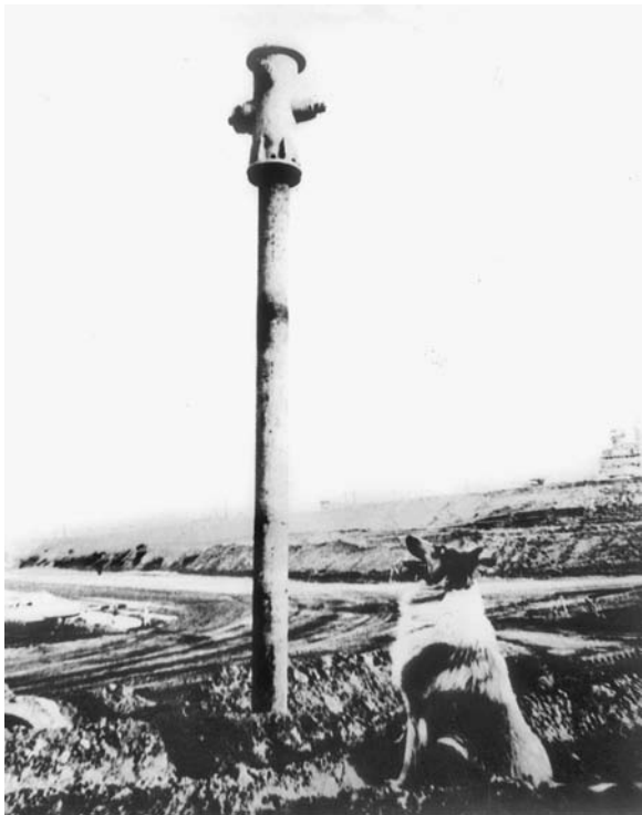
Dog and fire hydrant in Long Beach, California, 1950s, showing subsidence. The land surface used to be at the height of the base of the hydrant at the top of the long pipe, but extraction of fluids (water and oil) from beneath the surface caused the land surface to sink, placing the hydrant out of reach. (LBGO)
