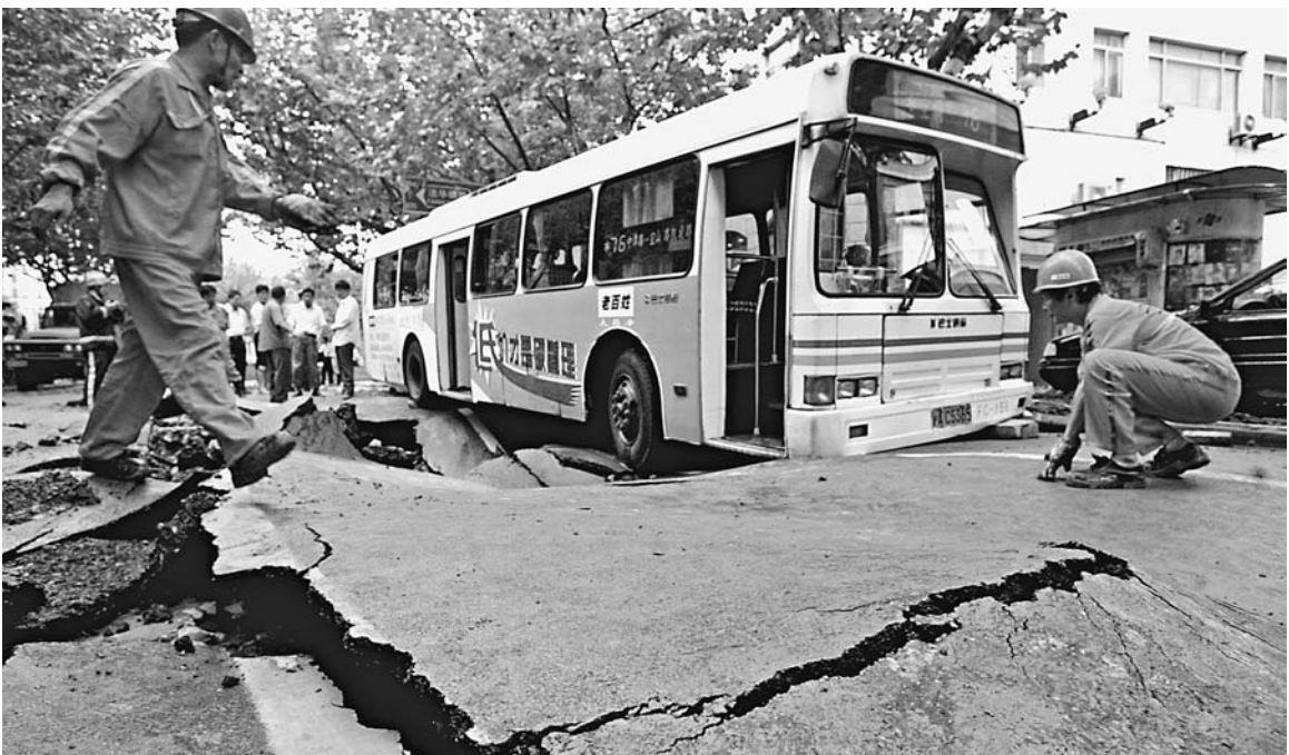
Two firefighters work beside a bus stuck in a hole in Shanghai, China, September 28, 2004. Water flooded a street and nearby houses after an underground water pipe exploded due to gradual ground subsidence. (AP)
