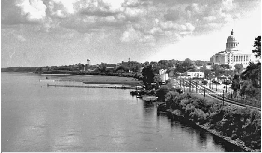
Wing dikes on the Missouri River, looking east at Jefferson City, Missouri, circa 1960. The wing dikes change the flow of the river and cause the river to deposit sand and mud, thereby making the channel become narrower. ( Missouri State Archives )
