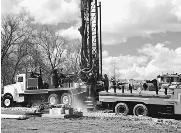
Drilling a groundwater well (Shutterstock)
