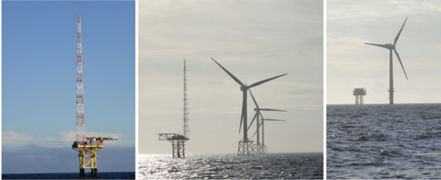
Fig. 9.3 Research platform Fino1 ( left and middle ) close to alpha ventus and relay/transformer station close to alpha ventus wind turbine AV12 ( right ), taken on 12/13 May 2013
