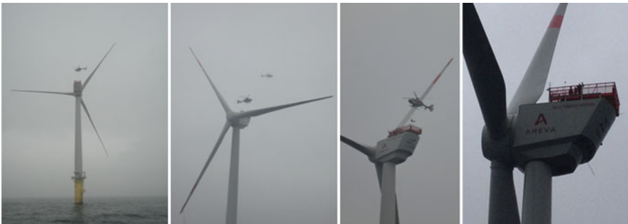
Fig. 9.4 Impressions of dimension of offshore wind turbine and nacelle. Helicopters bring people to offshore wind farm and let them down on a rope for maintenance work at wind turbine
