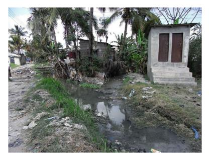
Fig. 6.7 Elevated toilets next to a clogged drain (Picture: Sigrun Kabisch 2012)
