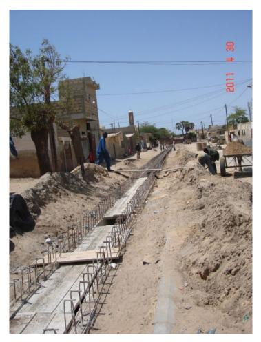
Fig. 9.5 Construction of new drains and sewerage in Diaminar (Picture: Trond Vedeld 2012)
