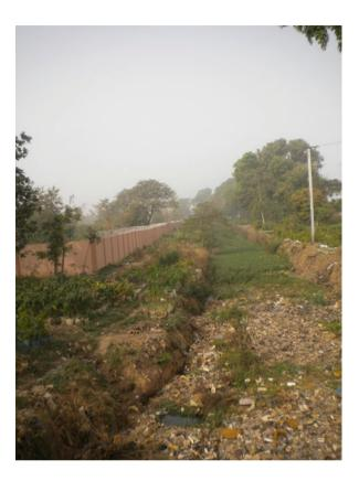
**Fig. 12.4** Sewer clogged by waste in the city of Ouagadougou (Picture: Hamidou Touré 2011)
