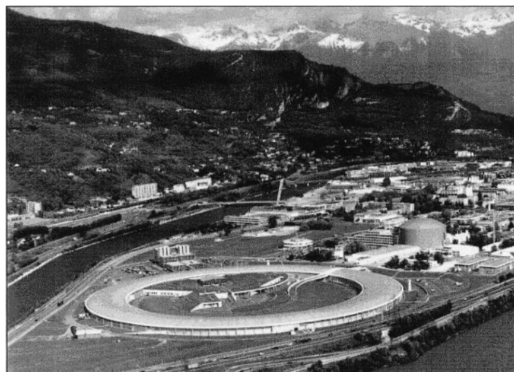
Fig. 13.3 The European Synchrotron Radiation Facility sited at Grenoble, France
