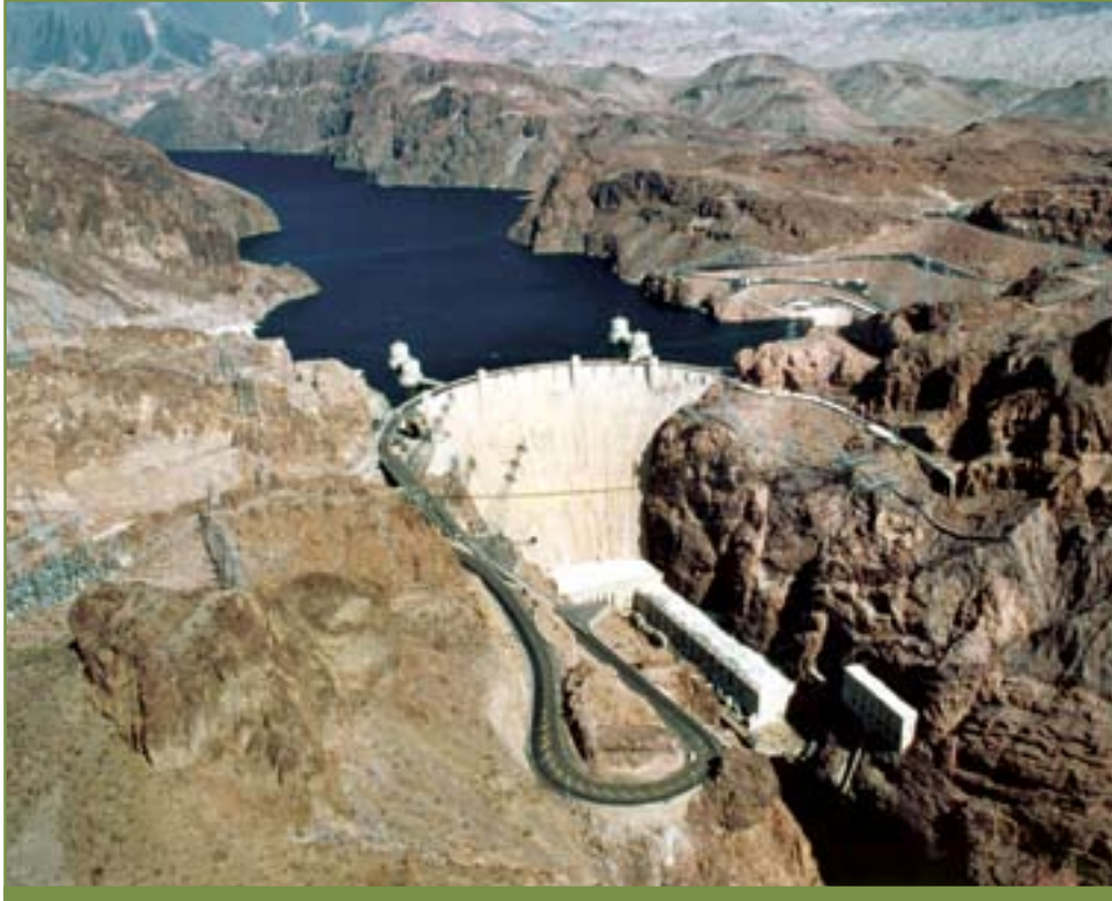
The Hoover Dam on the Arizona-Nevada border blocks the flow of the Colorado River to create Lake Mead. The dam was built to control floods, improve navigation, and regulate water flow, and the dam's power plant was built to generate electricity. ( U.S. Department of the Interior / United States Bureau of Reclamation )
