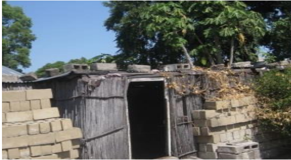
Figure 3. Various habitats searched for mosquito larva including clay pots, disused bottles, cement blocks placed by household owners to stop wind blowing roof tops, and cement blocks stored for future house construction.
