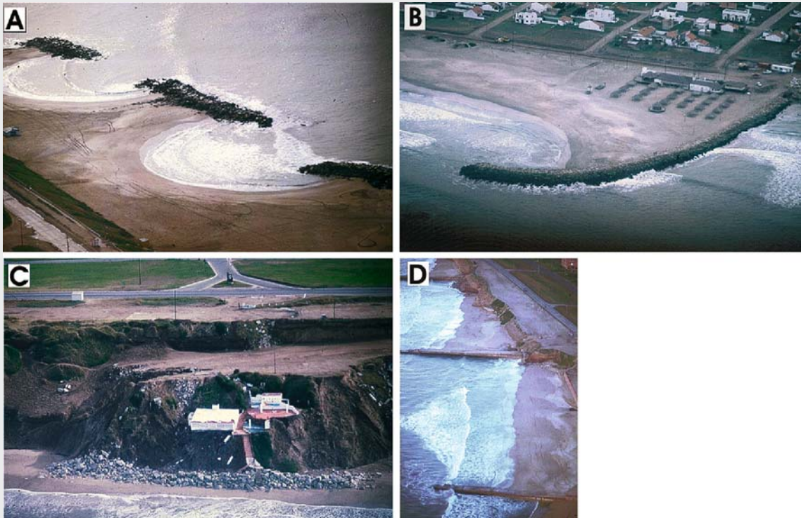
Fig. TB2.11.2. Some of the mechanisms of beach and cliff protection constructed along the Mar del Plata coast, Argentina
