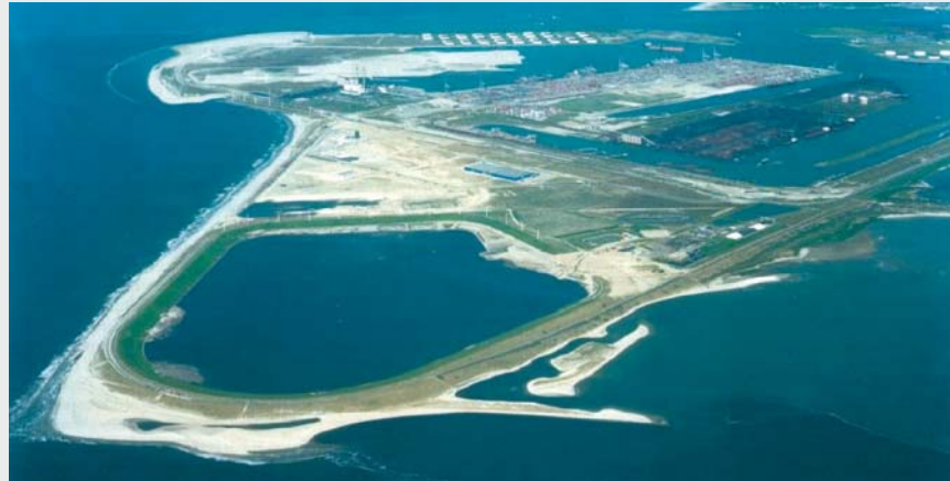
Fig. TB4.8.1. The Slufter (Rotterdam) – a confined disposal site for contaminated dredged material (from Grandrass and Salomons 2001)
