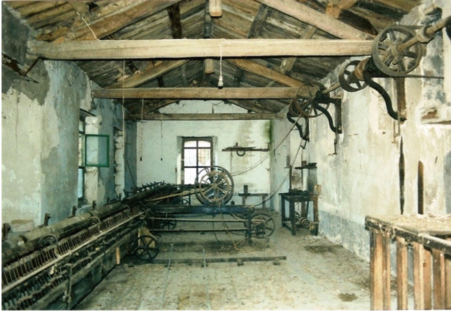
Fig. 17 Room and machinery as abandoned in the paper mill in Sant'Elia Fiumerapido
