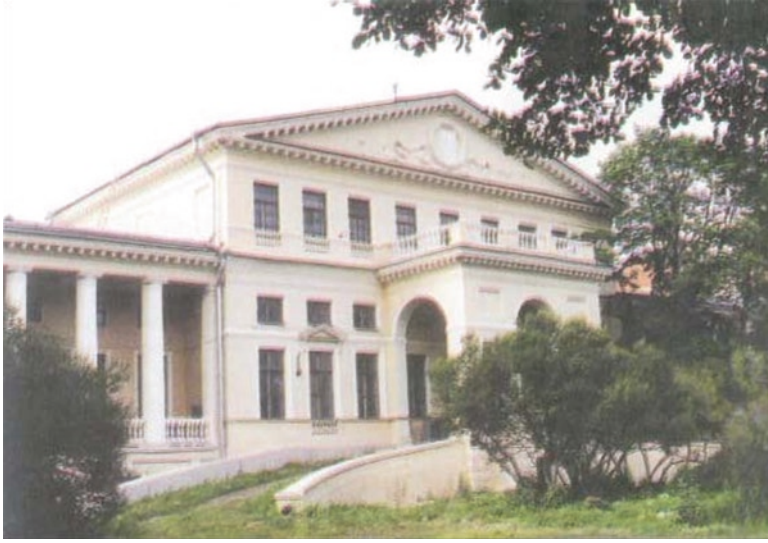
Fig. 11 First building of the Institute
