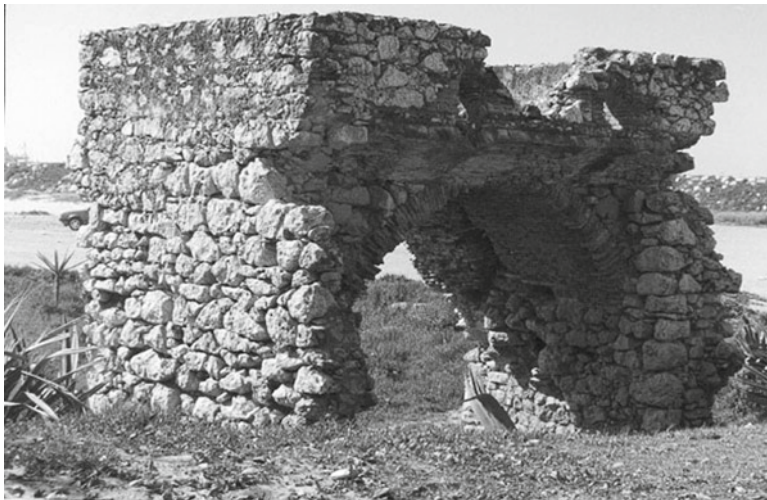
Fig. 4 Current remains. Centre building with the gathering pond
