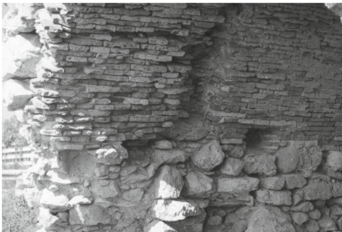
Fig. 5 Current remains. Symmetrical cavities
