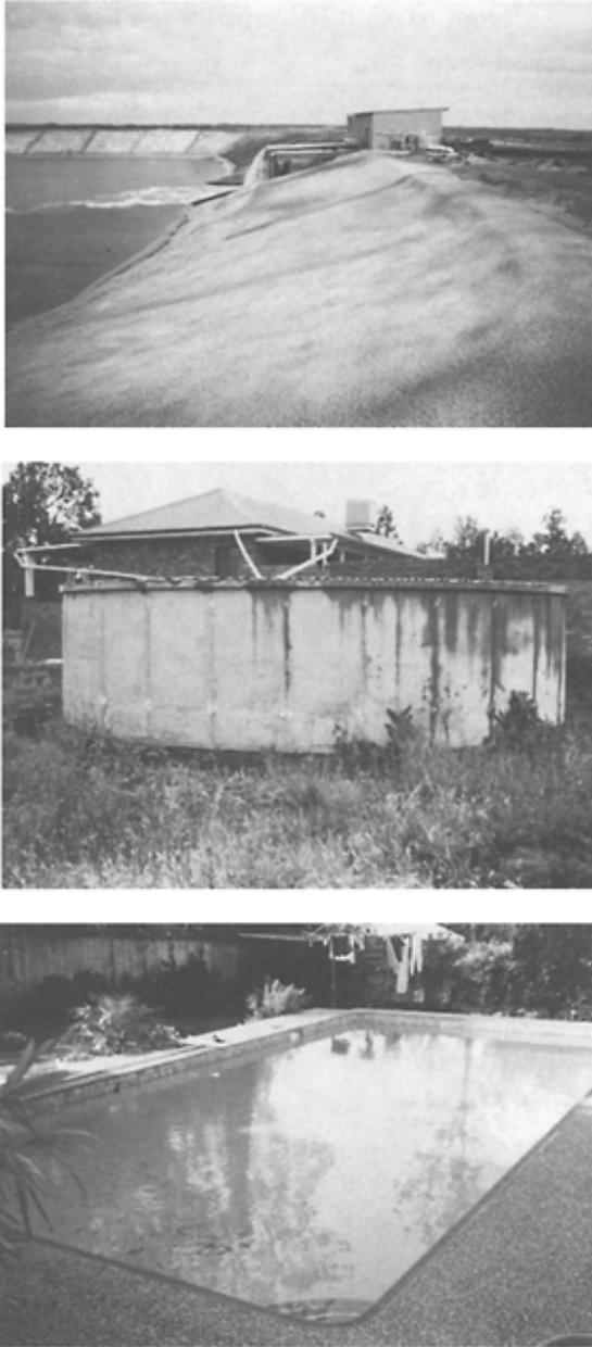
FIGURE 7.40 Australian use of SFRC in irrigation reservoirs (upper), water storage tanks (middle) and precast or cast-in-place swimming pools (lower) (Courtesy of BHP Reinforcing Products)
