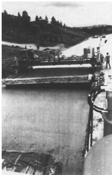
FIGURE 7.53 Bridge deck overlay placement on US 83 (upper) and full-depth highway construction (lower) in South Dakota using polyolefin fiber-reinforced concrete (Courtesy of V.Ramakrishnan)
