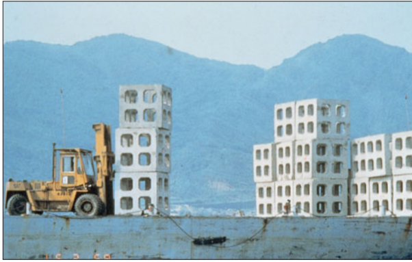
Figure 17.22 In Taiwan, high structural-strength coal-ash concrete has been developed to construct complex artificial reef units. These modules are about to be deployed from a barge. (Courtesy of Kwang-Tsao Shao, Institute of Zoology, Academia Sinica, Taipei, Taiwan, ROC.)
