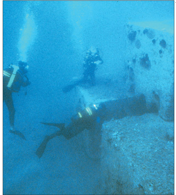
Figure 17.18 Illegal trawling of sensitive marine areas in Spain is being counteracted by these anti-trawling units. The steel railway lines protruding from the solid concrete blocks snag and destroy nets. (Courtesy of Technologia Ambiental, SA, Madrid, Spain.)
