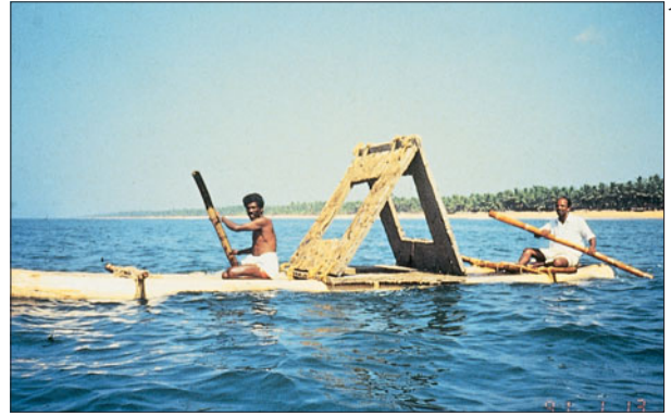
Figure 17.17 Smaller concrete slabs, cast in the sand on the beach, have been assembled into artificial reef units and are being paddled out to sea balanced on canoes made from three tree trunks lashed together (CWARP, Coal Waste Artificial Reef Program). (Courtesy of Steve Creech, Hampshire, England.)
