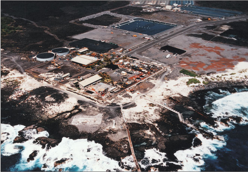
Figure 21.24 The Natural Energy Laboratory of Hawaii Authority's plant at Keahole Point, where there is an experimental 210 kW open-cycle OTEC plant. In an open-cycle plant, sea water is evaporated in near-vacuum conditions to create low-pressure steam, which drives a turbine; once the steam condenses the resulting water is discarded (compare with closed-cycle OTEC, as described in Figure 21.23 ). On the site, pipes can be seen for accessing cold ocean water (6°C from 600 m) and warm surface water (25–28°C); the large round tanks are ponds for growing fish and algae (kelp). (© Greg Vaughn, Natural Energy, Laboratory of Hawaii Authority, US.)
