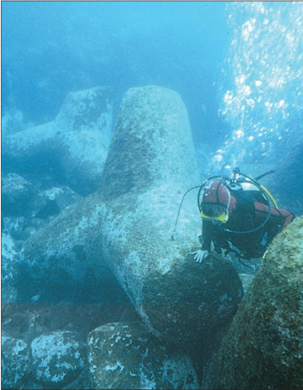
Figure 17.4 Coastal defence structures, such as these concrete tetrapods off Funchal, Madeira, provide new surfaces for colonisation by algae and encrusting animals.
