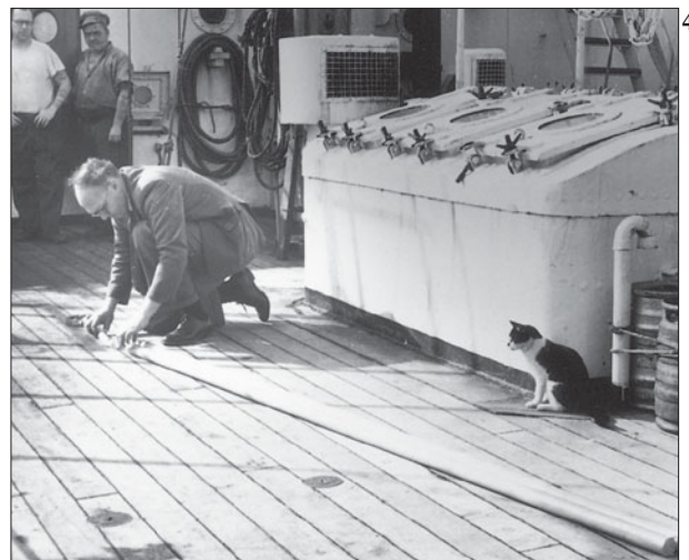
Figure 4.3 The invention of the neutrally buoyant Swallow float in the 1950s gave the first indication that deep currents in the interior of the ocean were not the then-predicted sluggish drift, but were dominated by energetic (a few centimetres per second) currents associated with meso-scale eddies. Here John Swallow is on board the RRS Discovery II preparing an early float (made from scaffold tube) and watched intently by the ship's cat and two of the crew.
