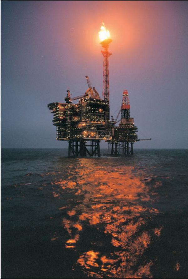
Figure 21.25 North Sea production platform complex in BP's Bruce gas field. (© British Petroleum.)
