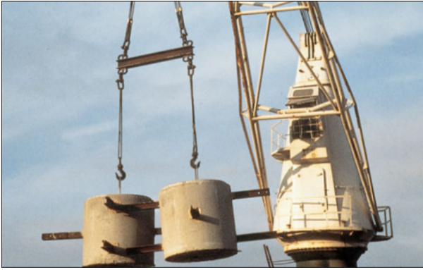
Figure 17.18 Illegal trawling of sensitive marine areas in Spain is being counteracted by these anti-trawling units. The steel railway lines protruding from the solid concrete blocks snag and destroy nets. (Courtesy of Technologia Ambiental, SA, Madrid, Spain.)
