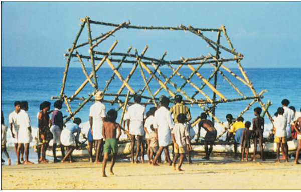
Figure 17.16 Artisan fishing communities in Kerala, Southern India, have used locally available materials, such as bamboo, to construct artificial reefs which are deployed on their village fishing grounds immediately offshore. (Courtesy of Steve Creech, Hampshire, England.)
