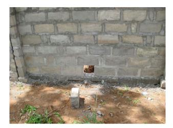
Fig. 4.20 The hole allows animals to pass through
