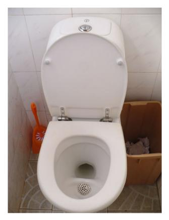
Fig. 4.37 Low-flush toilets with urine separator (5 instead of 10 L)
