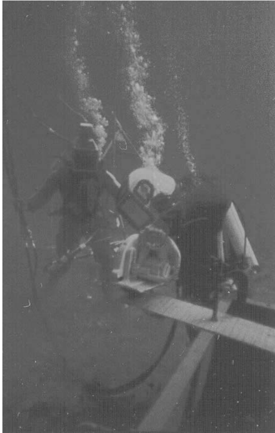
Figure 8.6 Surface-supplied divers using air-powered tools. (Courtesy of U.S. Navy.)
