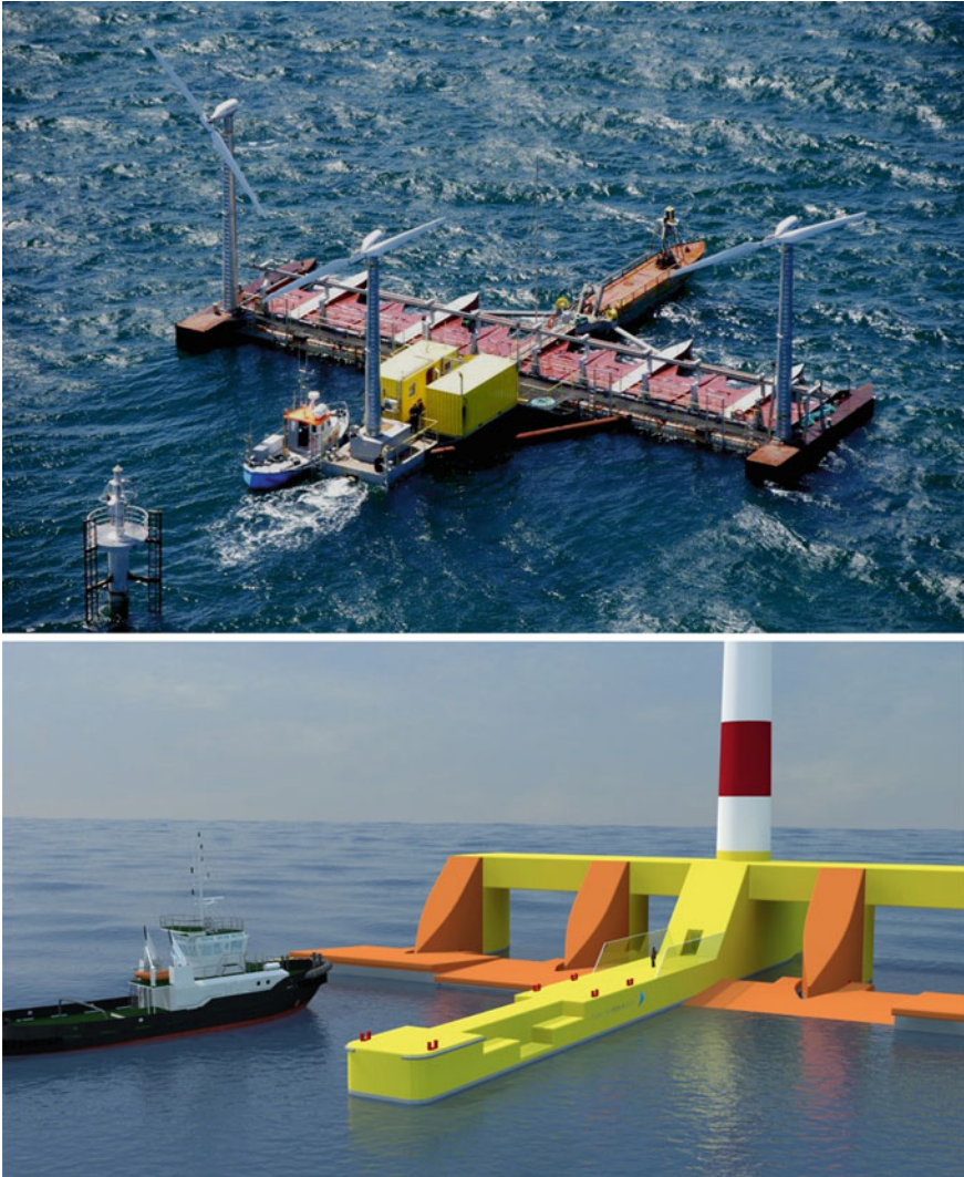
Fig. 22 Floating Power Plant, prototype deployed at Vindeby off-shore wind turbine farm, off the coast of Lolland in Denmark ( top ) and illustration of latest design ( bottom ). Courtesy of Floating Power Plant
