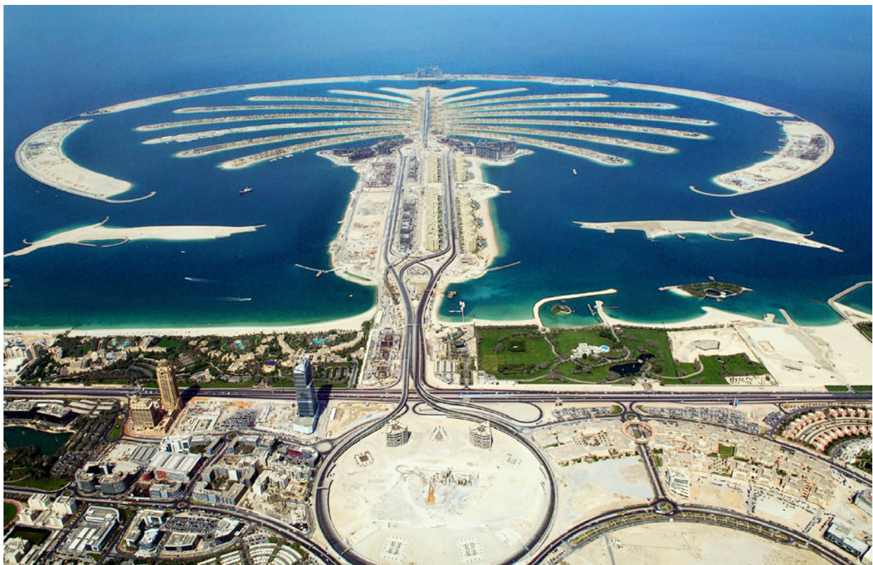
Fig. 8.44 a) Artificial islands (Palm Jumeirah) with about 5 km diameter at the Emirates coastline, 25^{\circ}07'N and 55^{\circ}05'E . (Photo credit: ©Google Earth 2010). b) Aerial photograph from Palm Jumeirah (Photo credit: ©Van Oord).
