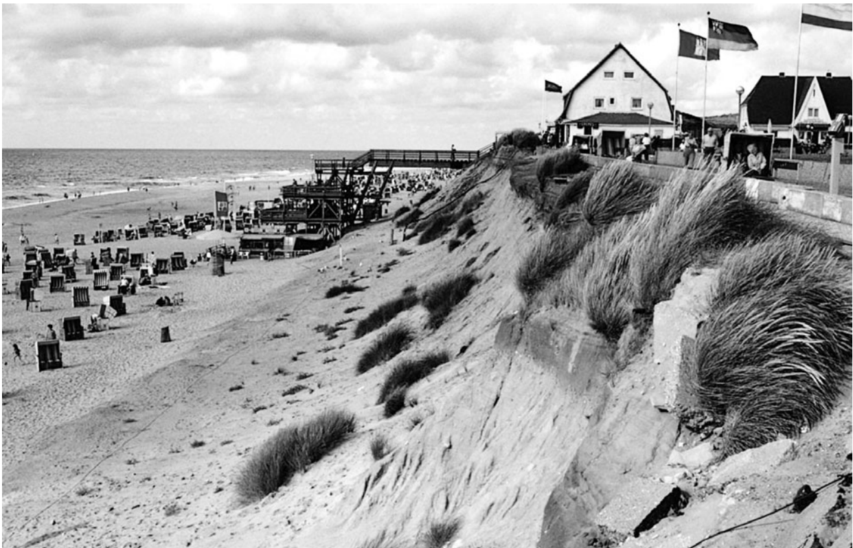
Fig. 4.51 Cliffs may also exist for a short time as quasi stable features in sand as in these mid-Holocene dunes with soil development and vegetation cover of Sylt Island, German North Sea coast. Many houses have been destroyed by rapid cliff retreat in these dunes during the last 200 years. (Photo credit: D. Kelletat).
