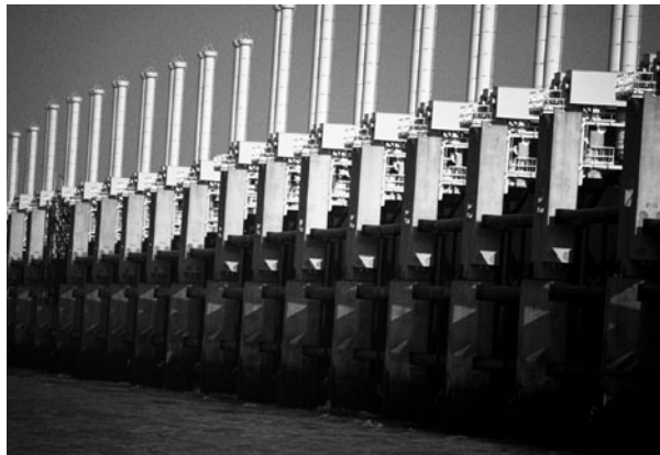
Fig. 8.11 a,b,c The Deltaplan protection works at the mouth of Scheldt river in the Netherlands protects the low-lying lands in the south western part of the Netherlands. The closing of the Eastern Scheldt Estuary was made a national priority after the catastrophic floods of February 1953. Originally, the Eastern Scheldt was to be a closed dam, but with increasing environmental awareness the Dutch started realising that only working with nature, and not against it, could ensure real safety. In 1975, the Dutch government proposed building an open barrier, instead of a simple closed dam, which could be closed during an emergency but would otherwise be open, preserving the ecology of the area. Now the Eastern Scheldt Dam has become quite an important tourist attraction, for visitors from all over the world. That makes sense, after all, the open barrier is one of the most impressive and beautiful maritime infrastructure feats ever conceived. The American Society of Civil Engineers (ASCE), a professional body founded in 1852, represents the members of the civil engineering profession around the world. This society made its own list of marvels of the civil engineering in an effort to recognize an actual equivalent to the Ancient Seven Wonders of the World. The Delta Work Plan of the Netherlands was listed a together with the Empire State Building, the Panama Canal, the Golden Gate Bridge or for example the Itaipu Dam. And the country has remained protected hitherto. (Photo credit: a) Google Earth 2010; b,c) istock).
