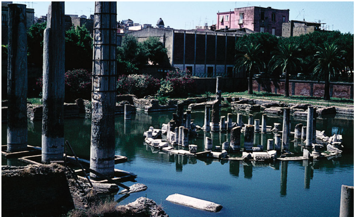
Fig. 1.57 The Serapeum, a temple from late Roman times near Pozzuoli in Italy, now located at groundwater level. The columns of the left part of the picture show dark rings with marine borings from a time when the sea inundated the temple. As it certainly was built on dry land, it provides evidence of several yo-yo-like earth movements during the last 2,000 years in this region. (Photo credit: D. Kelletat).
