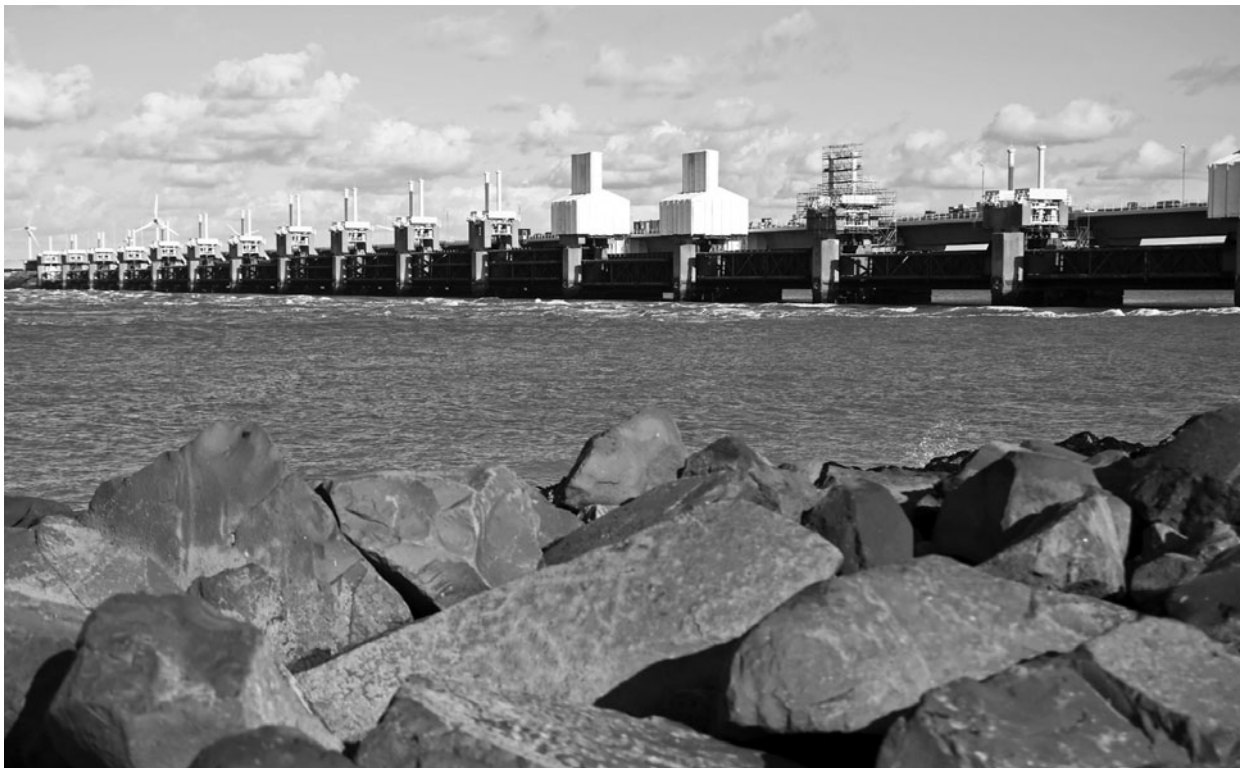
Fig. 8.11 a,b,c The Deltaplan protection works at the mouth of Scheldt river in the Netherlands protects the low-lying lands in the south western part of the Netherlands. The closing of the Eastern Scheldt Estuary was made a national priority after the catastrophic floods of February 1953. Originally, the Eastern Scheldt was to be a closed dam, but with increasing environmental awareness the Dutch started realising that only working with nature, and not against it, could ensure real safety. In 1975, the Dutch government proposed building an open barrier, instead of a simple closed dam, which could be closed during an emergency but would otherwise be open, preserving the ecology of the area. Now the Eastern Scheldt Dam has become quite an important tourist attraction, for visitors from all over the world. That makes sense, after all, the open barrier is one of the most impressive and beautiful maritime infrastructure feats ever conceived. The American Society of Civil Engineers (ASCE), a professional body founded in 1852, represents the members of the civil engineering profession around the world. This society made its own list of marvels of the civil engineering in an effort to recognize an actual equivalent to the Ancient Seven Wonders of the World. The Delta Work Plan of the Netherlands was listed a together with the Empire State Building, the Panama Canal, the Golden Gate Bridge or for example the Itaipu Dam. And the country has remained protected hitherto. (Photo credit: a) Google Earth 2010; b,c) istock).
