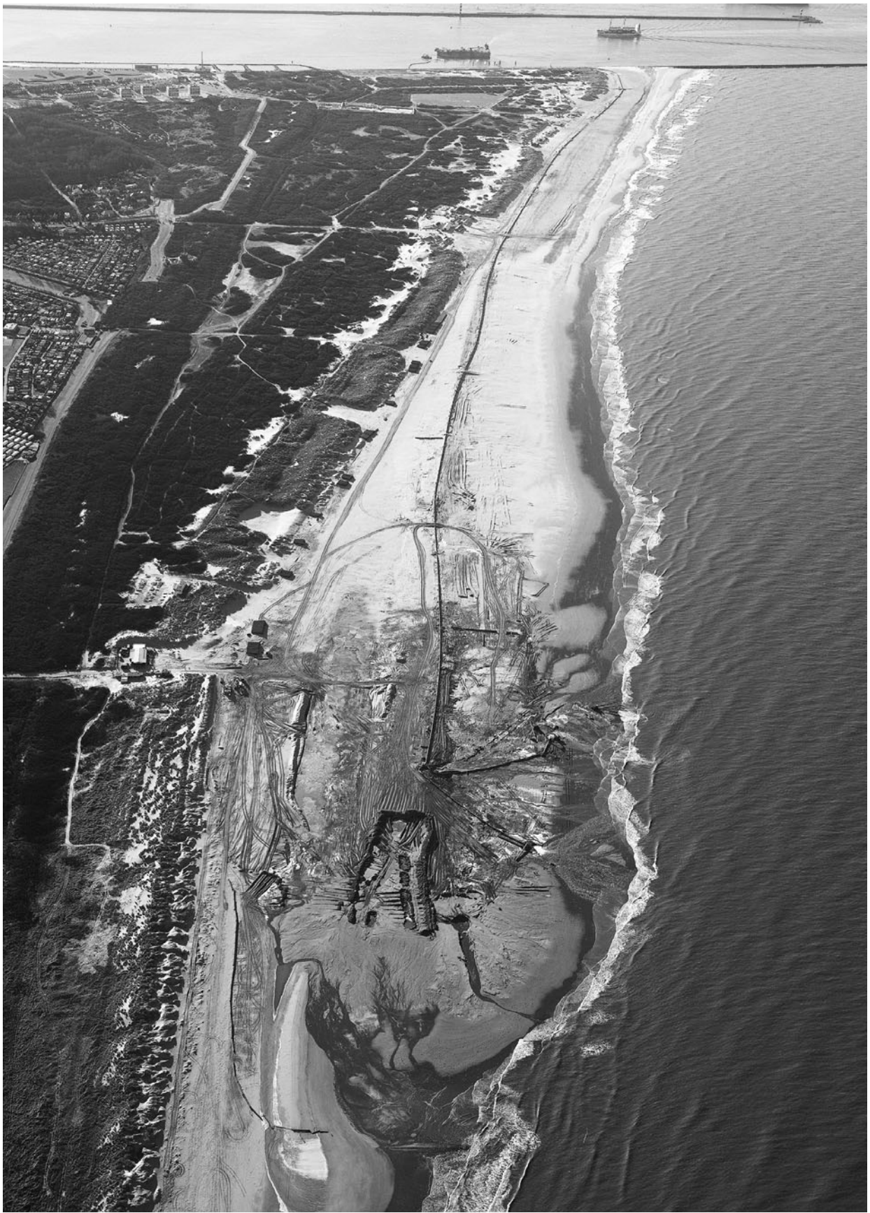
Fig. 8.41 a Artificial beach nourishment along the Delflandse coast (Photo credit: ©Van Oord)
