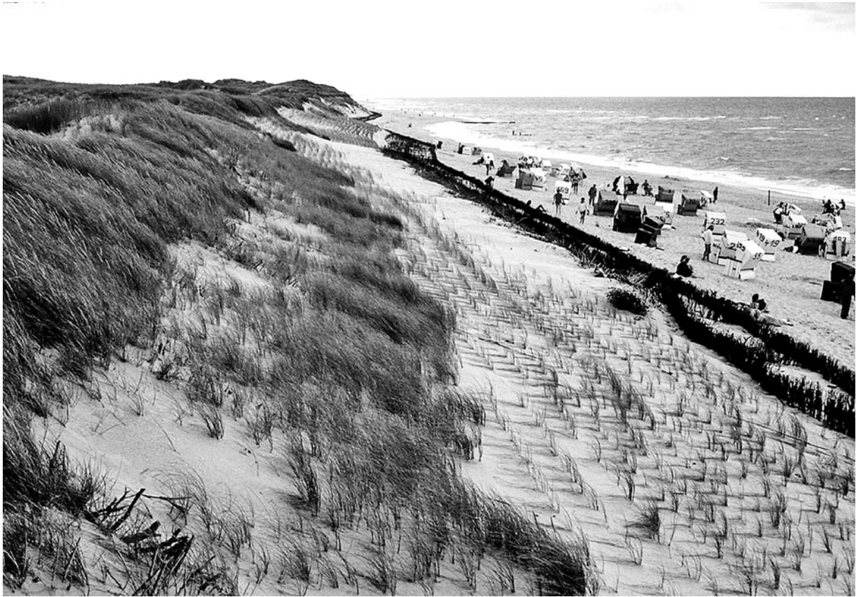
Fig. 8.40 A strategy to stabilize dune cliffs with vegetation to catch and retain sediments along the outer coasts of the barrier islands of the German North Sea coast. (Photo credit: D. Kelletat).
