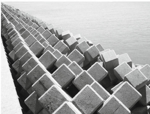
Fig. 8.36 Concrete tetrapods as storm wave protection. (Photo credit: Istockphoto LP).
