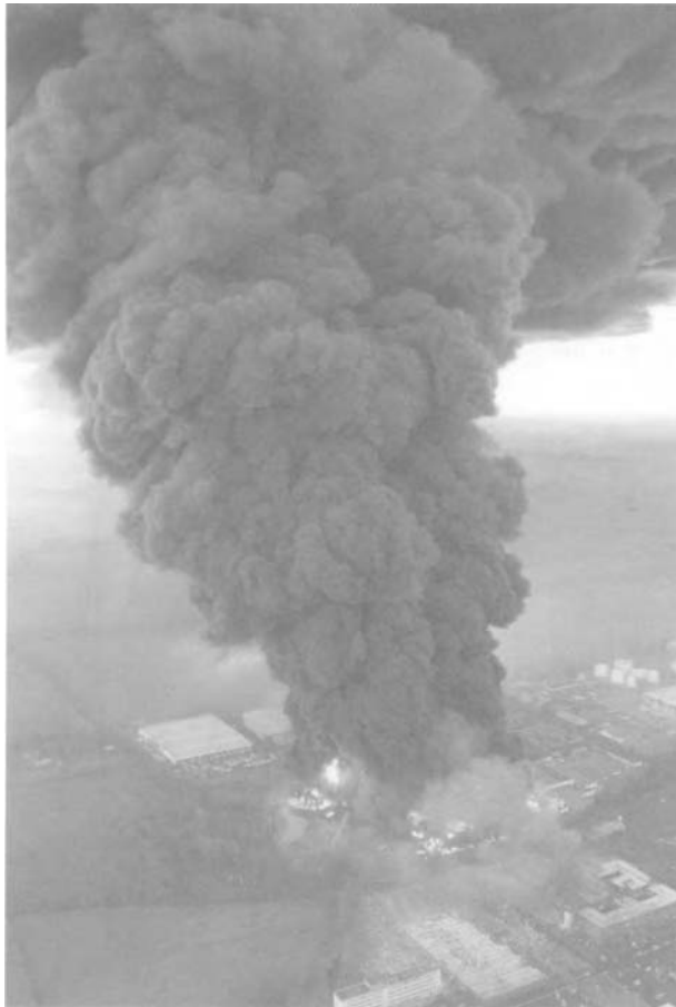
Fig. 8.6 Buncefield fuel depot fire (Photo courtesy of AP Photo/Hertfordshire Police).
