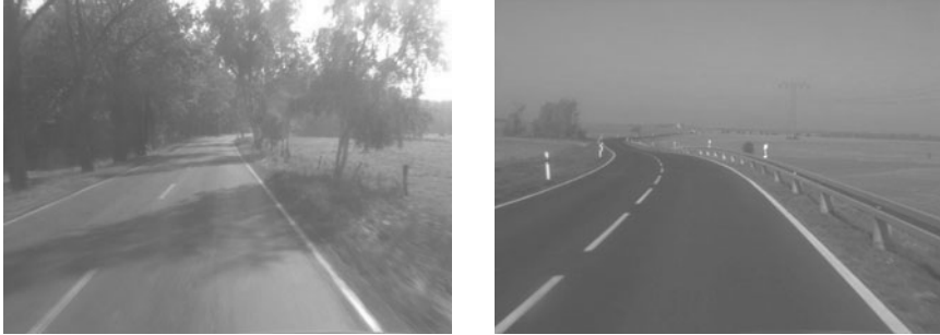
Figure 38. Pictures of sections A20 (left) and A44 (right). The latter also shows the preceding curve in opposite direction to the main curve (picture source: RoadView).
