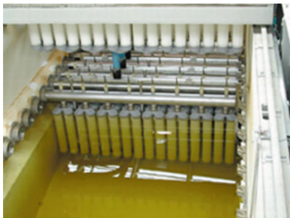
Fig. 3.14 Submerged hollow fiber modules of MEMCOR. The world’s largest CMF-S pure water treatment facility with the capacity of 126,000 m 3 /day is in operation in Bendigo, Victoria, AustraliaMF. Reprinted with the permission from Ref. [28]. Copyright 2016 XXXX
