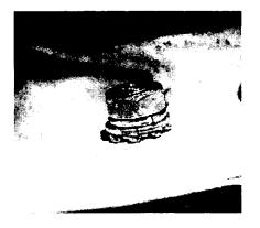
**Figure 7.5** A reliable Safety Earth Ground – note that a coarse 'Star' washer is used to cut through a paint finish. Constant pressure is applied onto the grounding hardware by a spring washer
