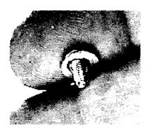
**Plate 17** This Safety Earth Ground fixing is a 'ring type' – which is good – but the fixing screw is much too small to provide a reliable connection
