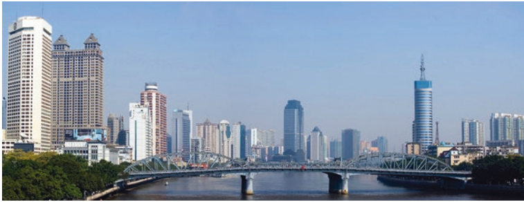
Fig. 6.1 The Pearl River Bridge, circa 2010
