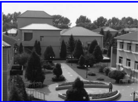
Figure 4. Good combination of building group and landscape.
