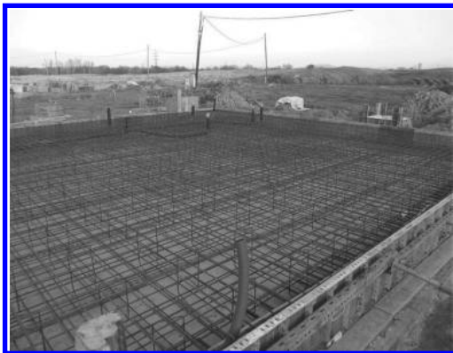
Figure 6. Reinforcement of concrete foundation slab.
