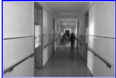
Figure 2. Continuous safety handrail in corridor.
