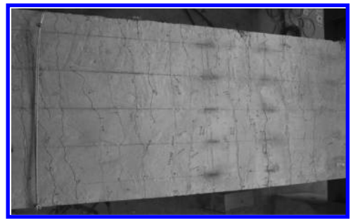
Figure 11. Concrete flange plate crack distribution.
