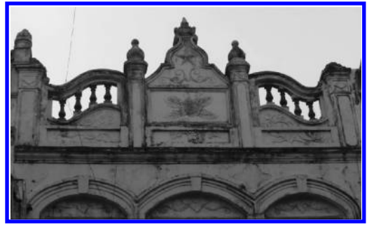
Figure 3. The pediments of a arcade building with ash plastic and prefabricated decorative components on it.
