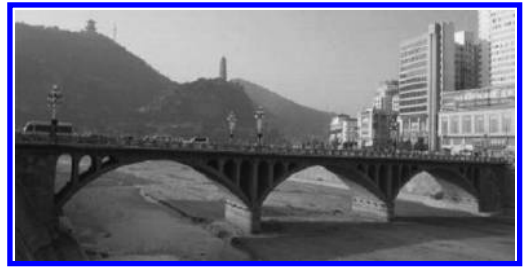
Figure 2. The site actual picture of Yanhe River Bridge.
