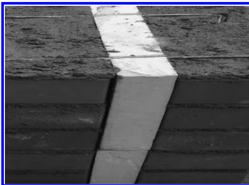
Figure 2. Tie and PCM between two leaves wall.
