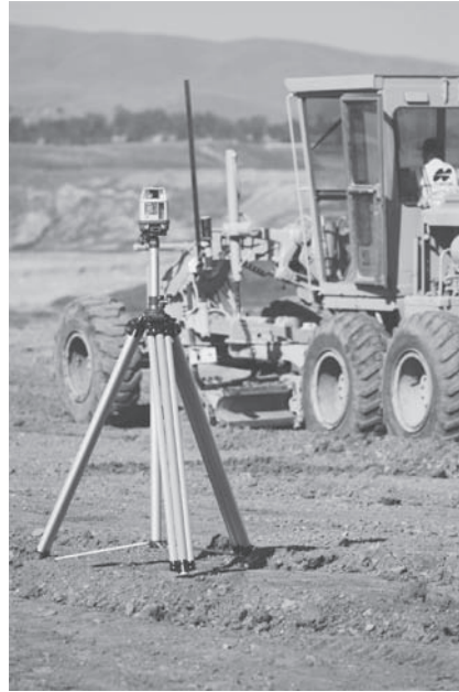
Figure 23.2 Rotating laser providing finished grades to machine control system in grader. (Courtesy Topcon Positioning Systems.)
