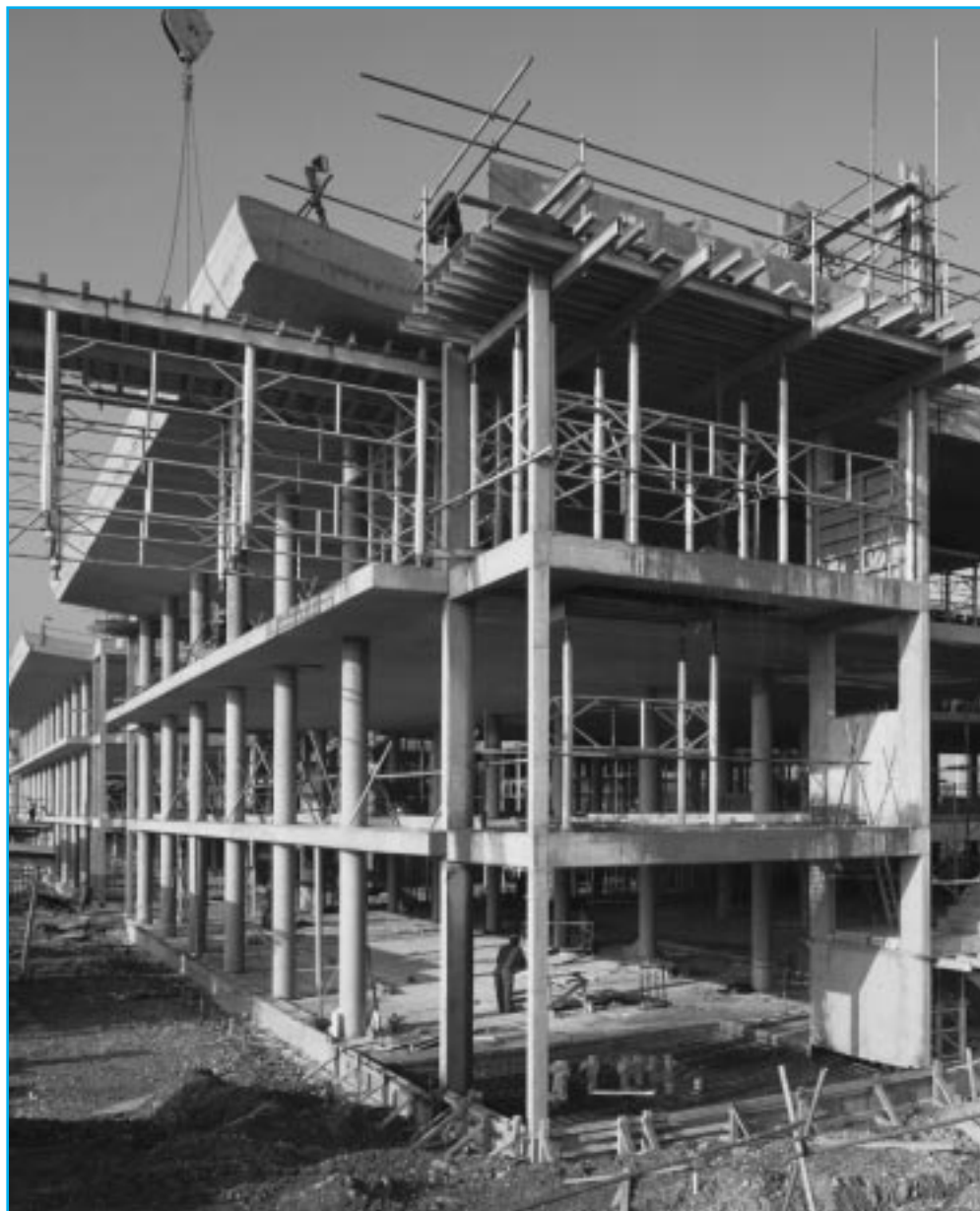
Combined Operations Centre, Heathrow, under construction
