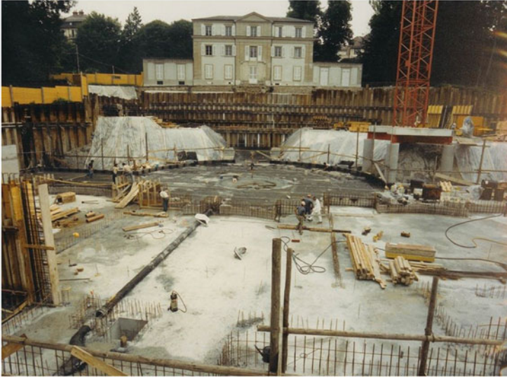
Fig. 4.3 IMEDE campus construction (1988). Source: Copyright@2014 IMD
