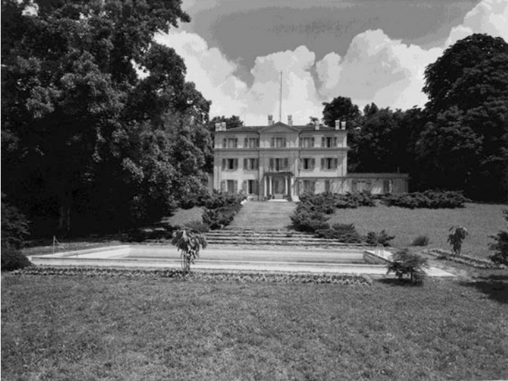
Fig. 2.1 The Bellerive Property 1950 (approx.). Source: Copyright© 2014 IMD
