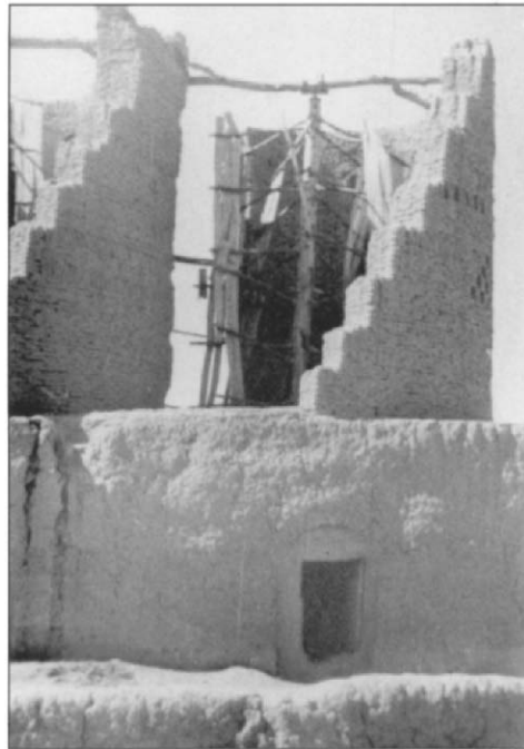
Plate 4 Afghan windmills (IslamQala) viewed from the south. Notice curved and stepped walls (Richard Hewer, 1971).
