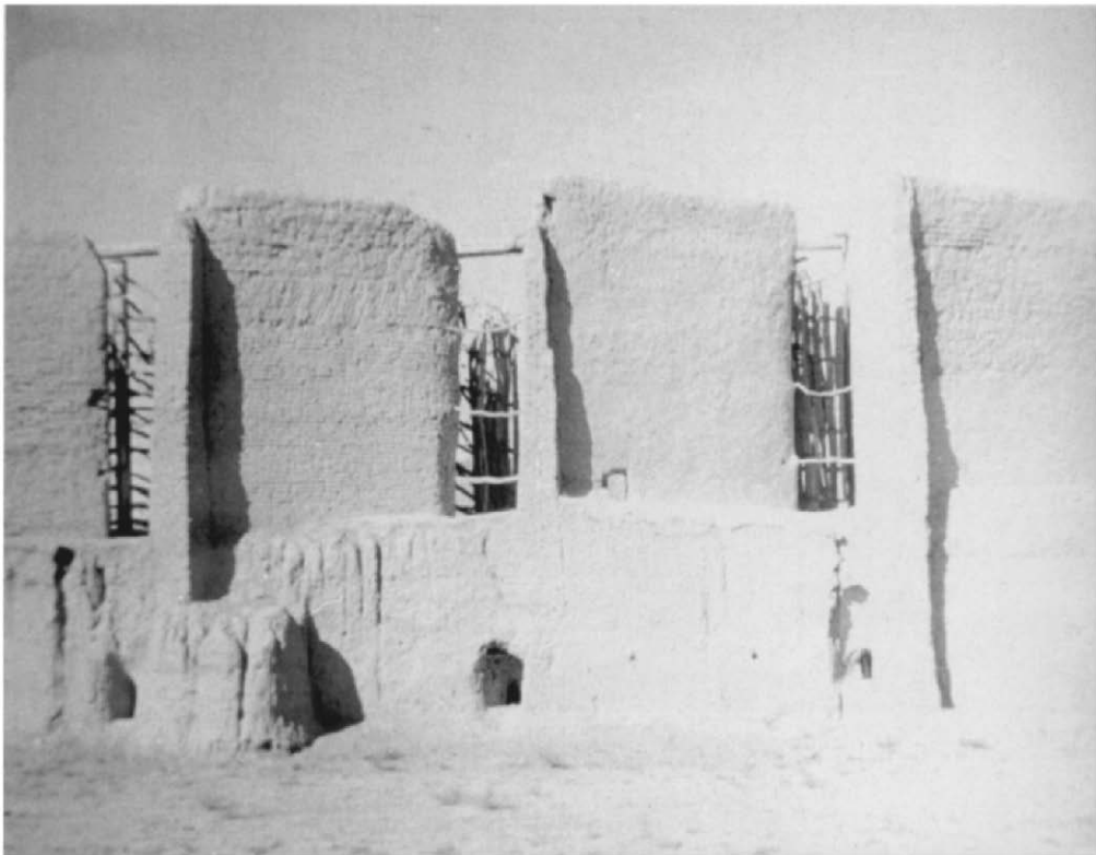
Plate 2 Windmills at Khaf: viewed from the north. Notice the winnowing slits near the ground below each of the main wind slits.
