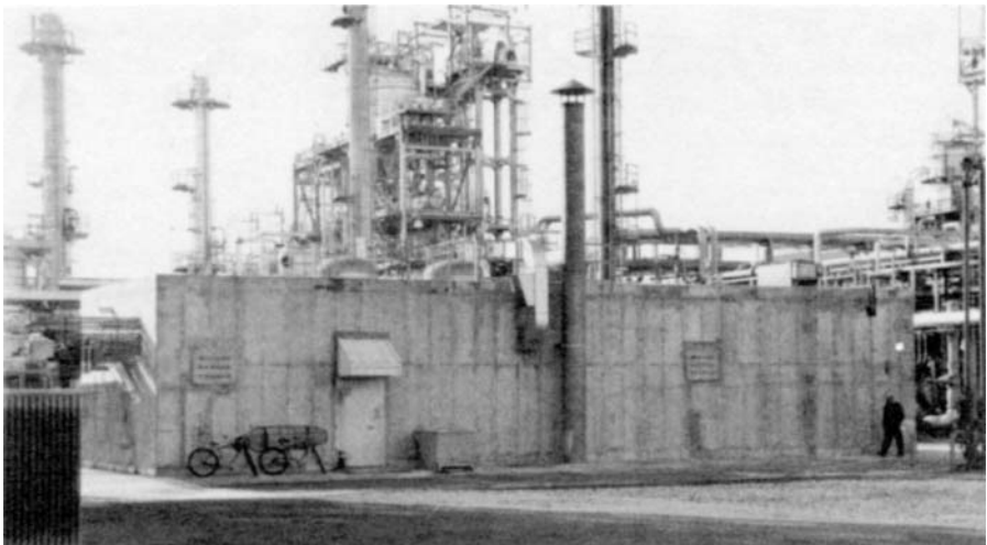
PHOTO 8. Reinforced Control Room Building in Operating Area'
