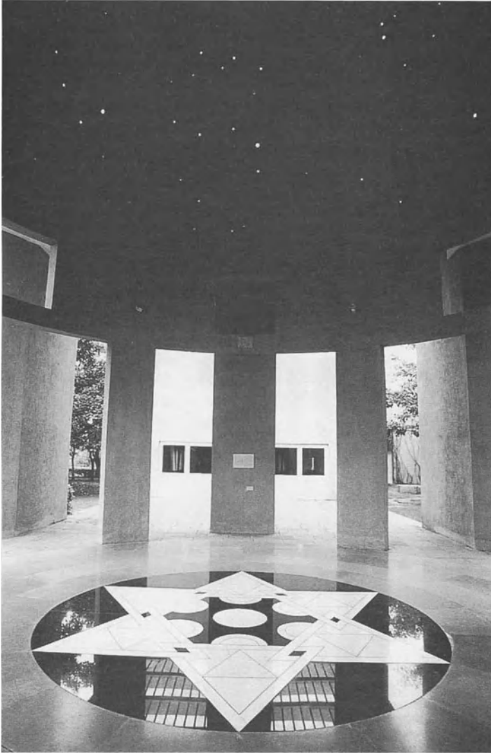
Figure 2. The dome which borders the central courtyard at IUCAA has tiny holes right through it. The holes are of varying sizes admitting day light through them so that persons standing underneath the dome see the star studded sky during the day time. The star distribution is arranged to match that prevails at 8:30 pm on IUCAA's Foundation Day, December 29, 1988.
