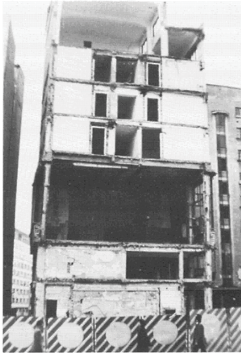
Figure 11.40 Collapse of a building in Bucharest during the 1977 earthquake. The building had been repaired after the 1940 earthquake.
