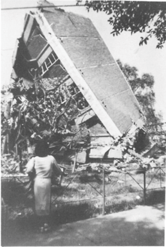
Figure 11.34 Torsional collapse of a building in Mexico City, 1985.
