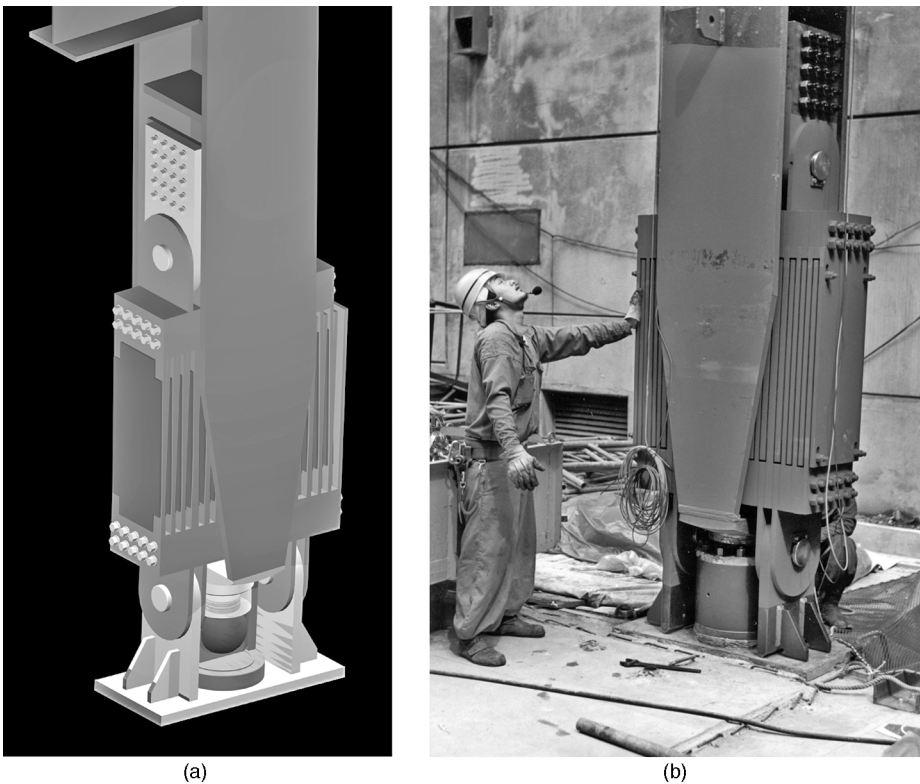
Fig. 13.5 Building incorporating 'stepping' columns, La Maison Hermes , Tokyo: (a) schematic; and (b) column during installation (see Lang et al. 2001)
