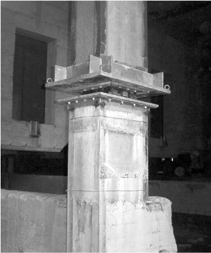
Fig. 13.4 Retrofitting of an existing reinforced concrete building. Multifunction centre, Napoli, Italy
