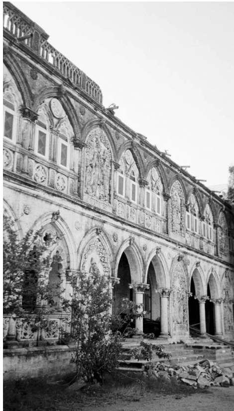
Fig. 10.1 Increase in seismic damage with height in a stone masonry building, Gujarat, India, 2001
