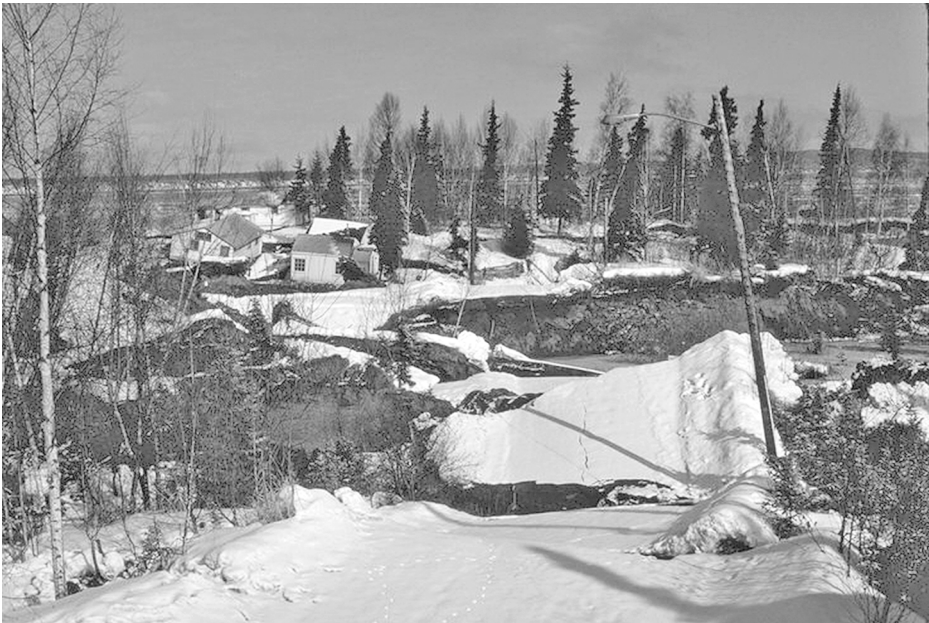
Fig. 4.6 Liquefaction-induced lateral spreading, Alaska 1964, showing destruction of a road and housing
