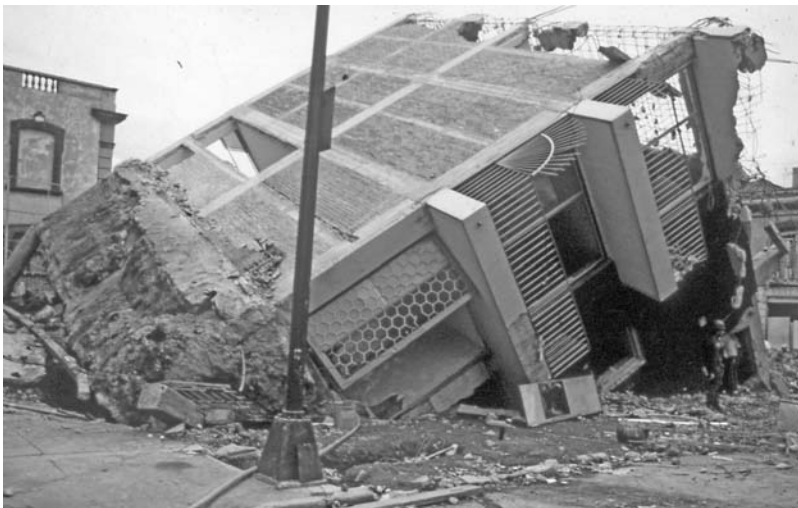
Fig. 7.2 Bearing capacity failure in Mexico City, 1985
