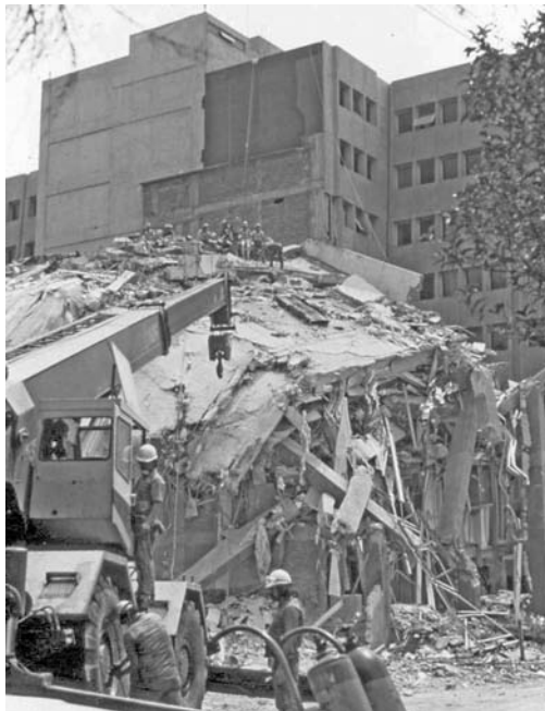
Fig. 1.3 Total collapse of a multi-storey reinforced concrete structure in Mexico City, 1985
