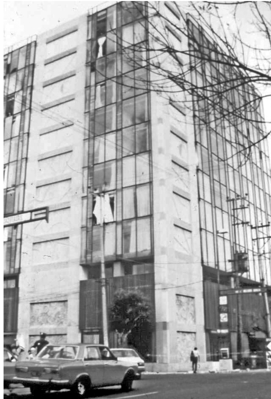
Fig. 14.1 Building in Mexico City after the 1985 earthquake. The building had previously been strengthened by the addition of external shear walls
