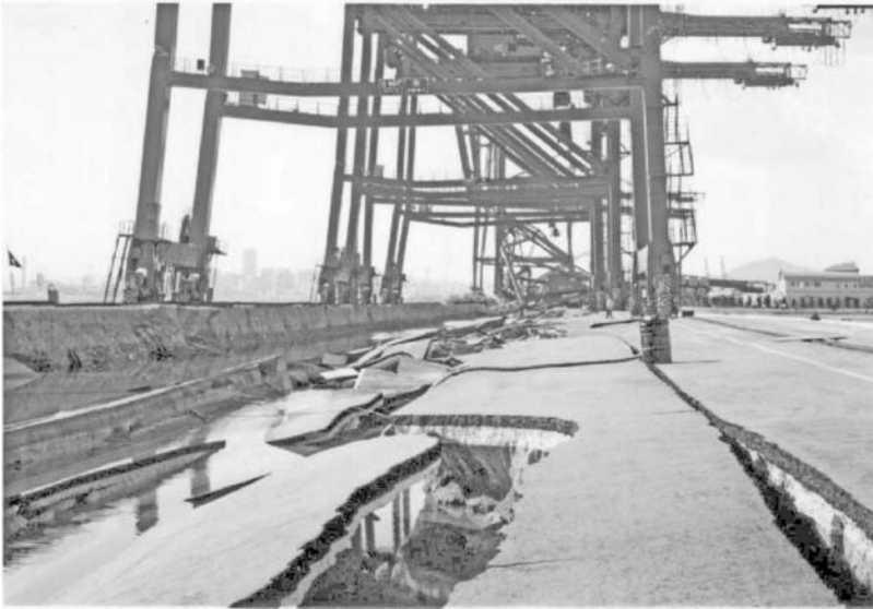
Fig. 1.1 Damage in the port of Kobe, Japan, 1995
