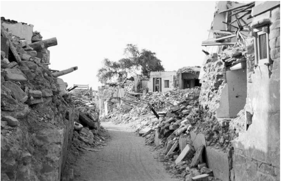
Fig. 1.9 Total collapse of weak random rubble masonry housing in Gujarat, India, 2001
