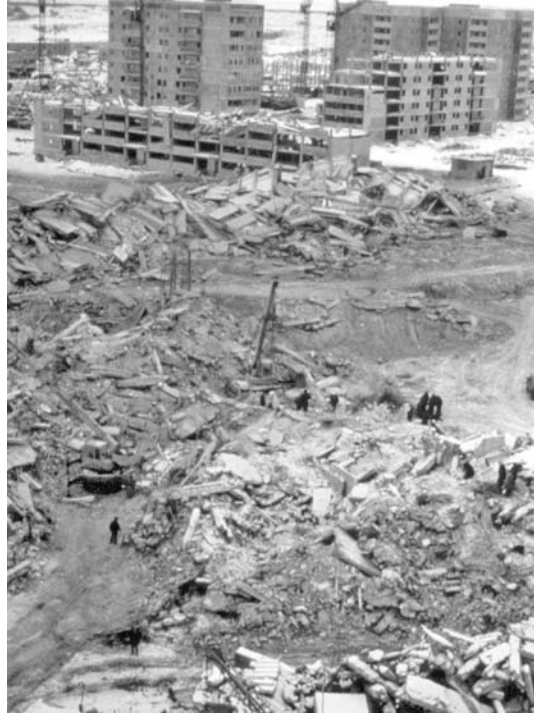
Fig. 1.18 Survival of precast panel buildings adjacent to razed precast frame buildings, Spitak, Armenia, 1988
