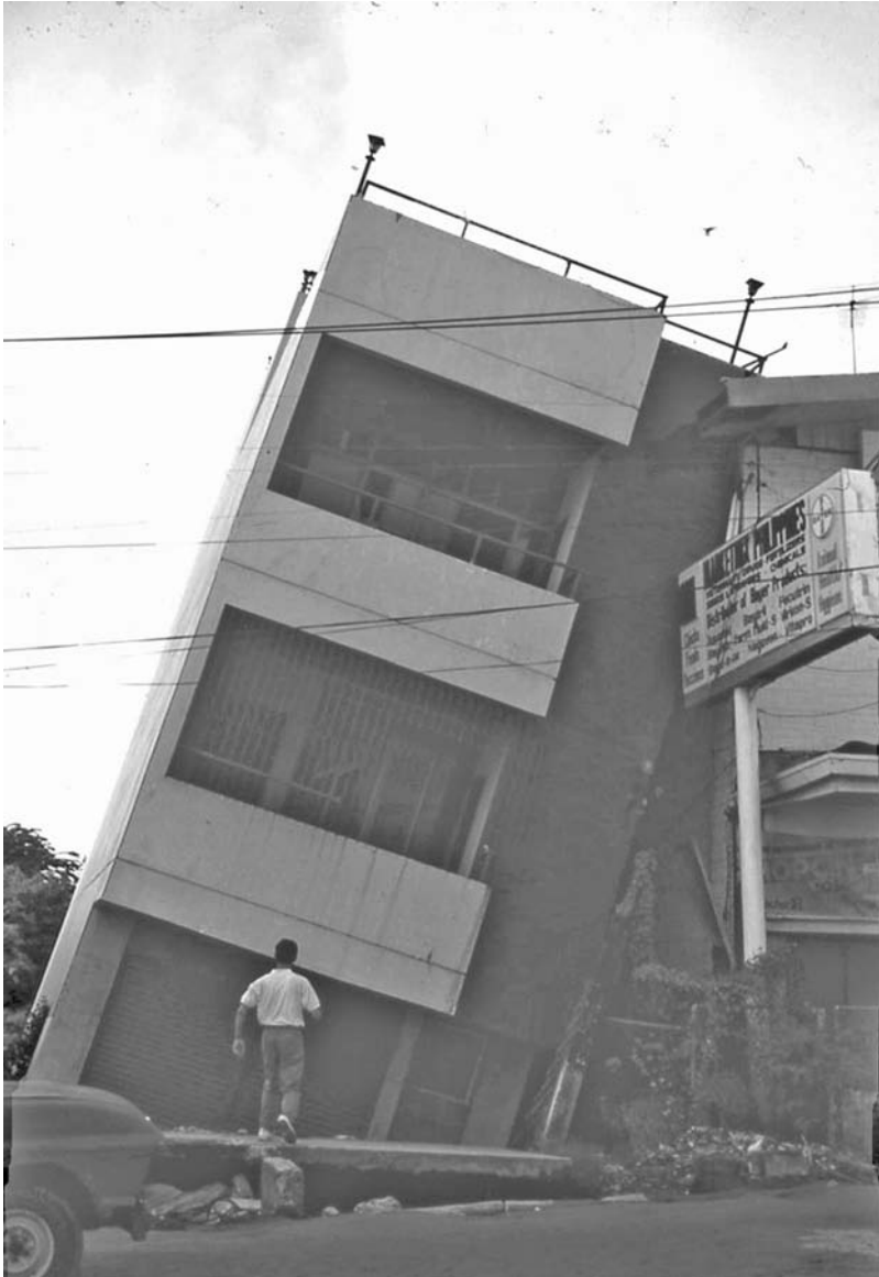
Fig. 1.23 Gross settlements due to liquefaction, Dagupan, Philippines, 1990
