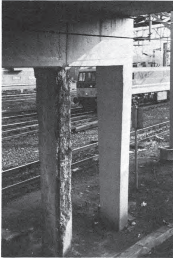
Fig. 9.9 Repaired column, Stafford Bridge.
