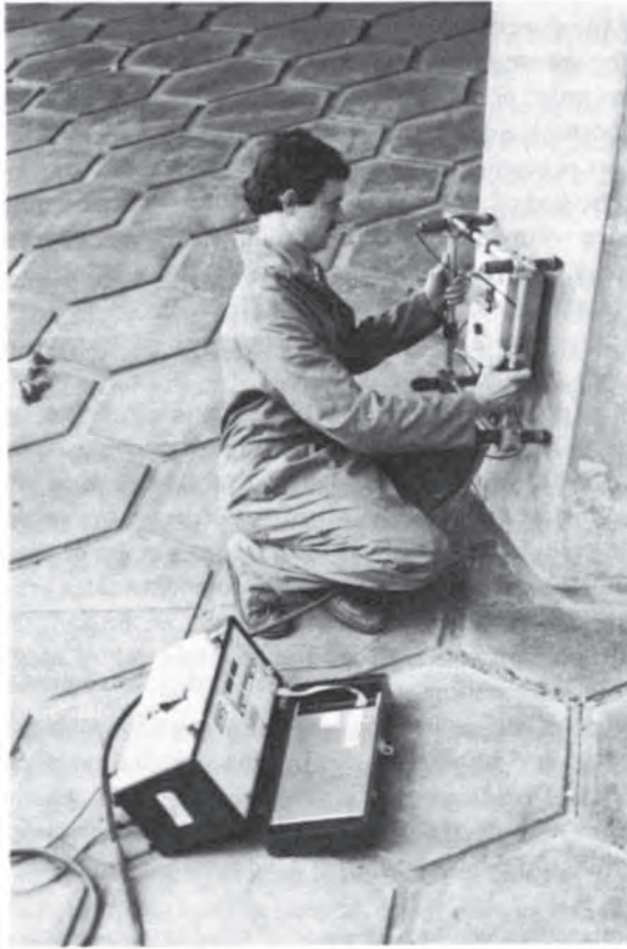
Fig. 3.7 Use of half-cell potential data logger on bridge column.
