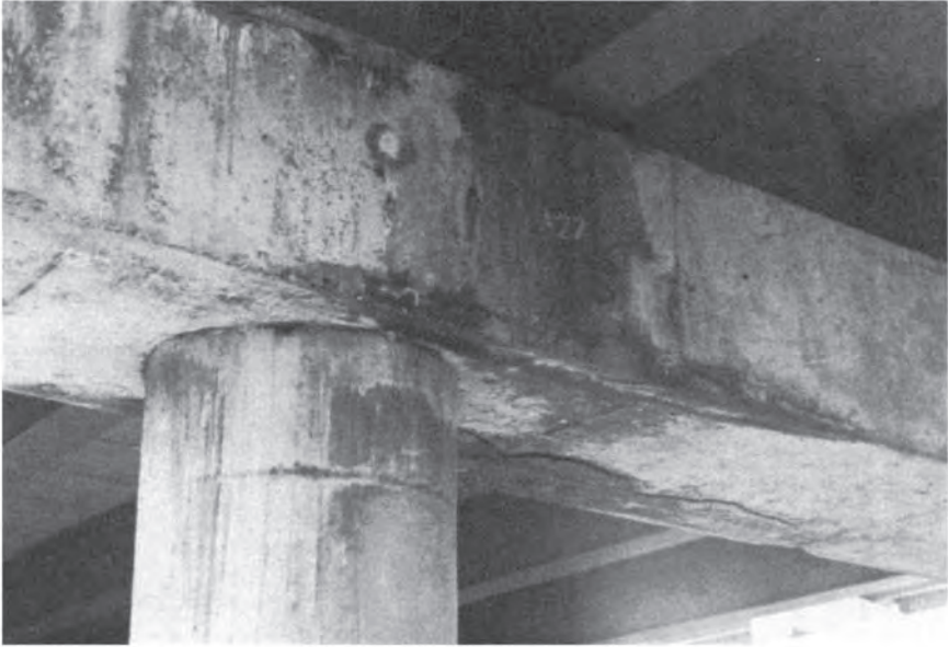
Fig. 8.3 Midlands Links Viaduct substructure.
