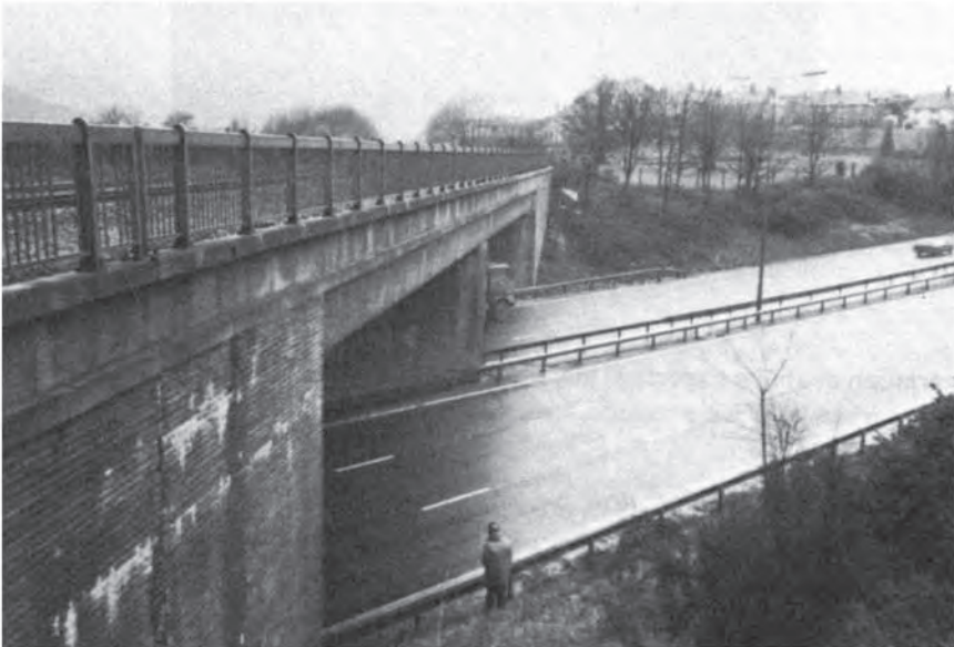
Fig. 9.11 Bassaleg Bridge, Newport, South Wales.
